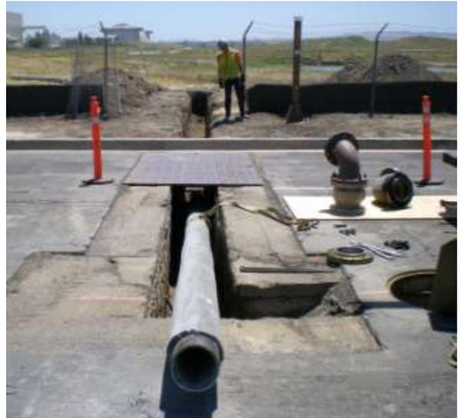
**Installation of pipe for new air release and vacuum valve located in Tustin**
