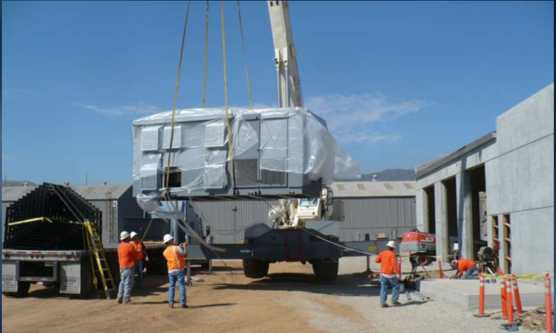
Setting loadbank for standby generators
