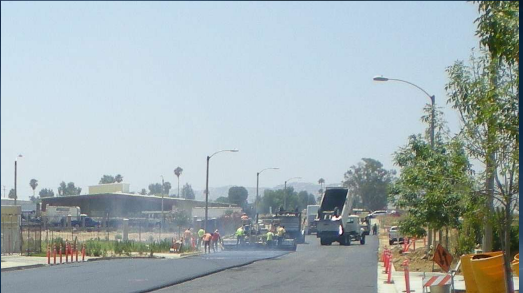
Street paving on Western Way
