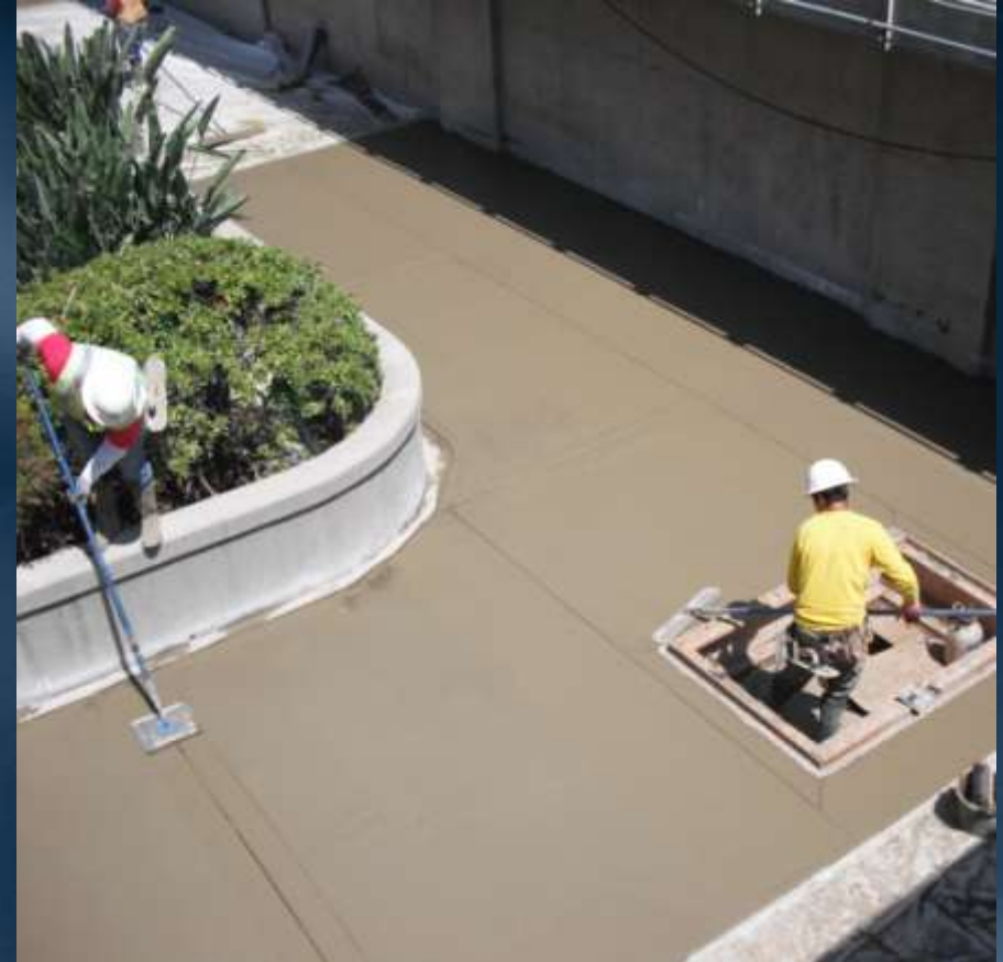
Deck concrete finishing
