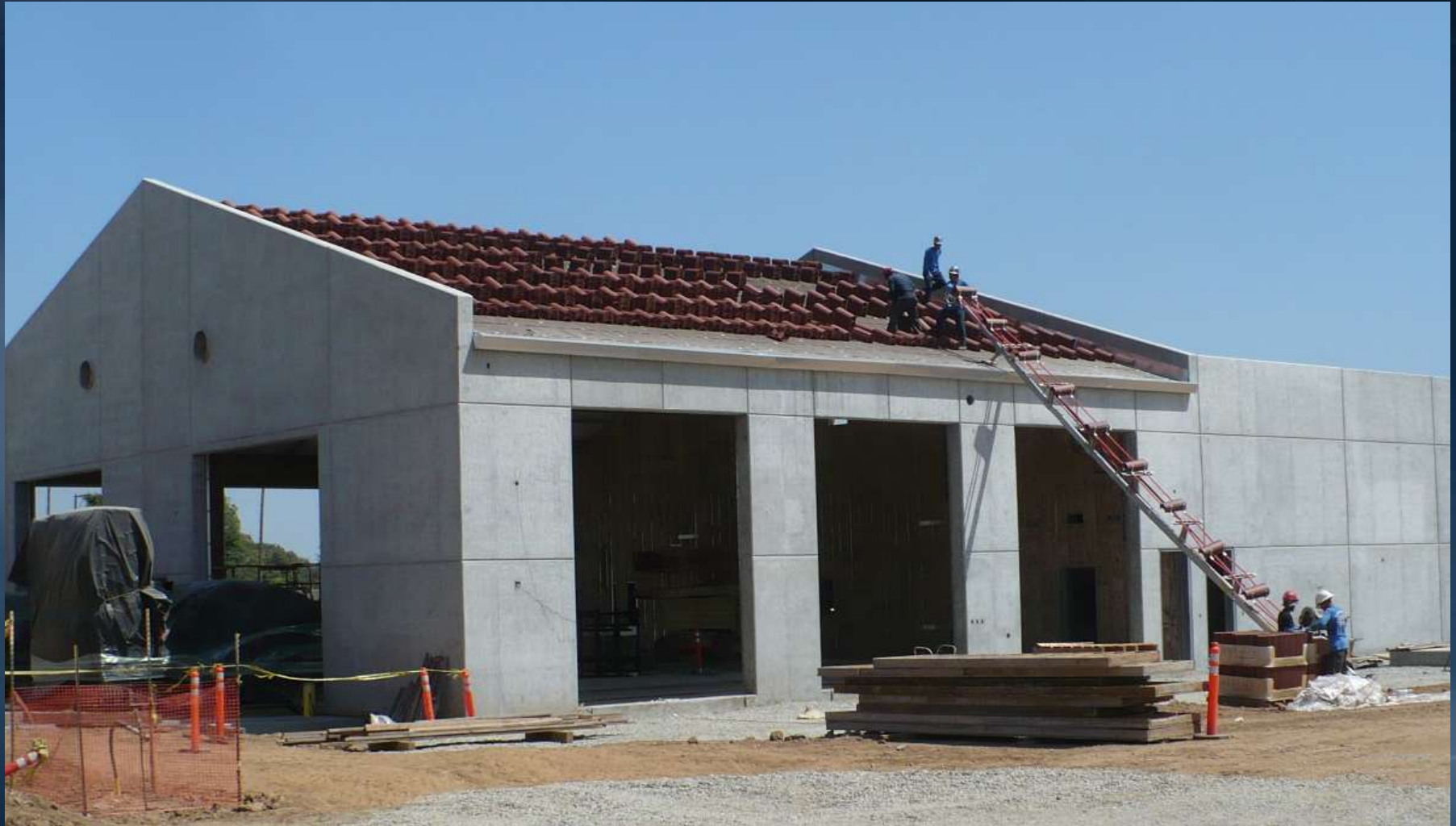
Main switchgear building roof tile installation
