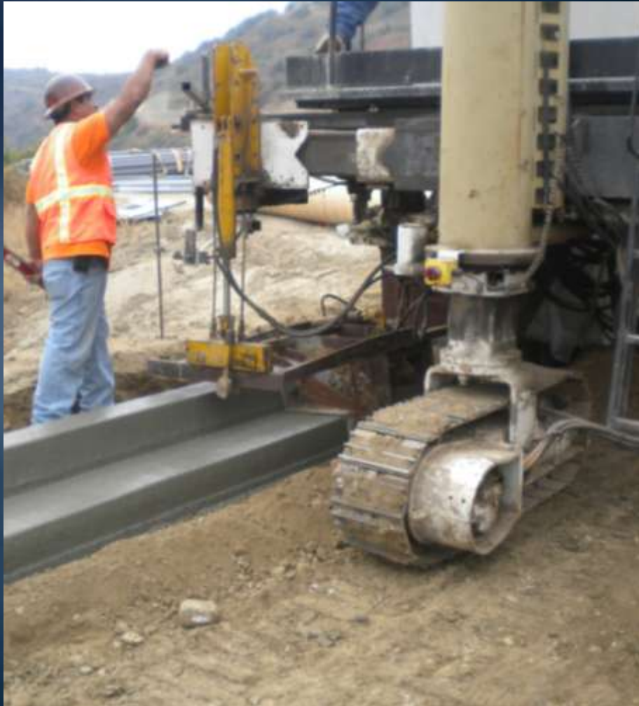
Curb and gutter installation
