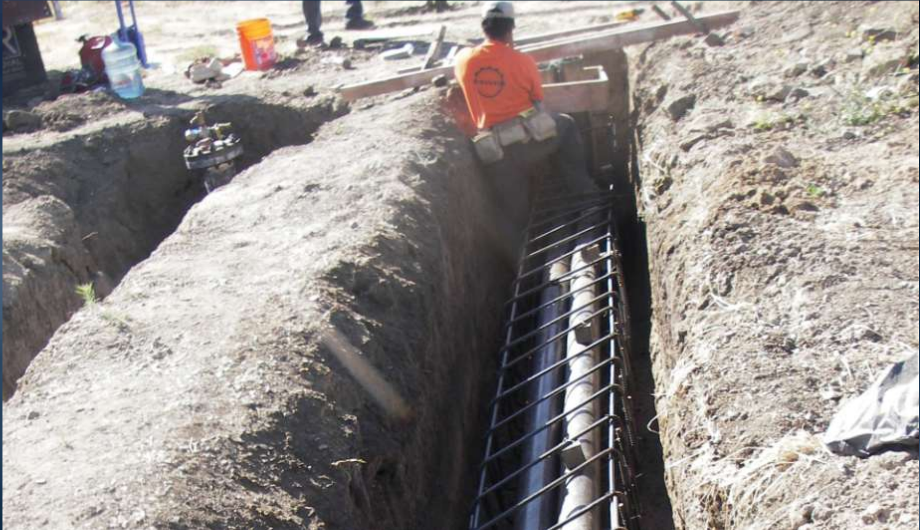
Reinforcing steel encasement of air vent and piping
