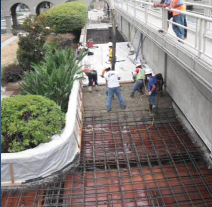
Deck concrete placement
