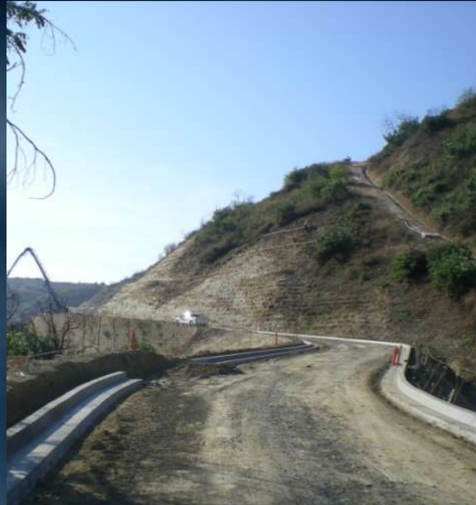
Curb and gutter installation
