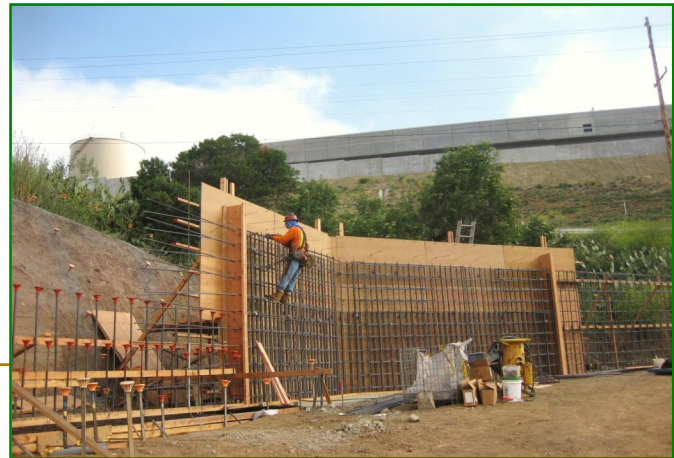
Diemer plant—Framework at the Fire and Potable Water Pump Station
