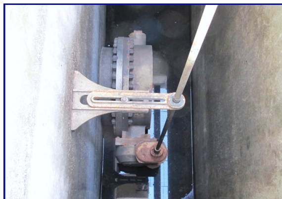
MILLS - Coating Teams completed blasting and coating of all 30-inch filter influent butterfly valves, mounting and support brackets for the Module No. 3 and 4 rehabilitation project.
