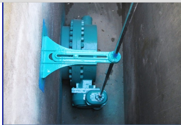
MILLS - Coating Teams completed blasting and coating of all 30-inch filter influent butterfly valves, mounting and support brackets for the Module No. 3 and 4 rehabilitation project.
