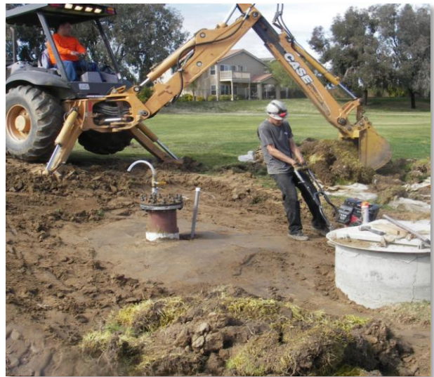
Backfill of a completed installation in Temecula
