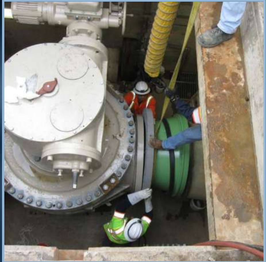
Installing reducer piece
