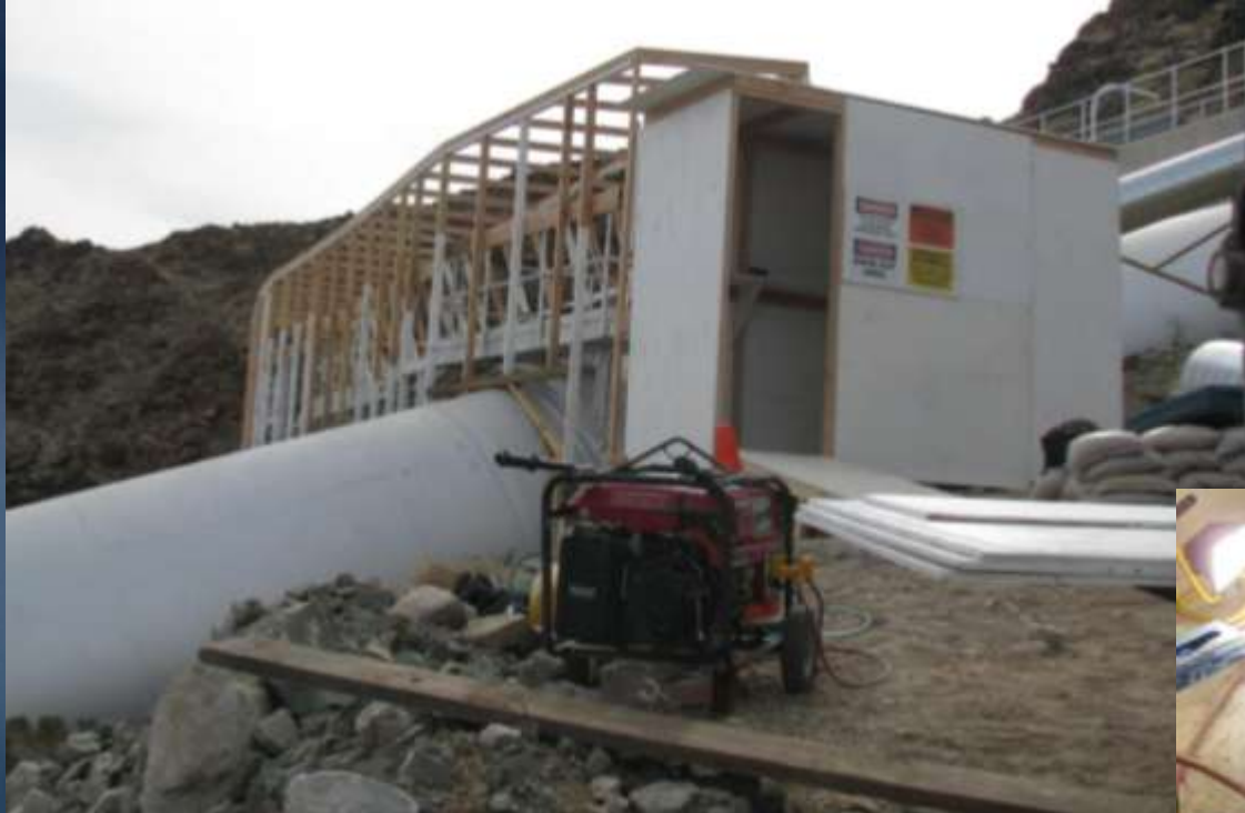
Waste material containment structure
