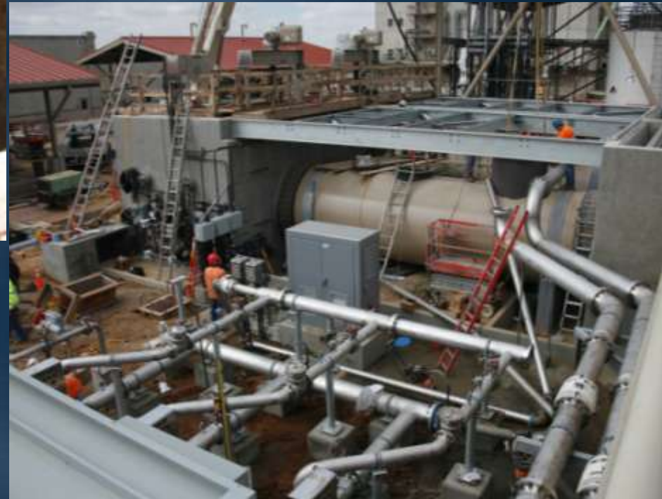
Rapid Mix start-up testing
