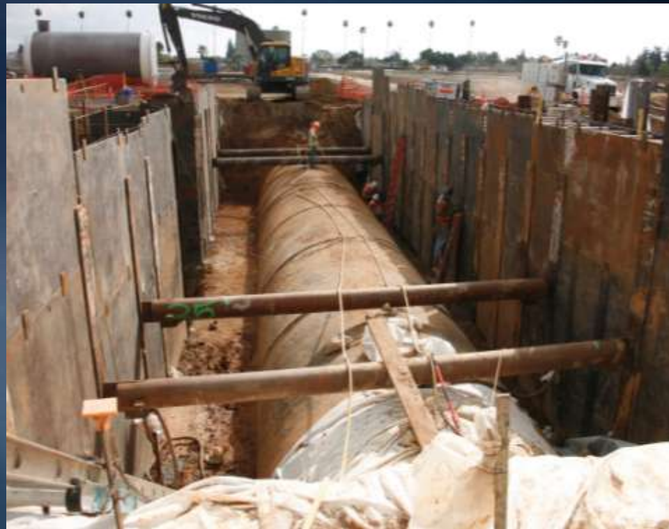
Excavation of upper feeder tie-in point
