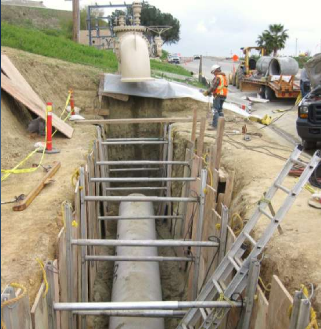
Installation of 36" potable water pipe
