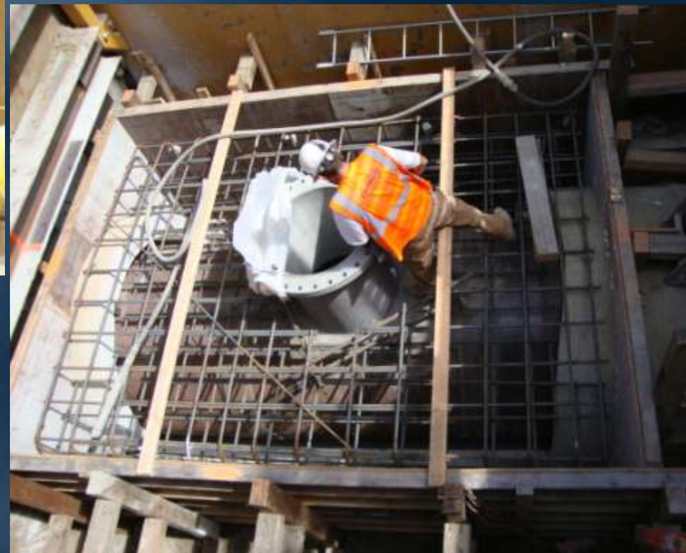
Rebar and formwork for encasement
