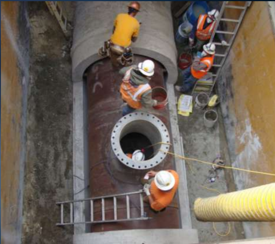
Installation of new pipe segment
