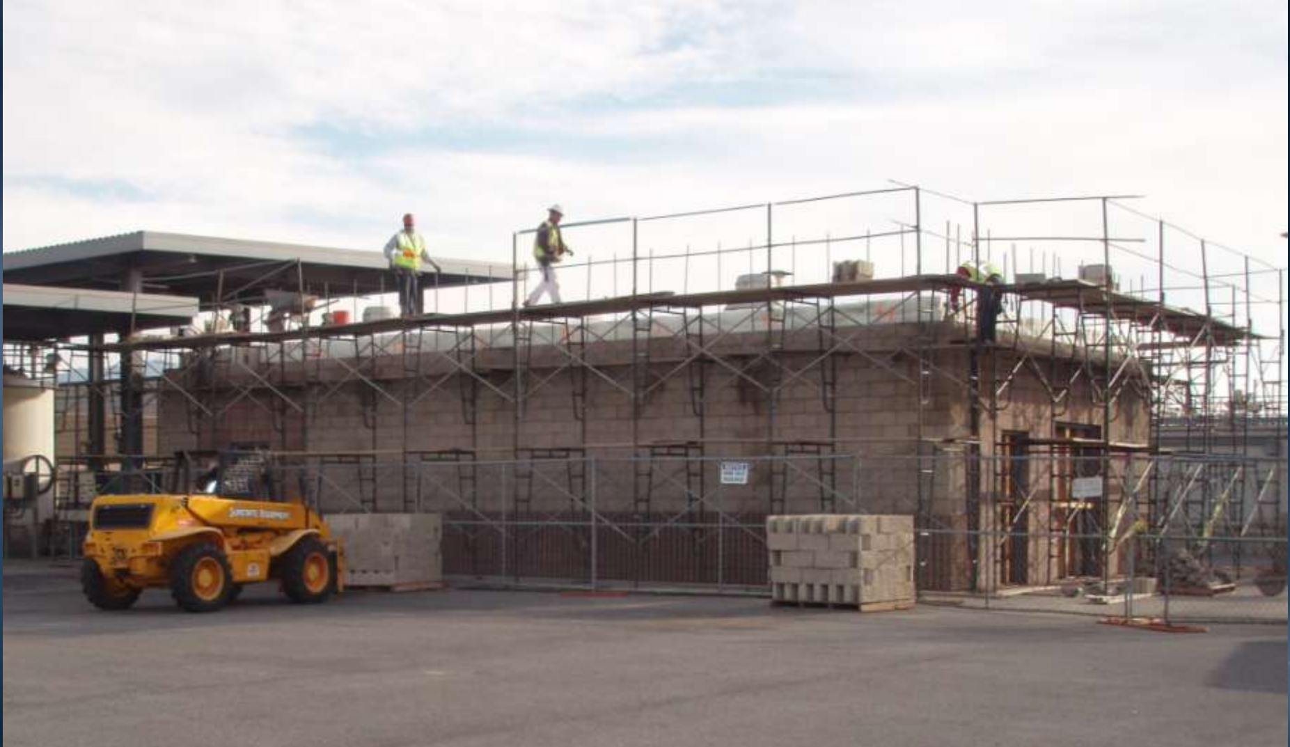
Installing masonry units
