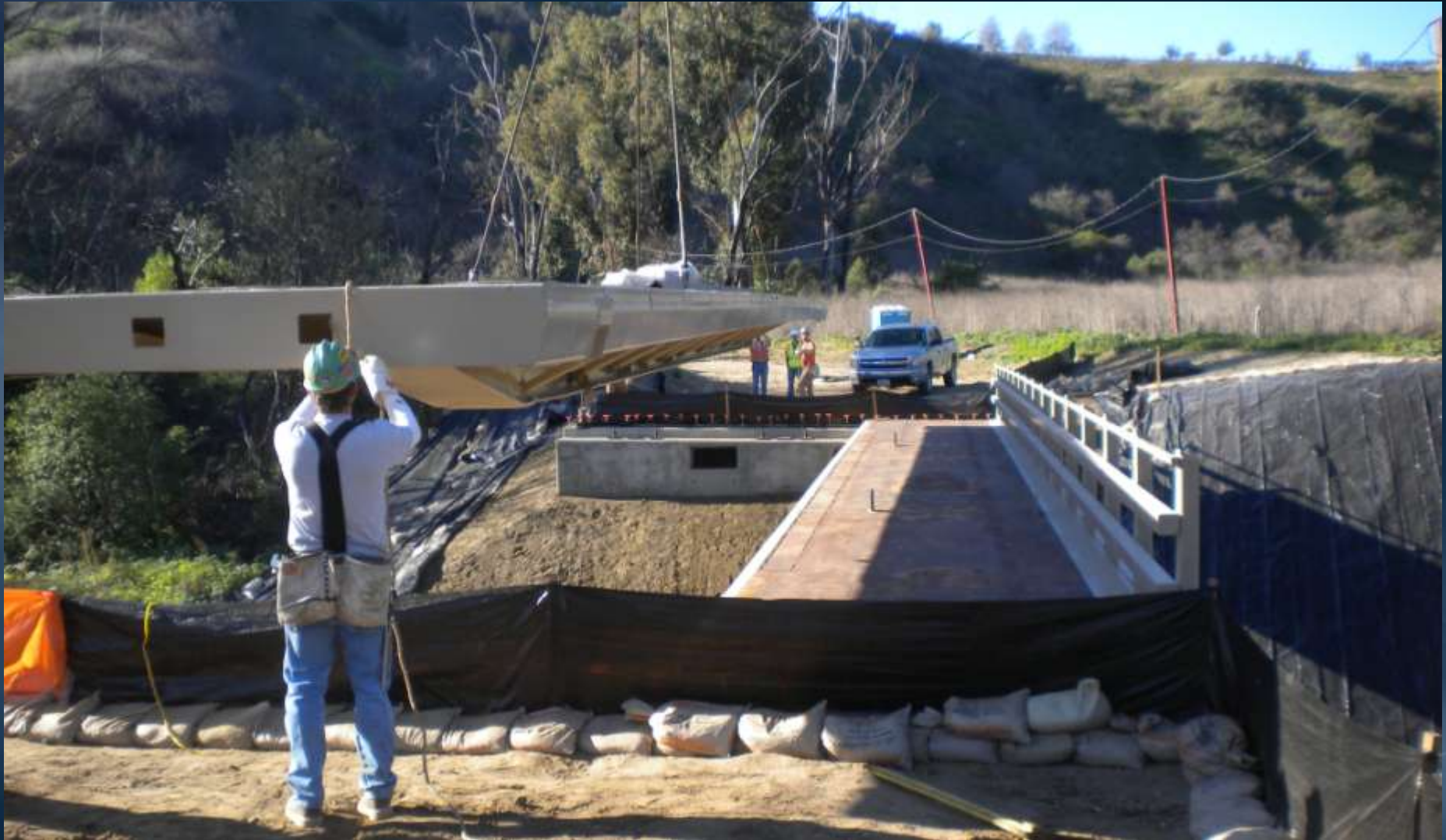
Setting deck of Carbon Canyon Creek Bridge
