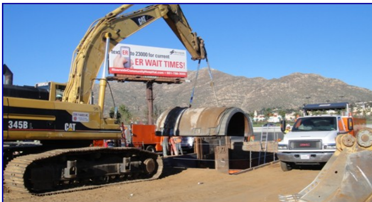
Contractor removal of distressed pipe section on Box Springs Feeder
