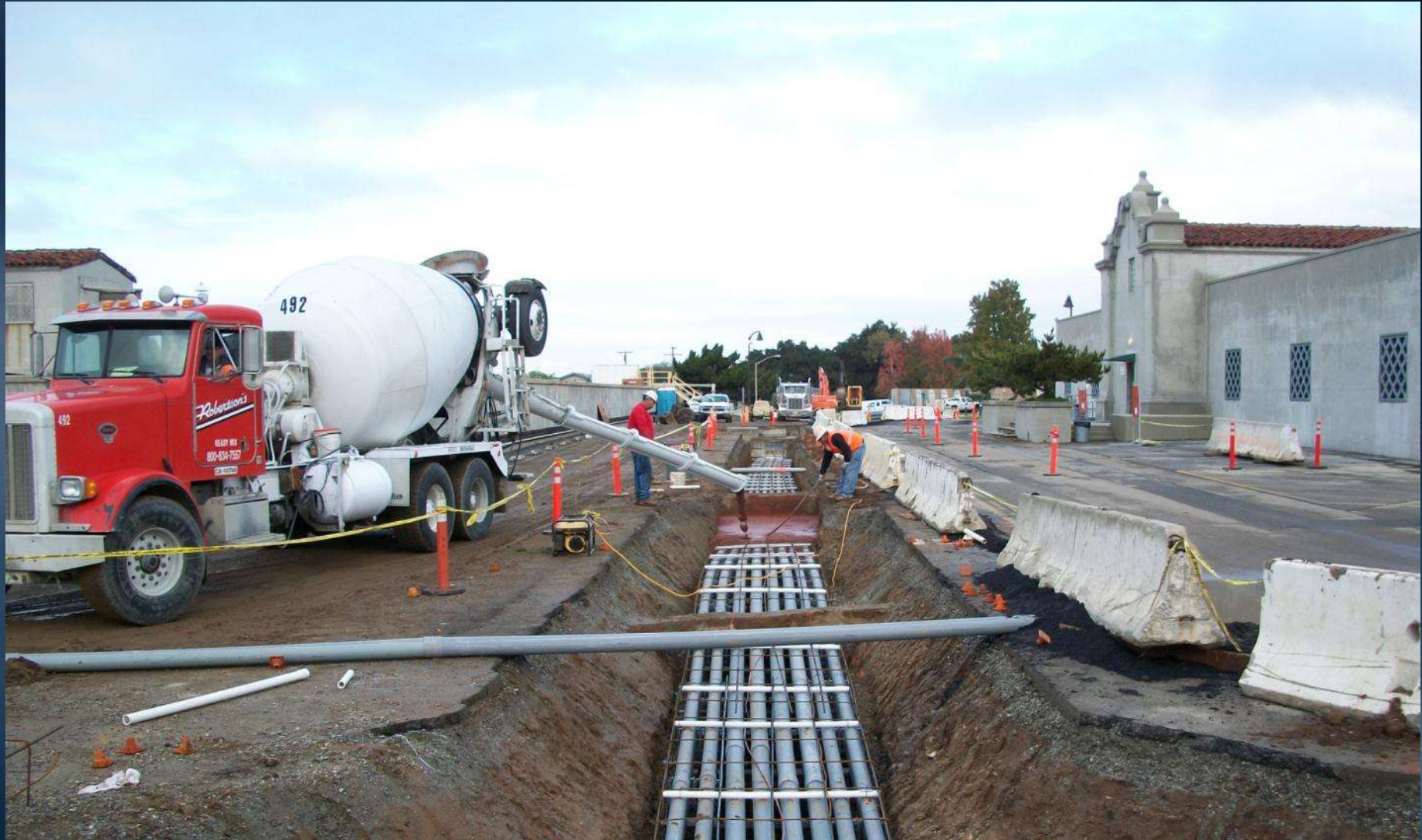
Concrete placement
