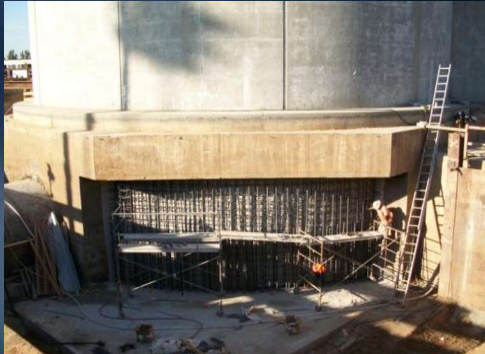
Rebar placement
