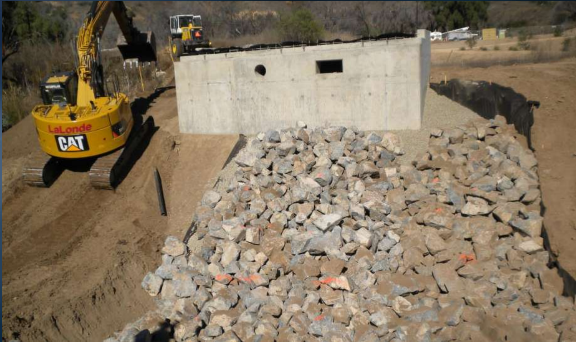
Bridge abutment protection
