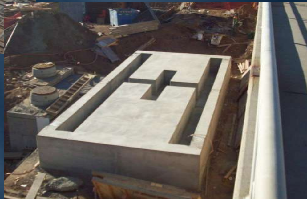
Finished Motor Control Center slab
