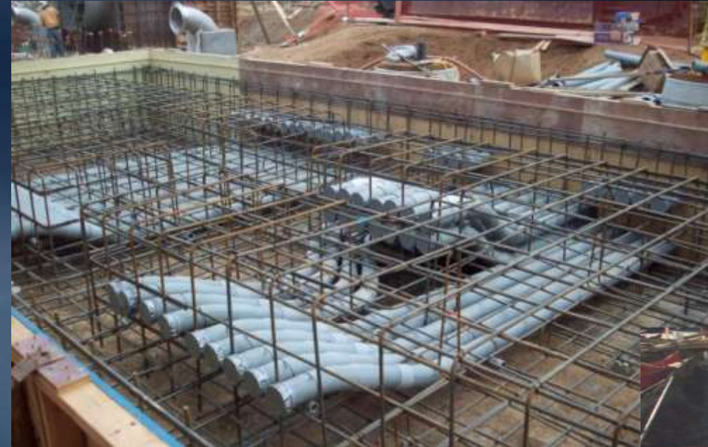
Motor Control Center conduit and formwork
