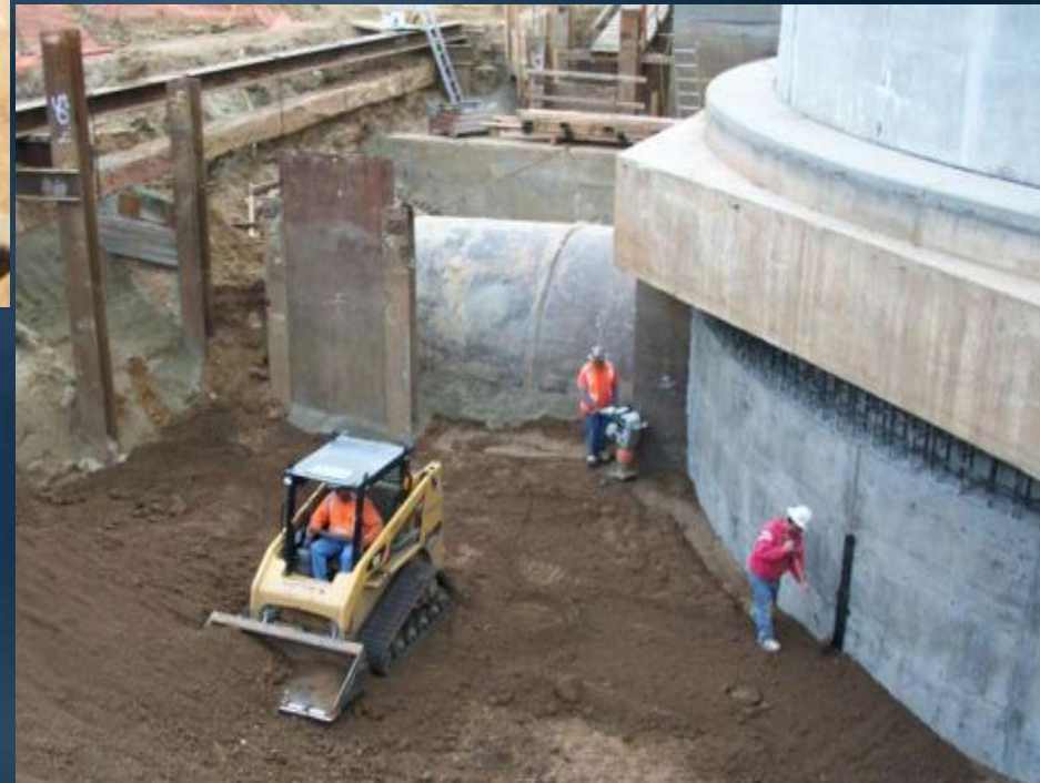
Backfill after concrete placement
