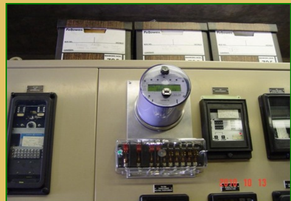
New CAL-ISO Meter at Valley View HEP
