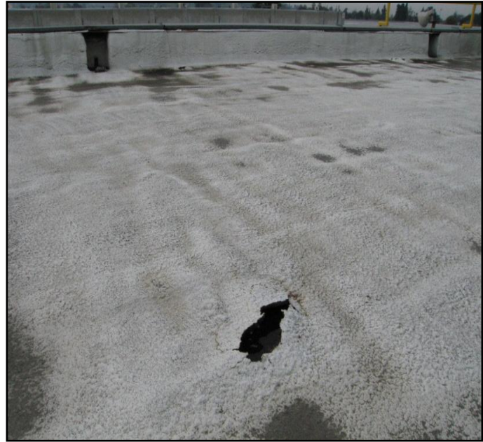
La Verne Machine Shop Upgrades Machine Shop roof to be replaced
