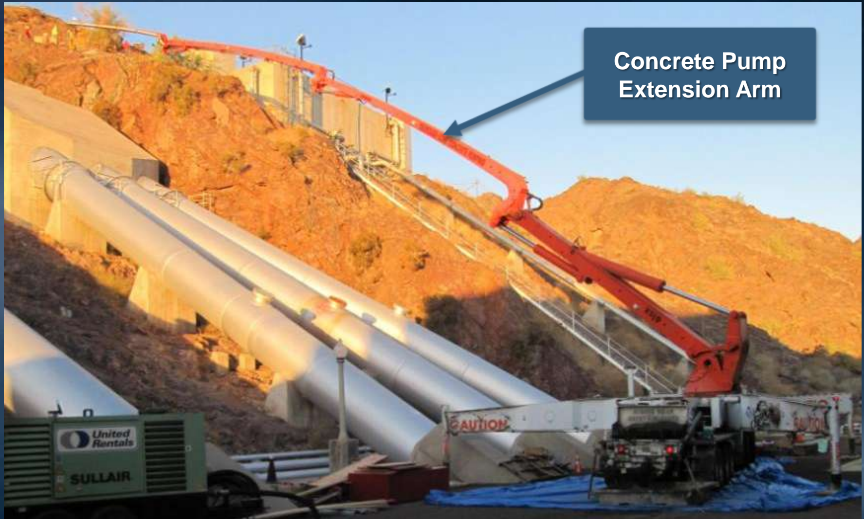
Pedestrian stairway construction
