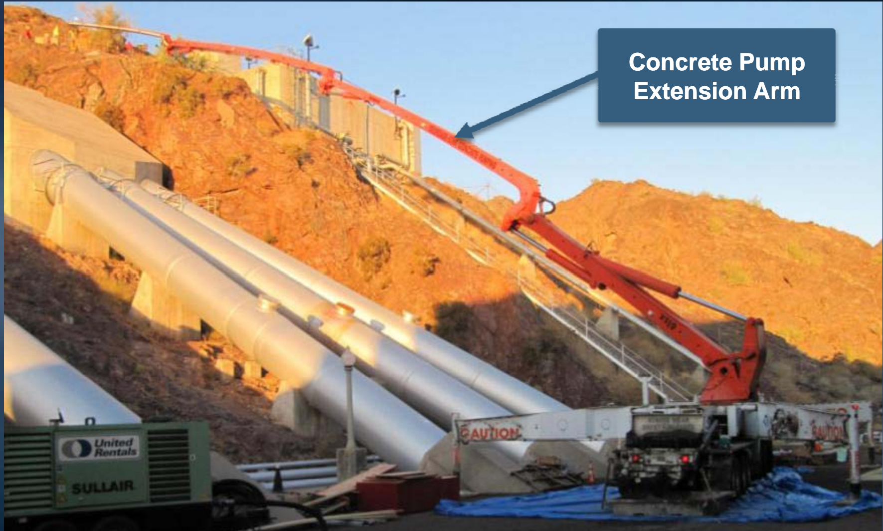
Pedestrian stairway construction
