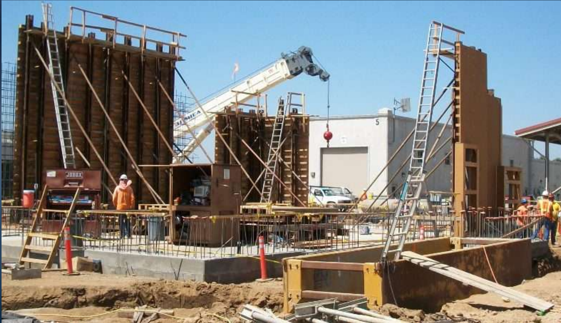
Main plant switchgear building wall forms
