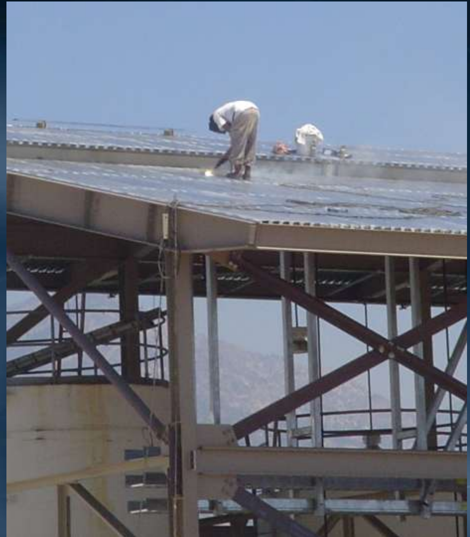
Welding metal roof deck
