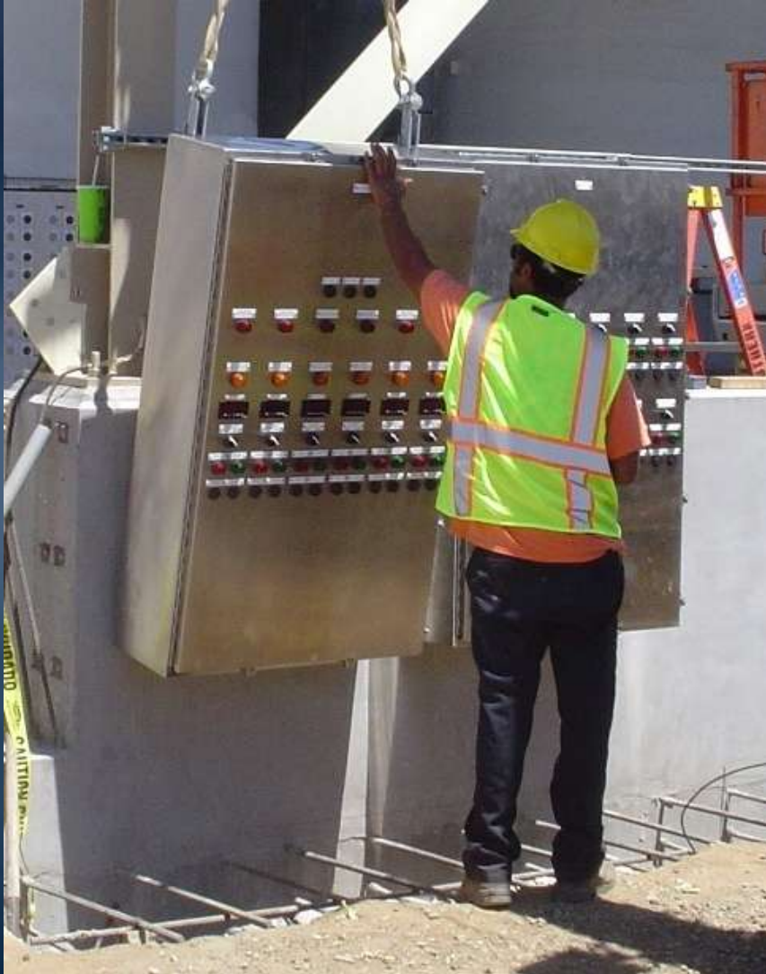
Control panel installation
