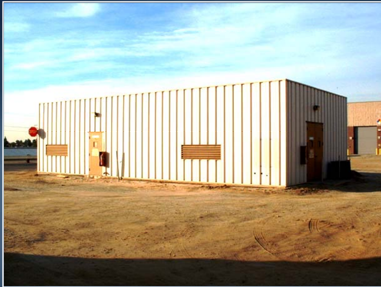
Electrical Bldg No. 1
