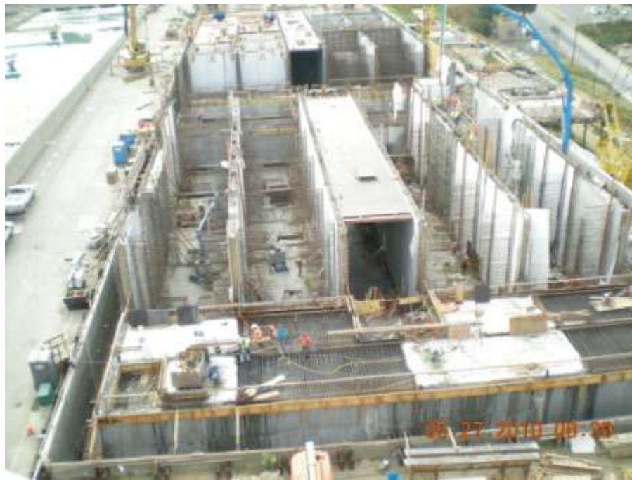
Figure 6: Construction of Diemer at ozone contactors
