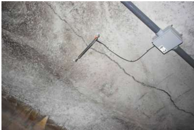
Figure 4: Crack meter at the crown of Iron Mountain Tunnel
