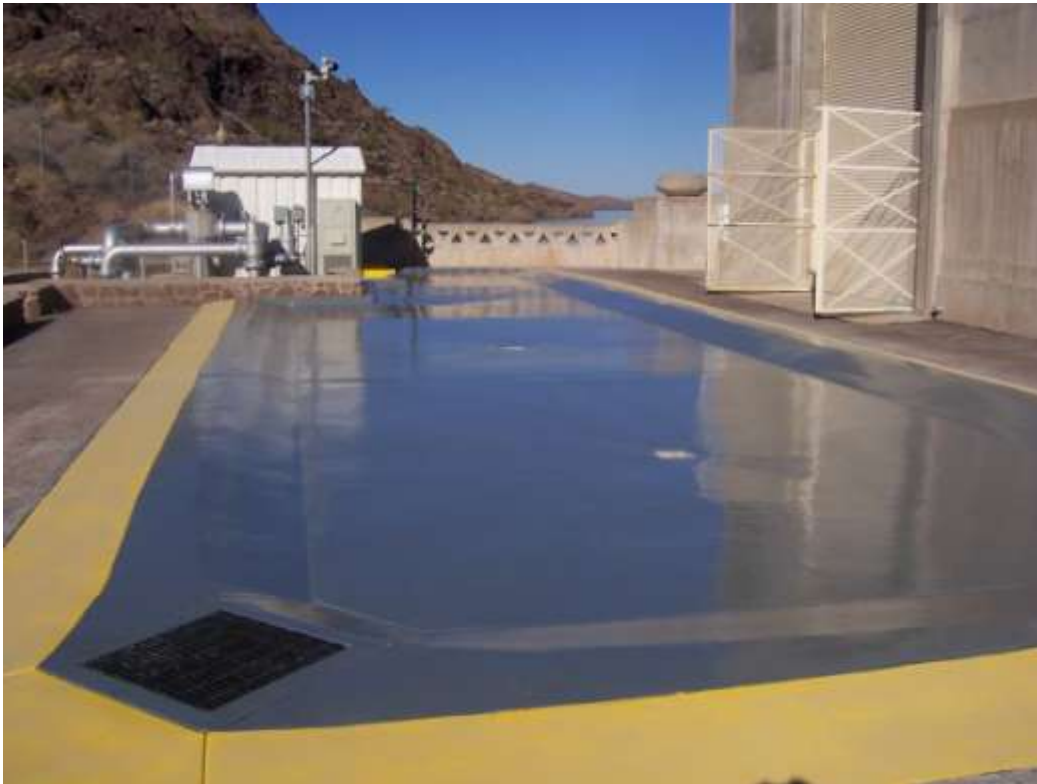
Figure 8: Completed unloading containment pad at Intake Pumping Plant
