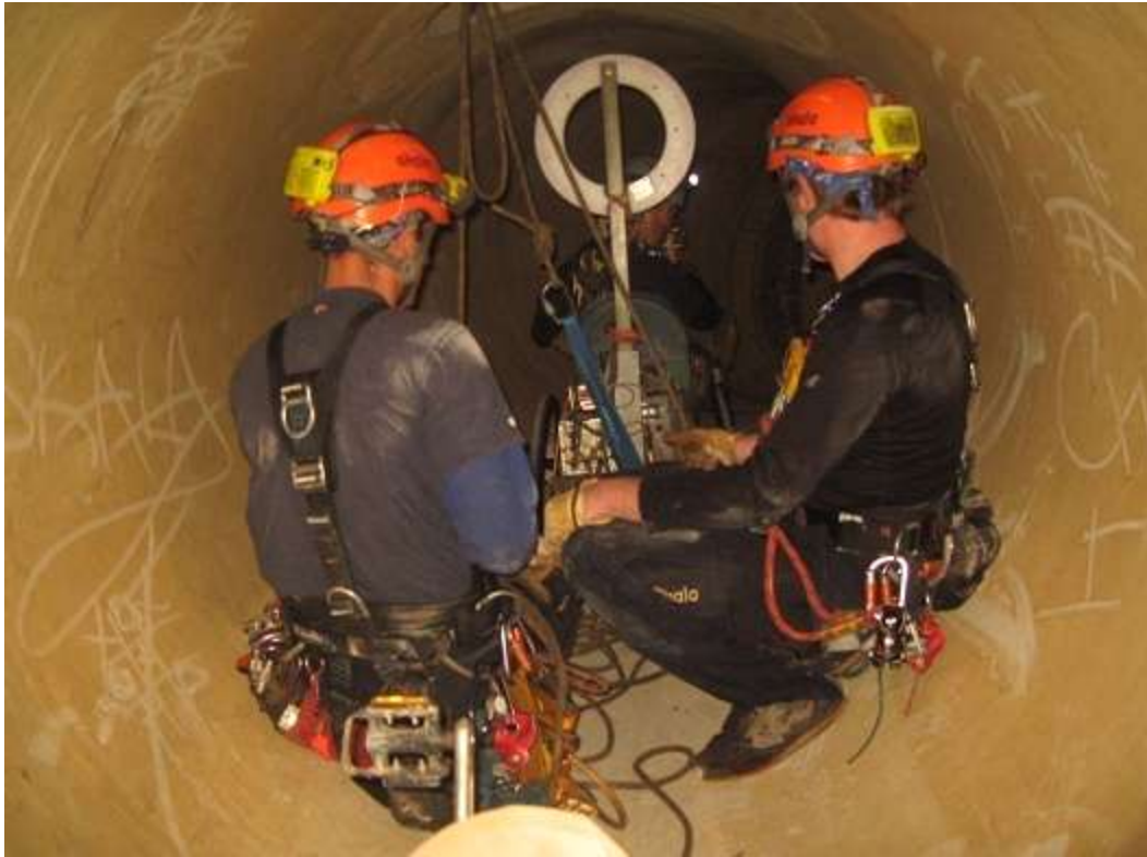
Figure 2: Remote Field Eddy Current (electromagnetic) inspection of the Calabasas Feeder
