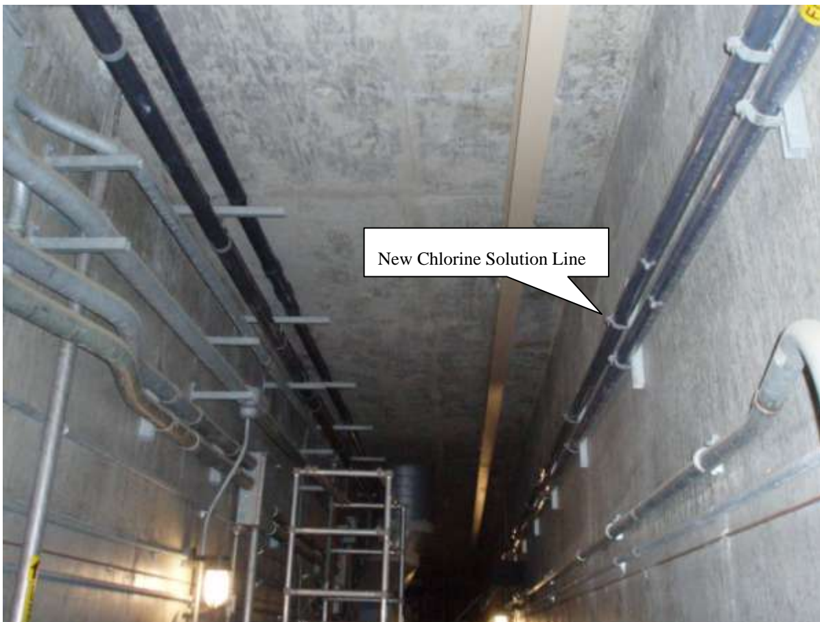
Figure 7: Construction of Mills Filter Outlet Chlorine Project
