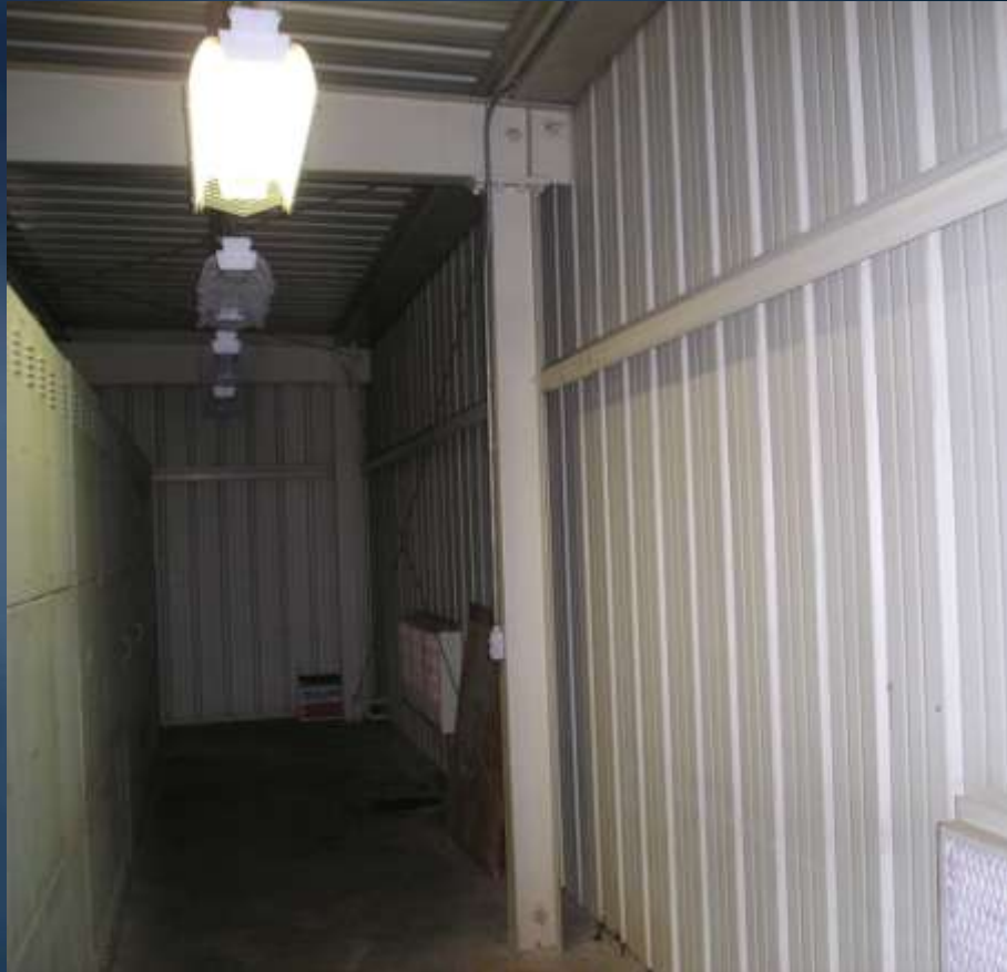
Typical UPC Building
