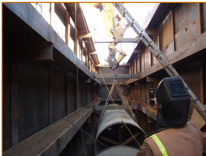
Pipe installation in deep, shored section of Western Way
