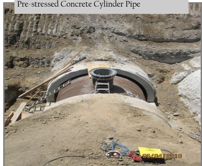
Lake Skinner Outlet Conduit Shutdown repair of Pre-stressed Concrete Cylinder Pipe
