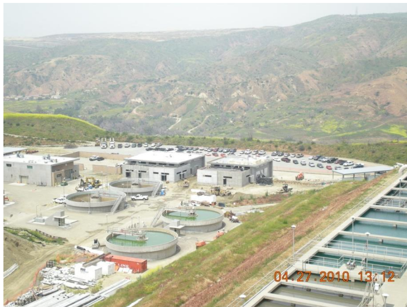
Figure 8: Diemer plant –Northwest view of solids clarifiers, Generator Building and Switchgear Building
