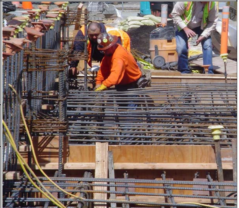
Placement of reinforcing steel
