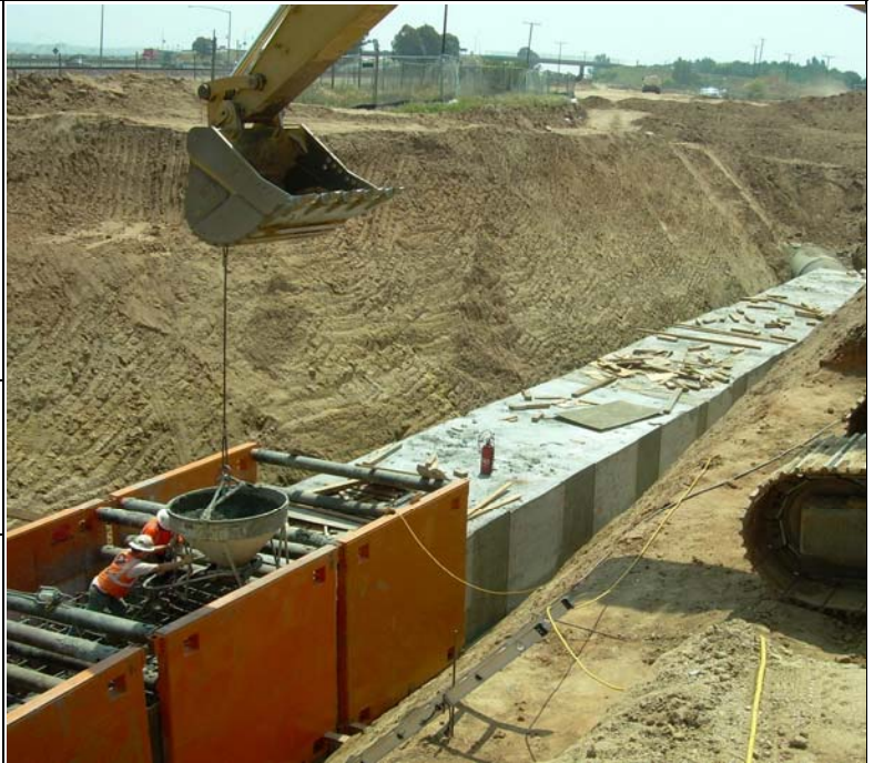
Concrete encasement of 97-inch pipe
