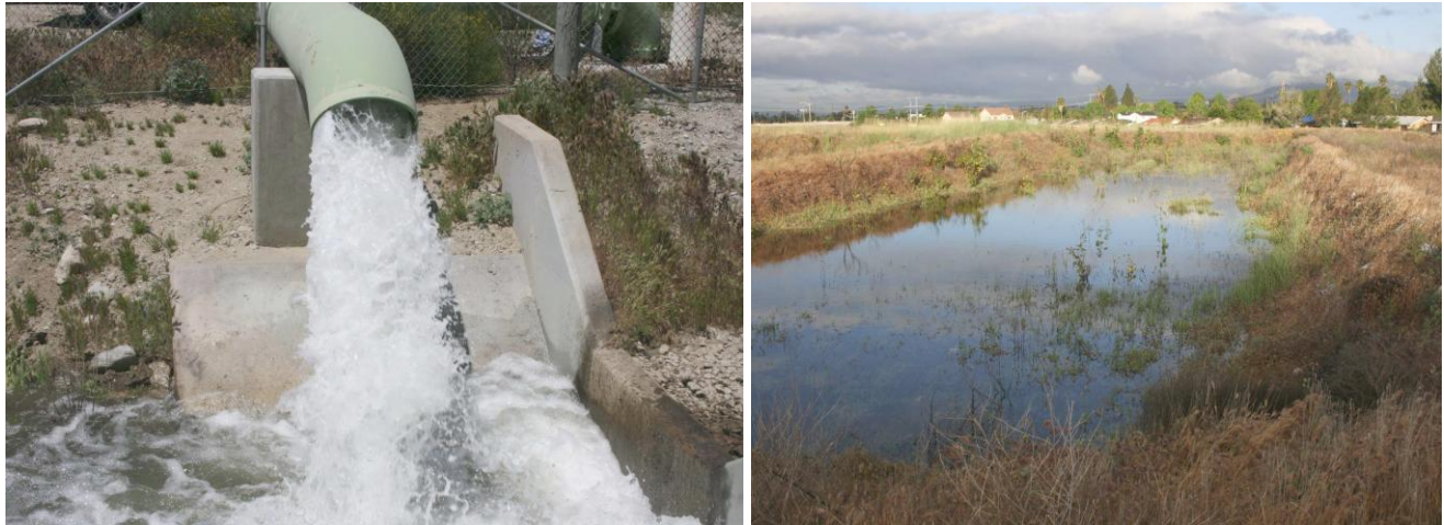
Figure 2: Left: Water delivery through service connection. Right: Spreading grounds
