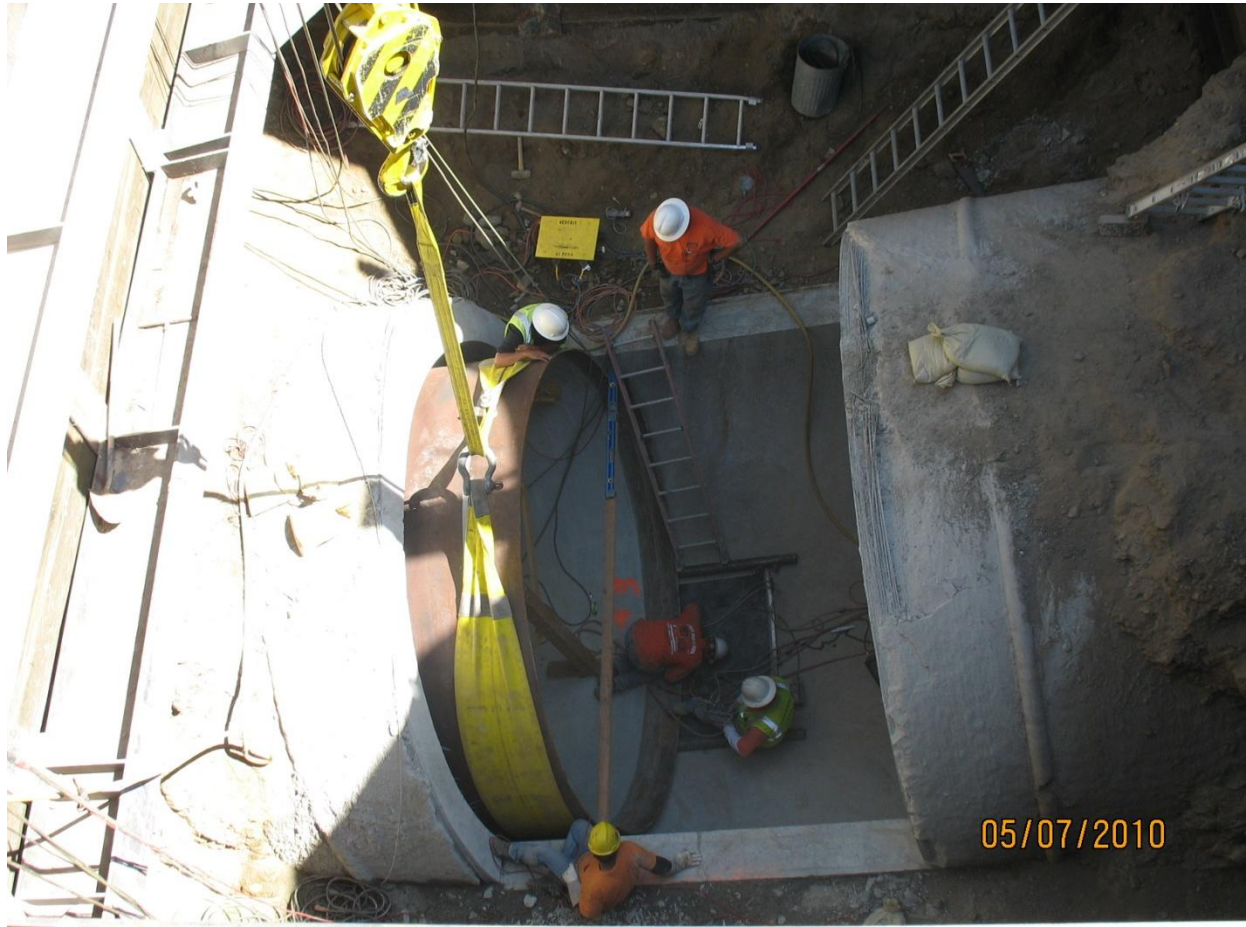
Figure 1: Replacement of distressed PCCP sections
