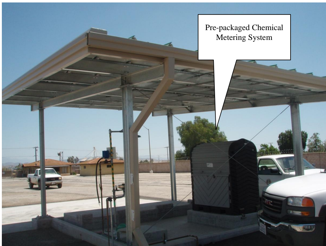
Figure 9: Construction progress of CUF Dechlorination System
