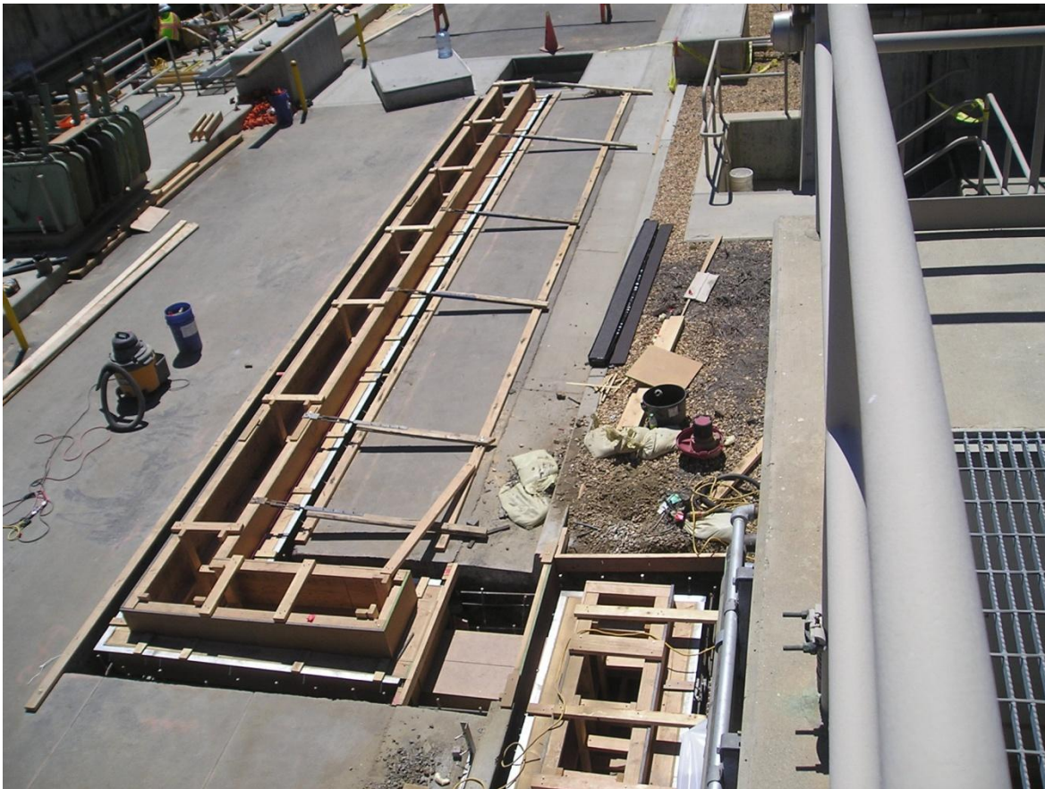
Figure 7: Concrete chemical trench construction under the Skinner Chemical System Improvements project
