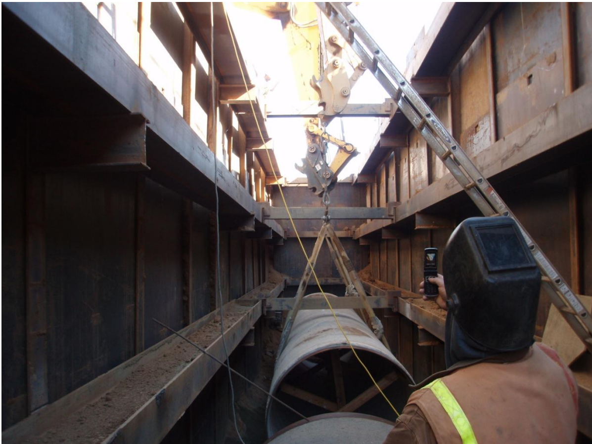
Figure 3: Pipe installation in deep, shored section of Western Way
