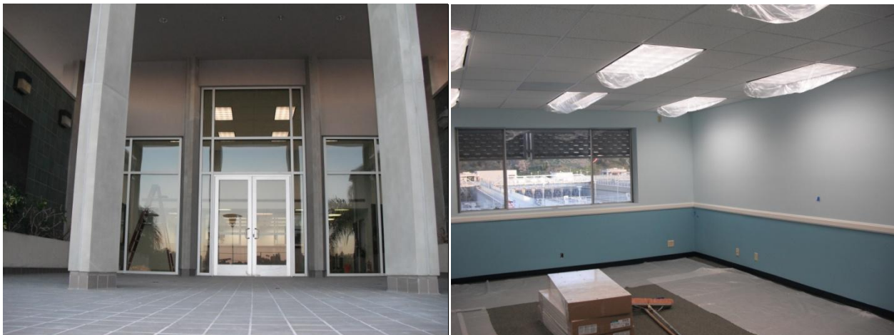
Figure 6: Completed seismic upgrades at the Jensen Administration Building
