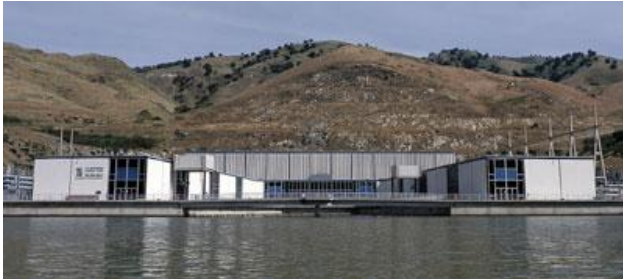
Edmonston Pumping Plant (DWR Photo).
