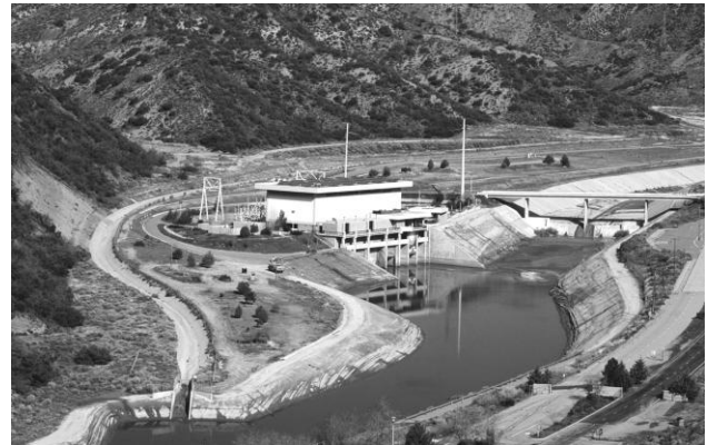
Warne Power Plant, located just upstream of Pyramid Lake (DWR Photo).
