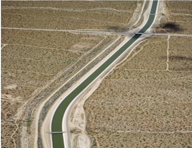
California Aqueduct in Southern California (DWR Photo).
