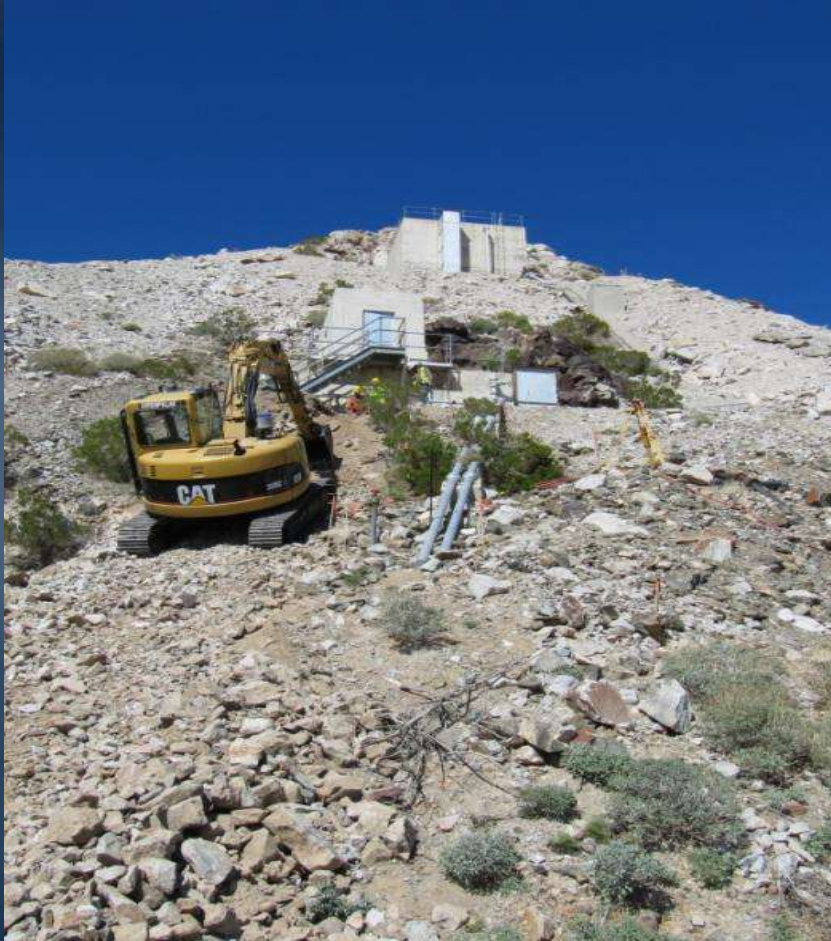
Hinds Pumping Plant excavating for stair footings
