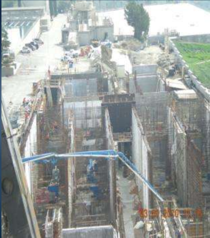
Ozone Building wall construction Looking South
