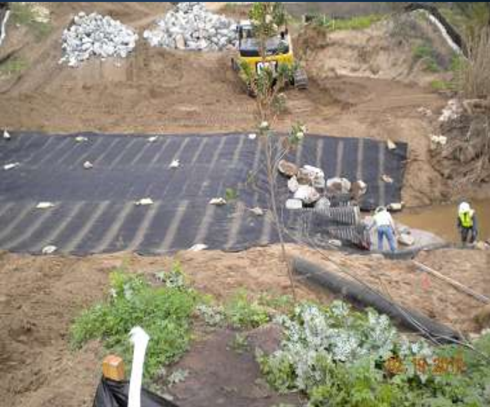
Temporary Crossing at Carbon Canyon Creek
