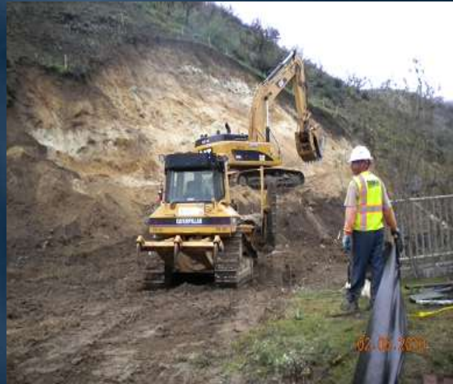
Pioneering/excavating road near the Basin 8 Dissipater Structure
