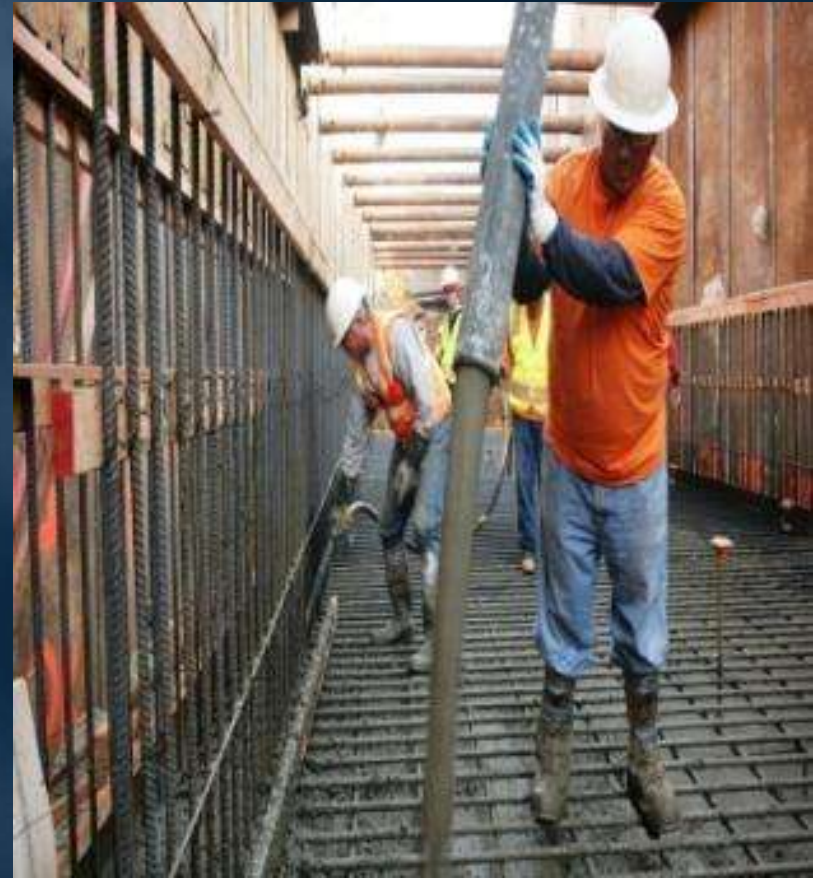
Placing concrete for Inlet Conduit slab
