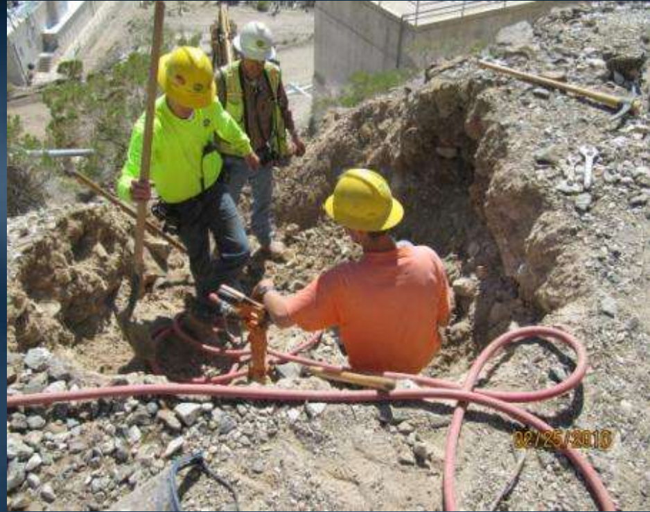
Surveyors checking location for stair footings on slope
