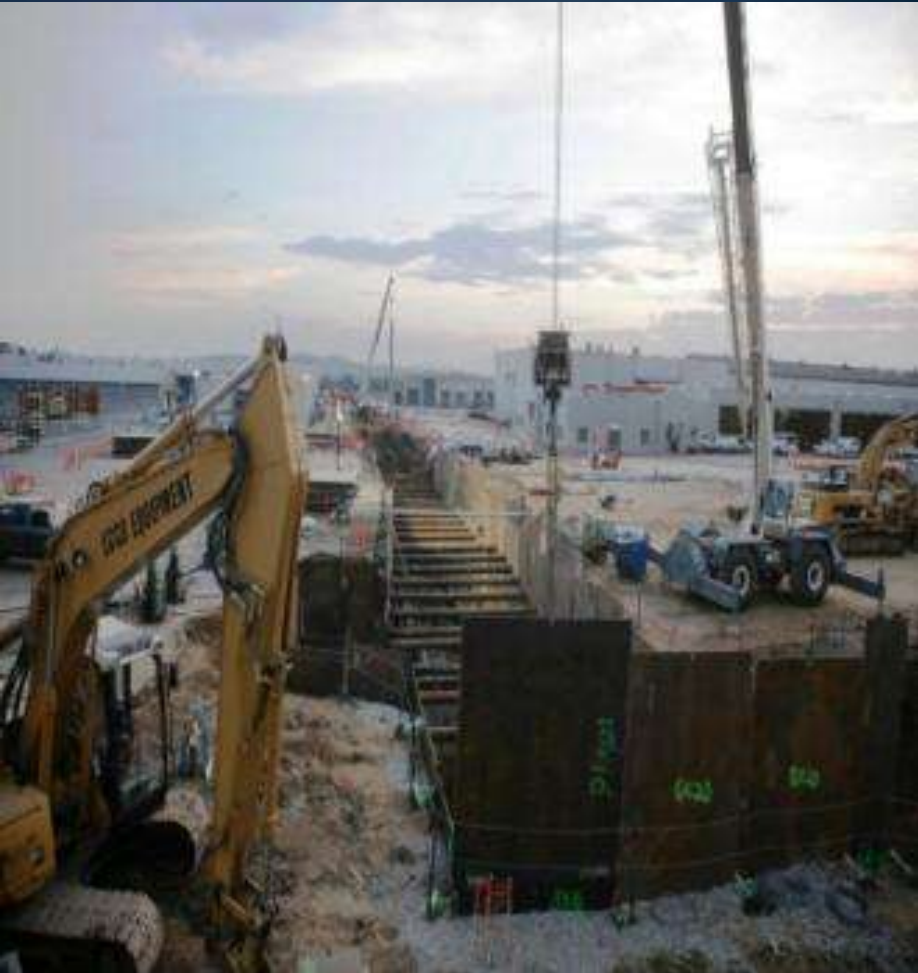
Looking South at Inlet Conduit trench excavation
