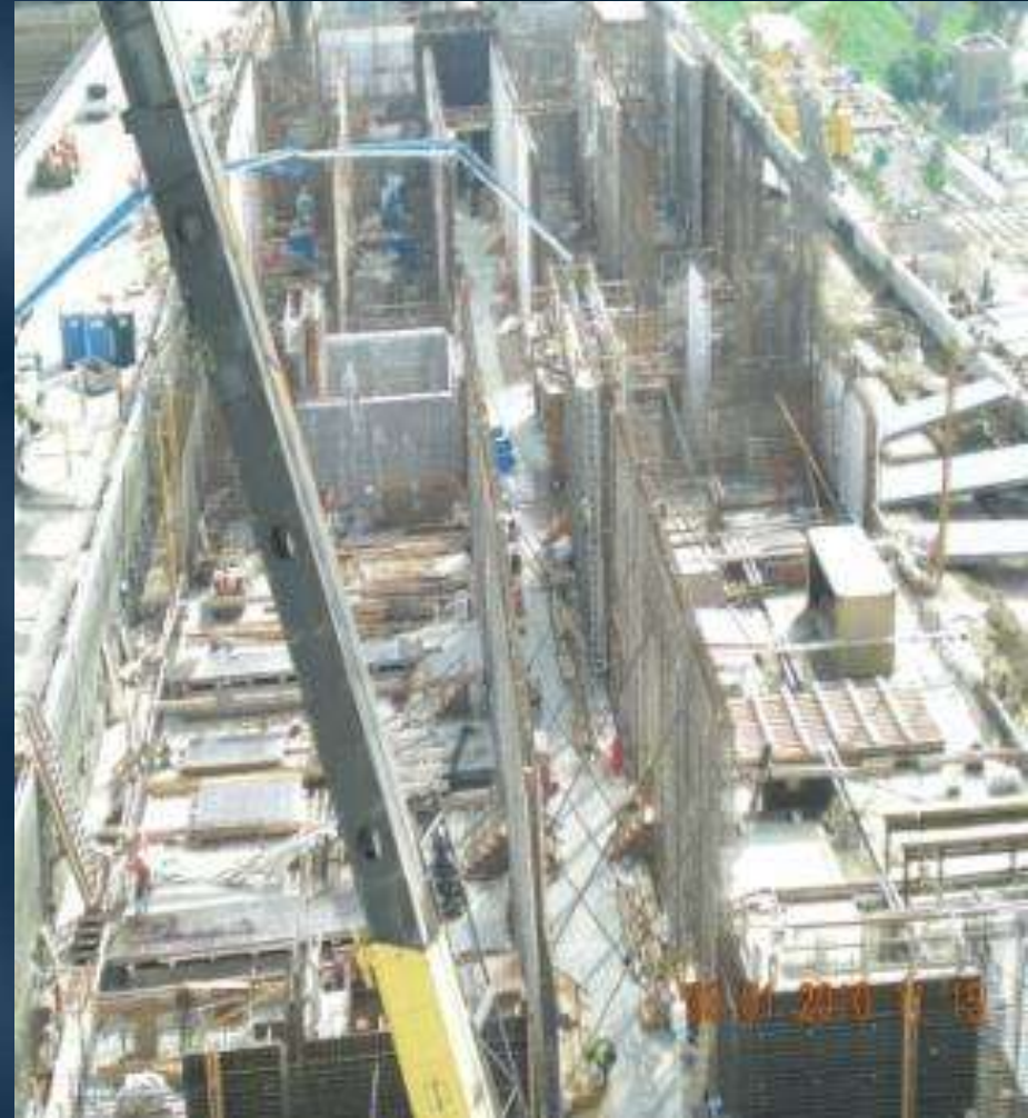
Ozone Contactors wall construction Looking East
