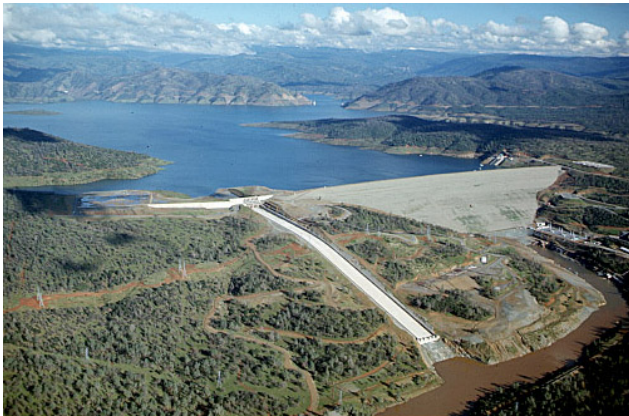
Figure 8. Oroville Dam (DWR Photo.)
