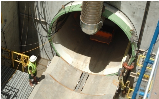
Figure 6. Arrowhead East Tunnel Construction for the Inland Feeder (MWD Photo.)
