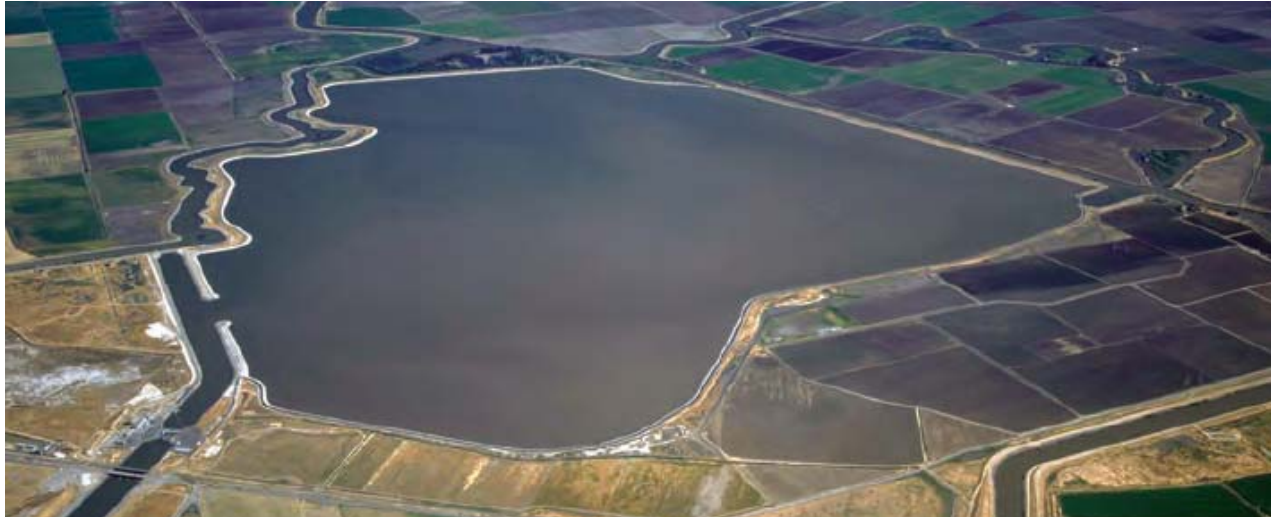
Figure 14. Clifton Court Forebay (DWR Photo).
