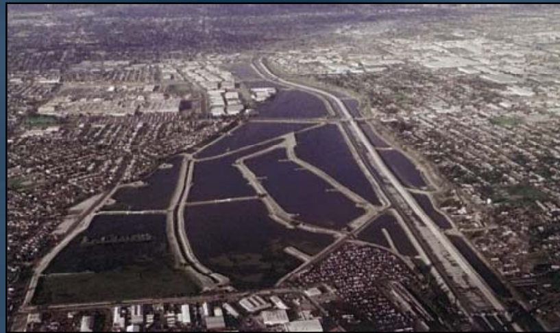
Groundwater Recharge at Rio Hondo Spreading Grounds
