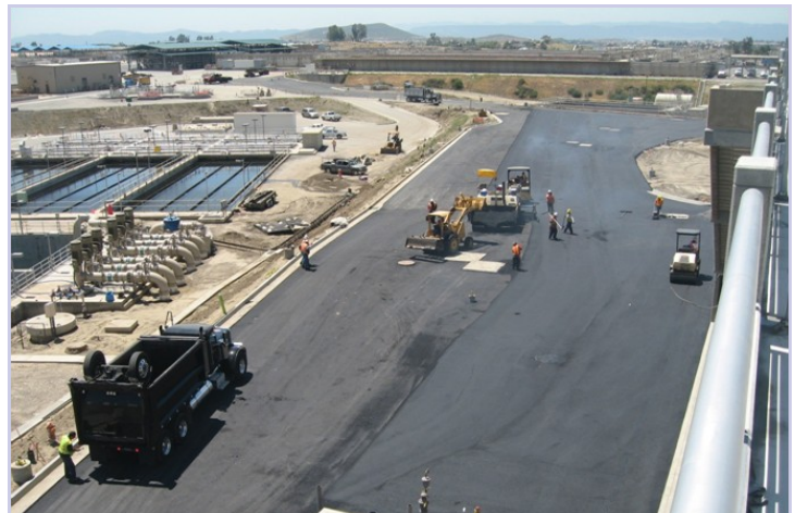
Paving around Skinner's reclaimed washwater return pumping station.
