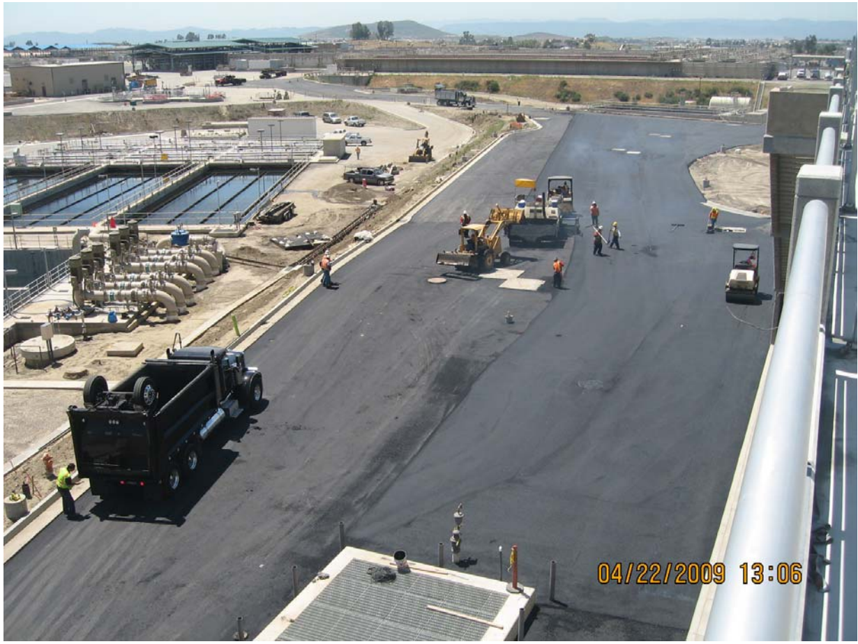
Figure 4: Paving around reclaimed washwater return pumping station
