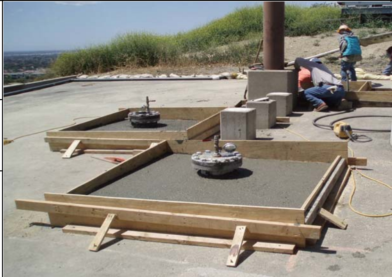
Placement of concrete enclosure pads located in Yorba Linda
