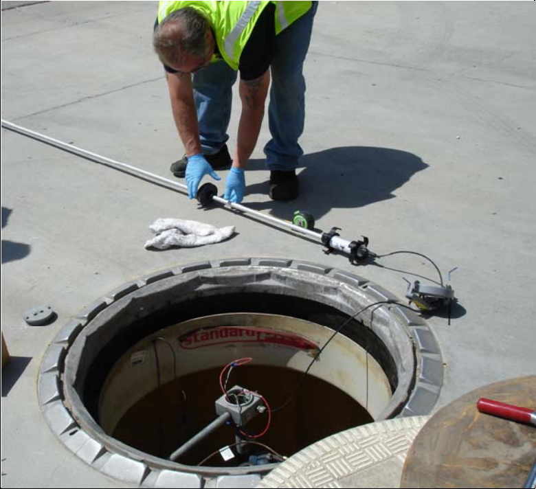
Testing and fire inspection at Jensen Plant
