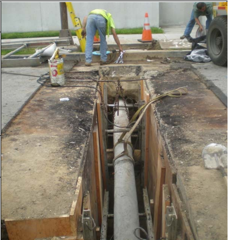
Installation of pipe extension located in Los Angeles
