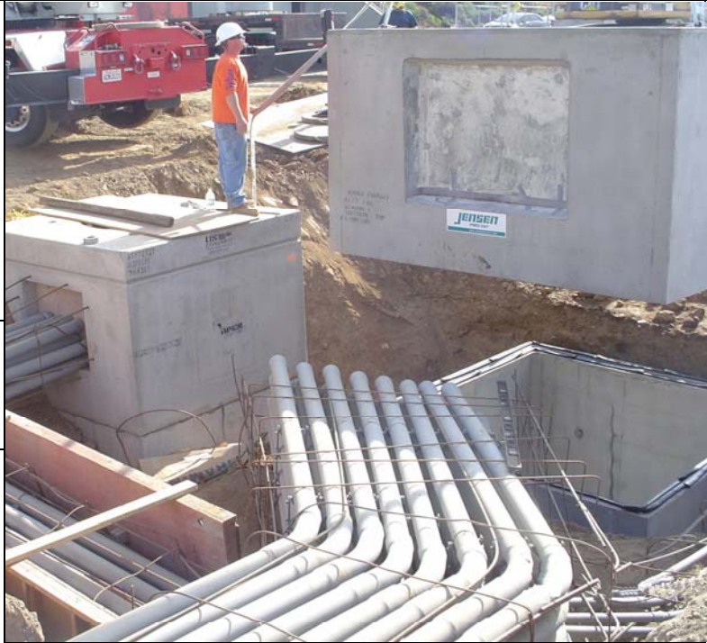
Placement of precast electrical vault
