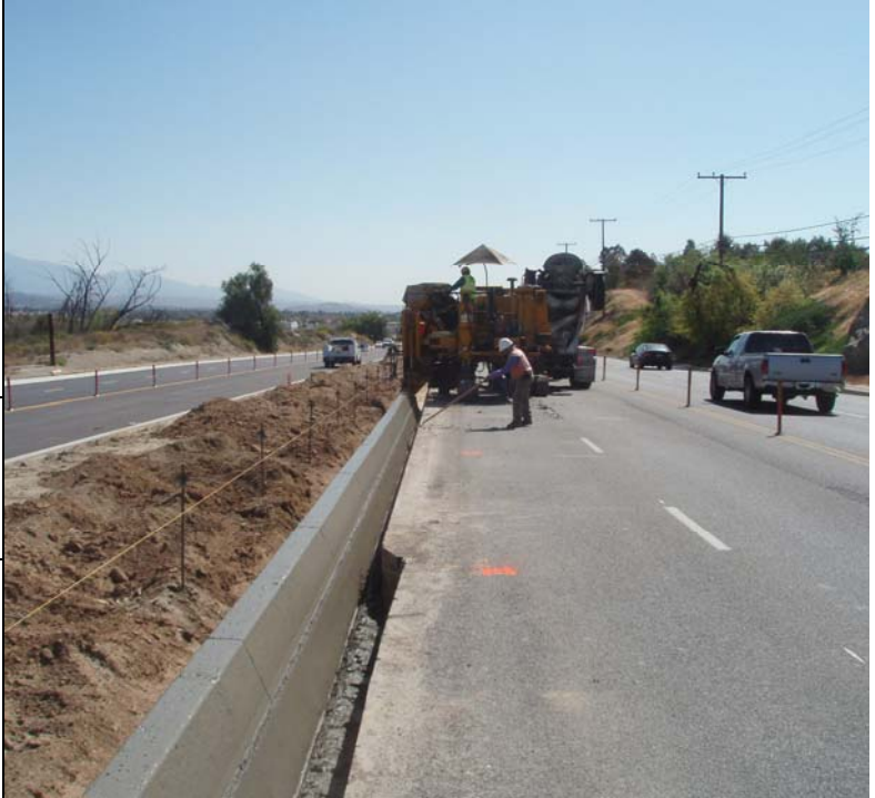
Placement of median curb on Alessandro Blvd.
