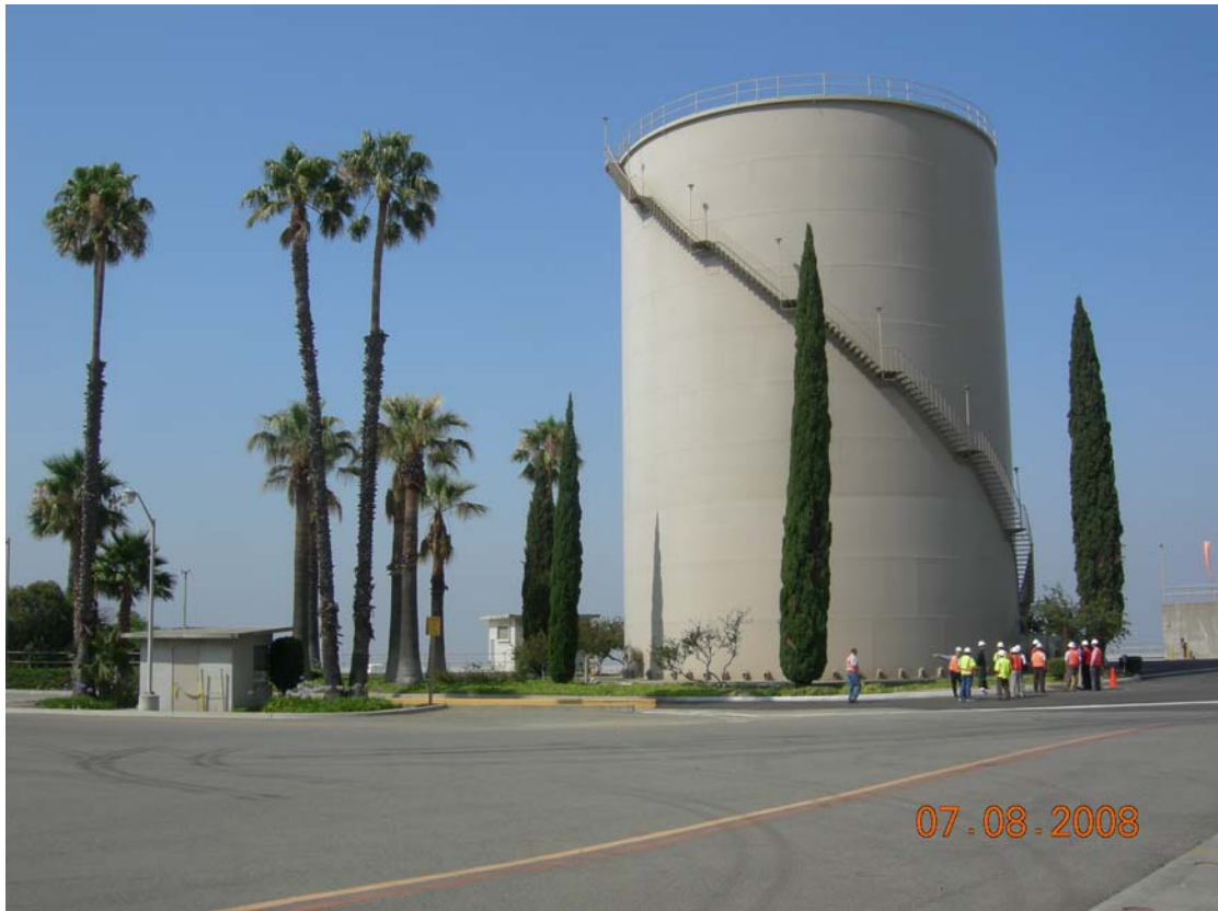
Figure 6: Washwater tank to be seismically upgraded
