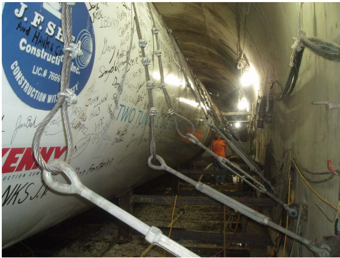
Figure 2: AWT – Installation of last piece of pipe in Arrowhead West Tunnel
