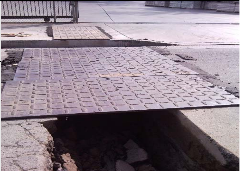
Excavated trench pipe trench for new pipe located in Burbank
