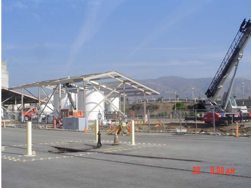
Figure 8: Weymouth new polymer tank farm construction – looking northwest
