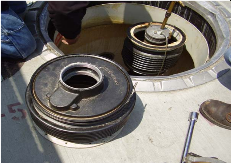
Installation of spill bucket at Mills Plant
