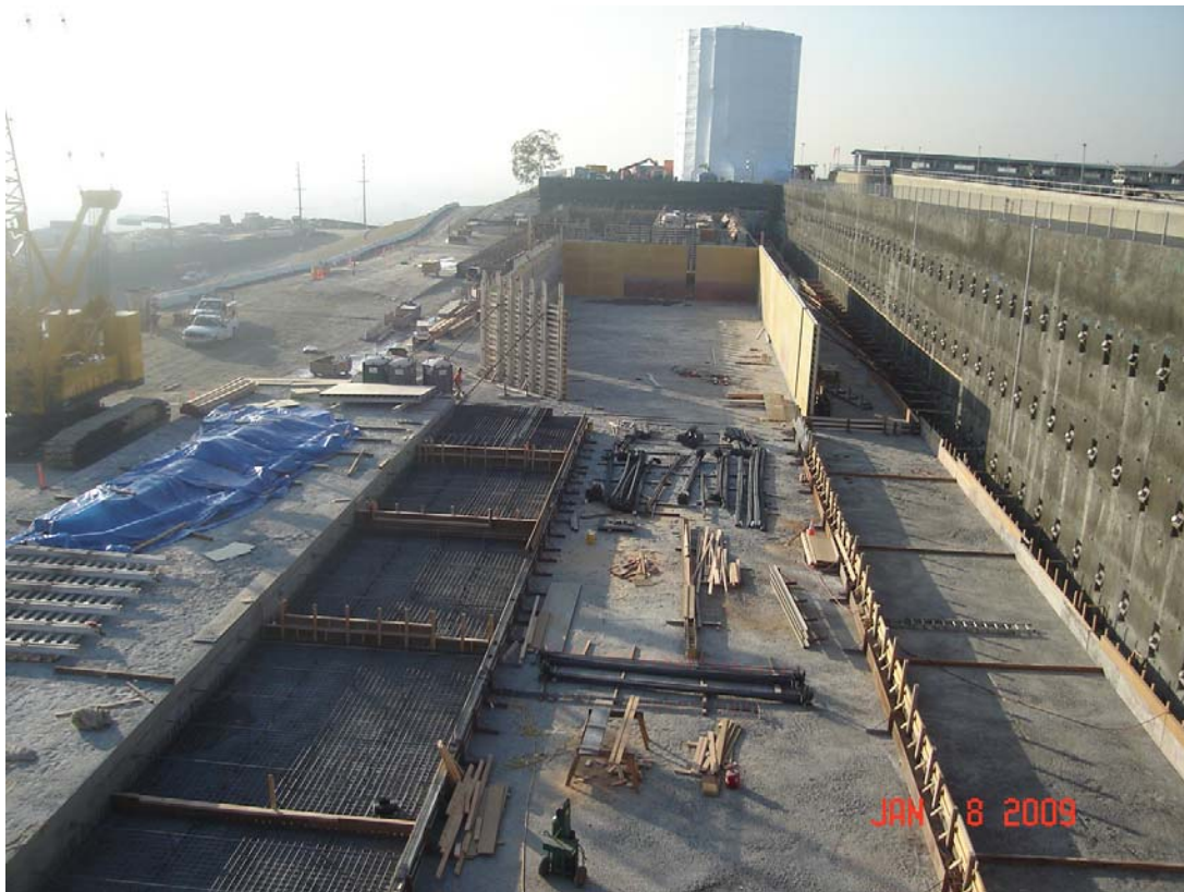
Figure 10: Diemer ORP contactor formwork construction
