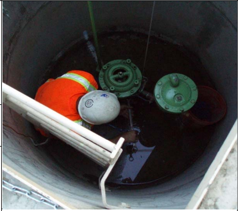
Removal of existing 4-inch vacuum valve located in Sun Valley
