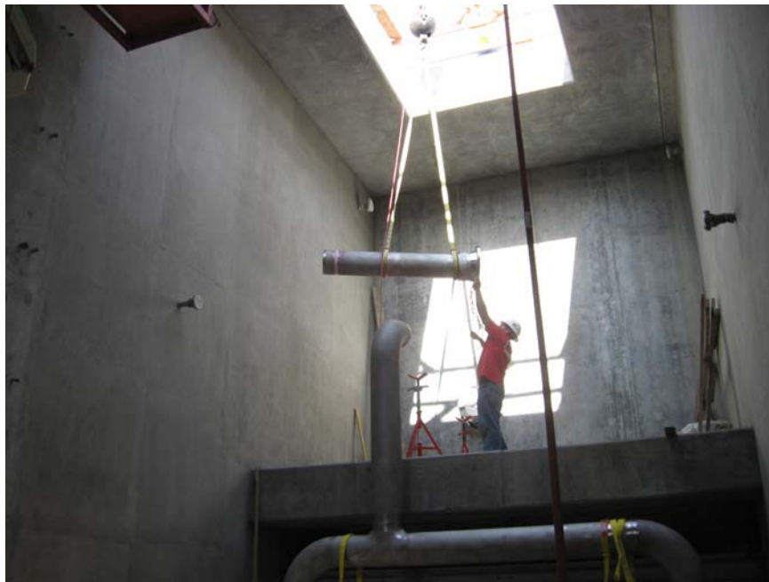
Figure 3: Installation of ozone piping in Contactors Nos. 3 and 4
