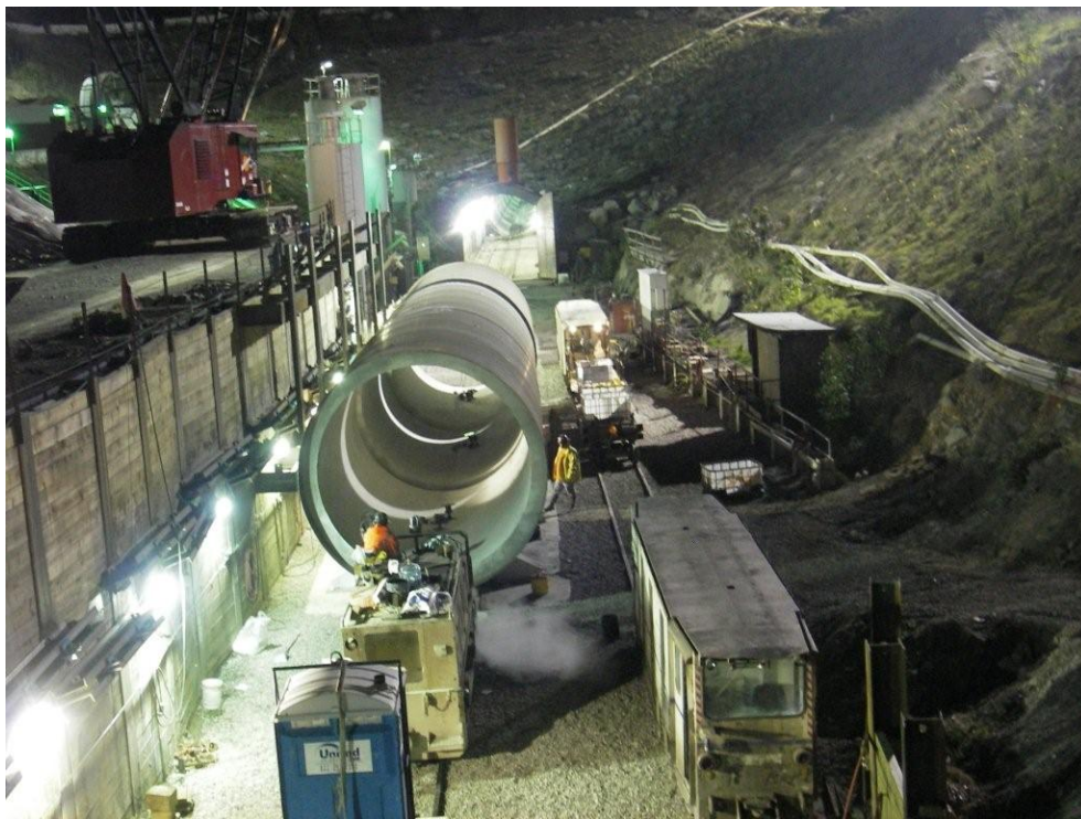
Figure 2: RCCP being transported into AWT at Waterman Canyon Portal
