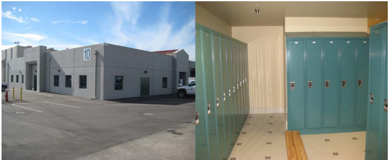
Figure 9: Completed Weymouth Plant Operations and Maintenance Center
