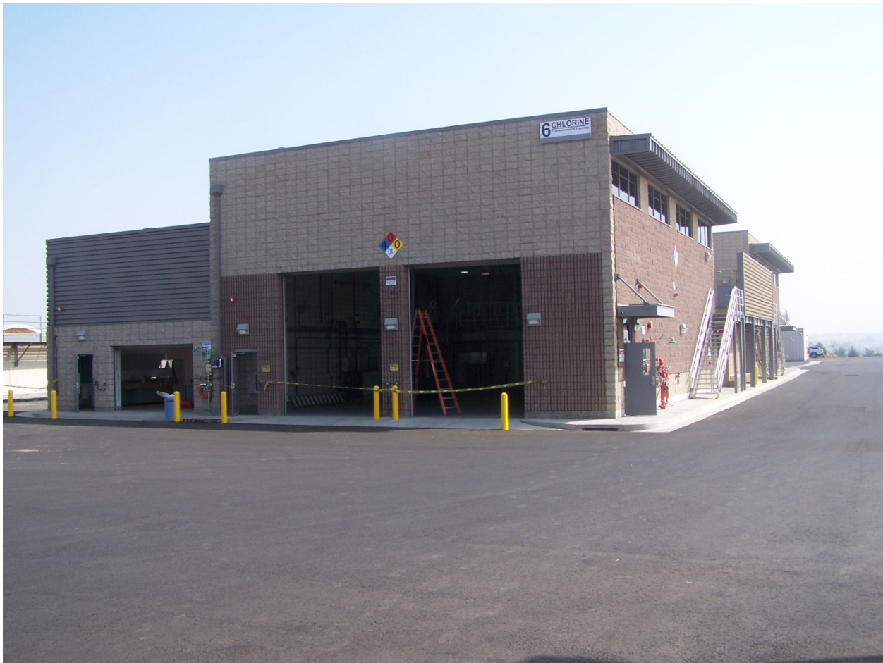
Figure 11: Recently completed Mills Chlorine Containment Facility
