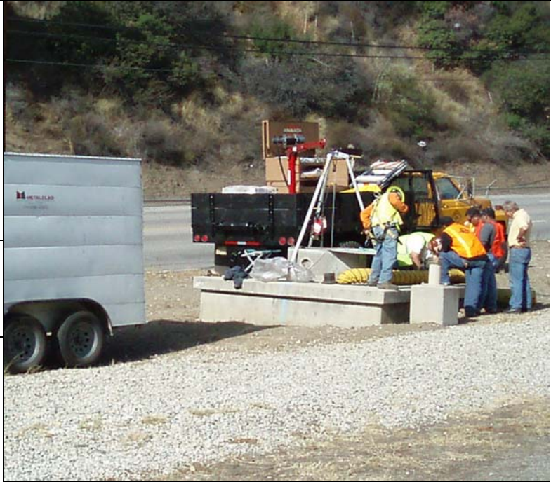
Removal of 8-inch vacuum valve located in the city of Los Angeles
