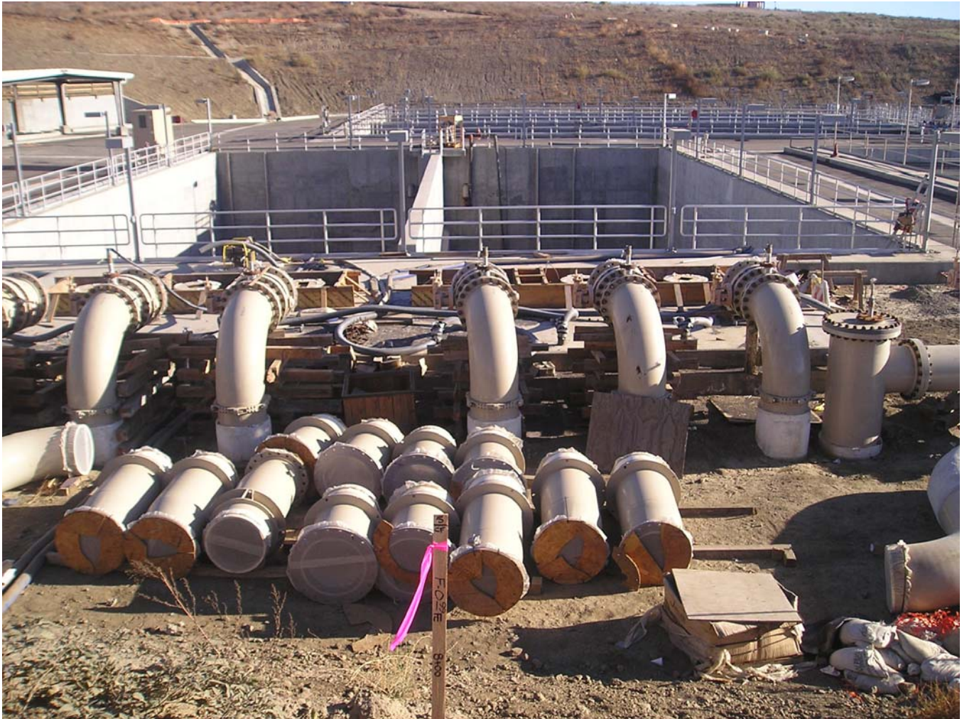
Figure 5: Construction of reclaimed washwater return pumping station
