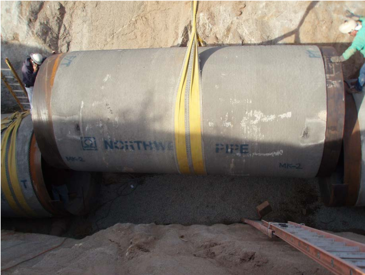
Figure 1: Installation of last pipe segment for Perris Valley Pipeline North Reach
