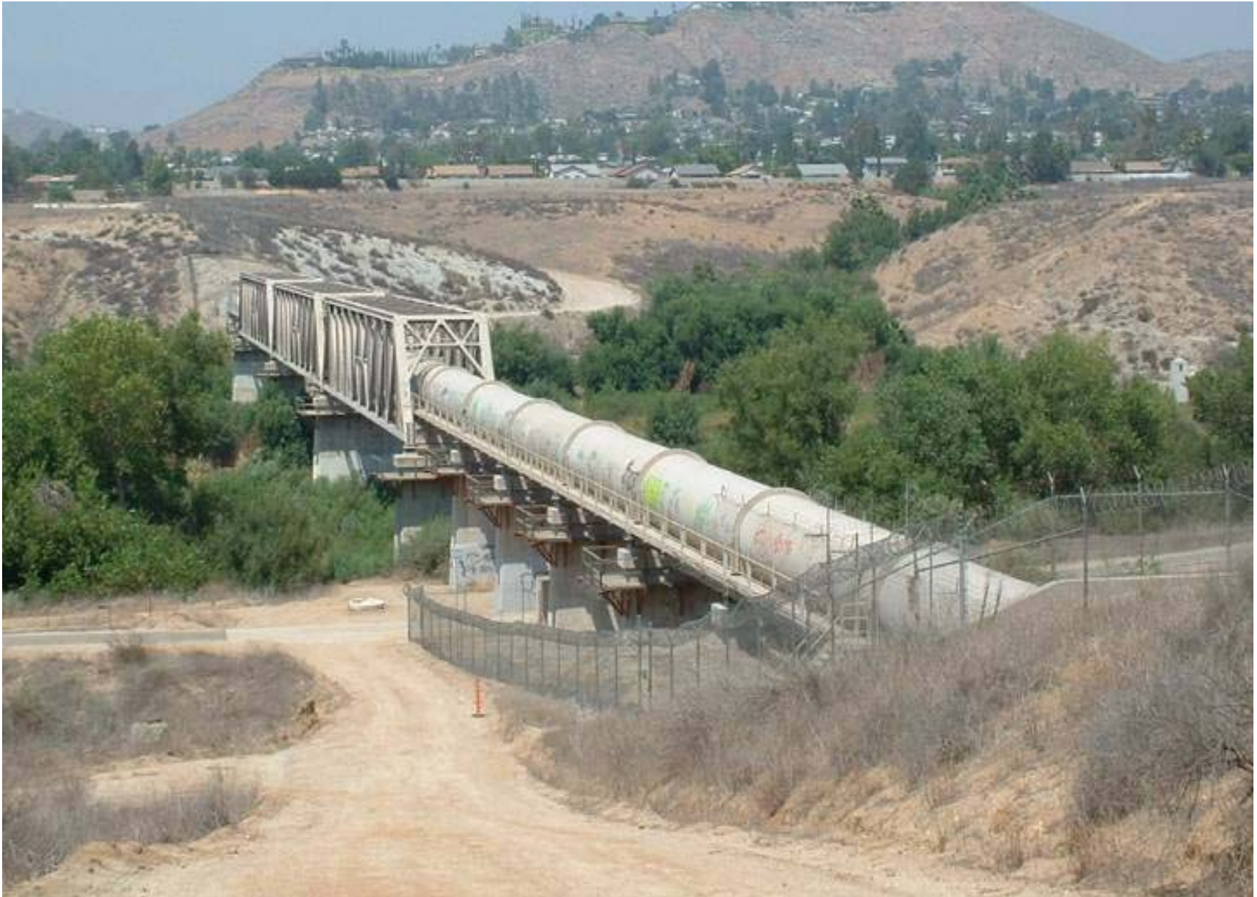
Santa Ana River Bridge and Upper Feeder
