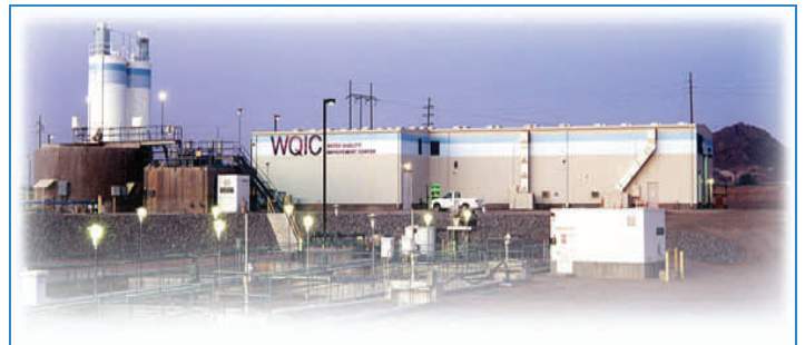
Yuma Desalting Plant
