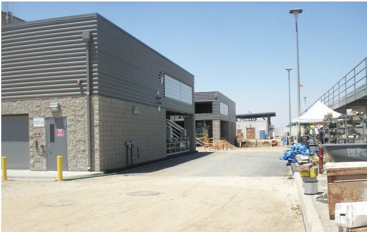
Figure 13: Mills Chlorine Containment facility nearing construction completion
