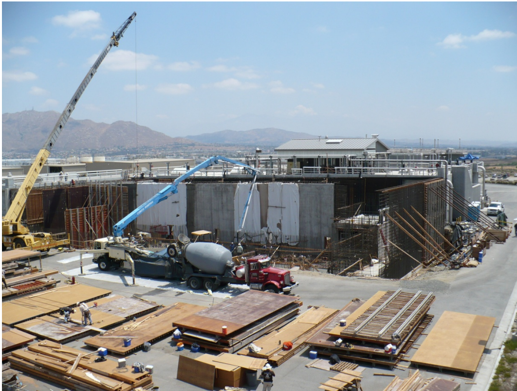
Figure 3: Construction of Wall Forms for Contactor Chambers
