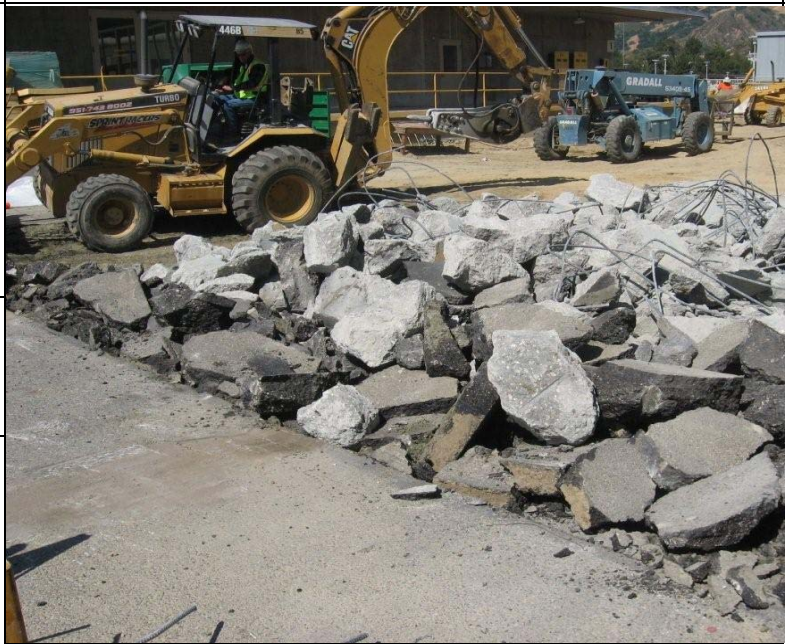
Demolition of caustic unloading pad
