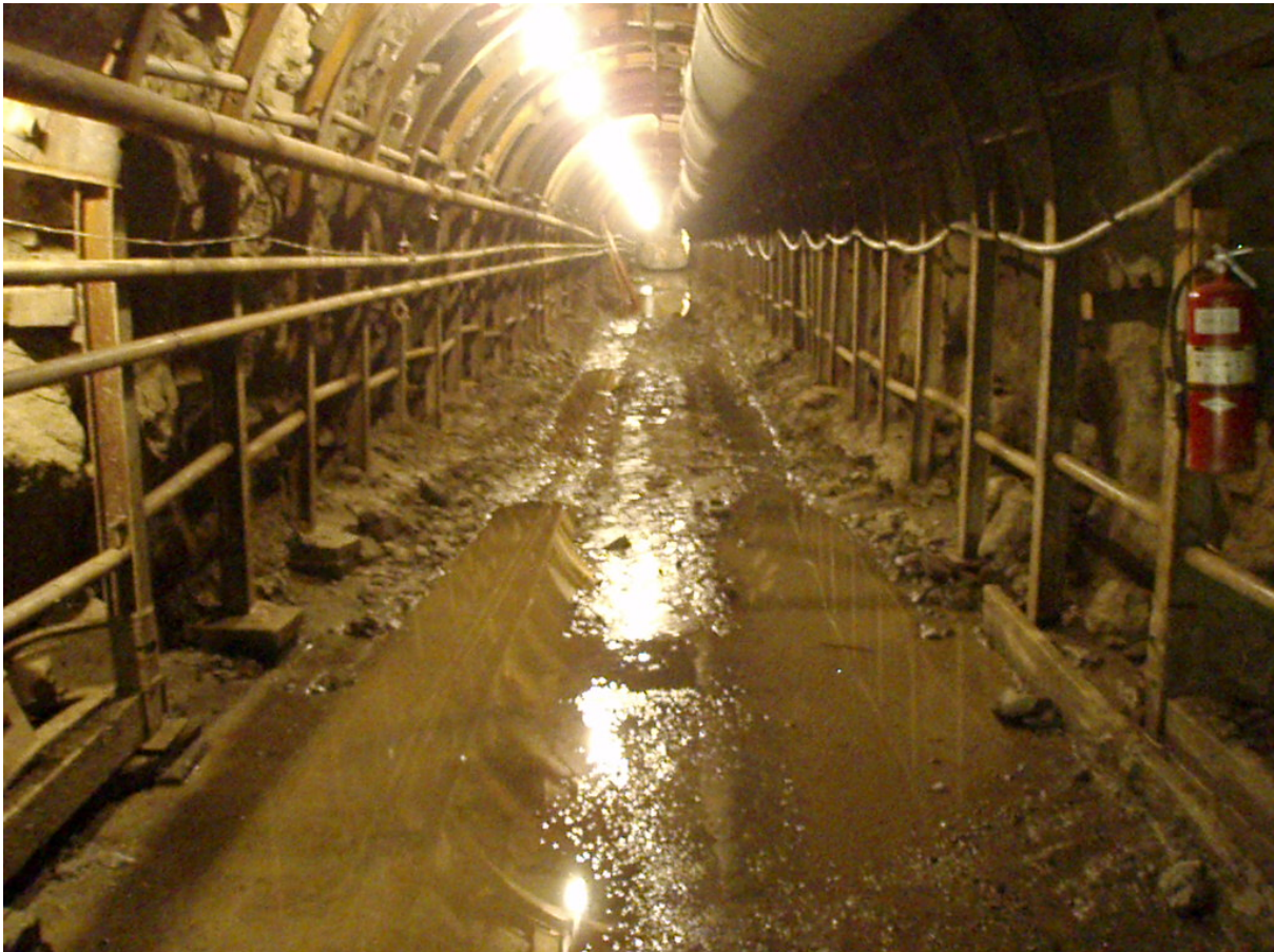
Figure 4: Tunnel at Alessandro Boulevard
