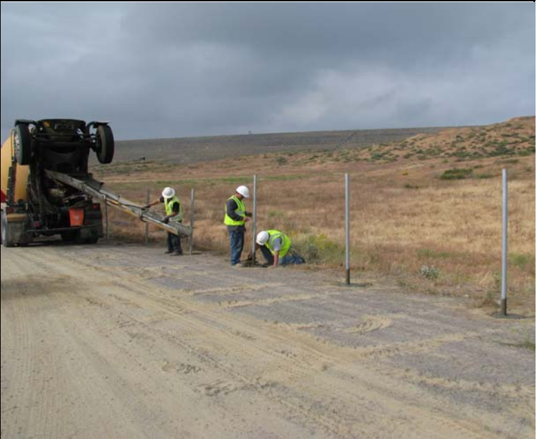
Placement of fence posts
