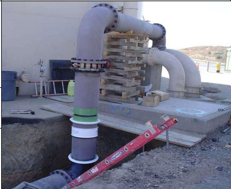
West Washwater Tank intertie bypass line
