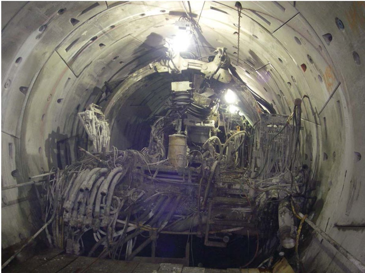
Figure 2: Dismantling and removal of the TBM at Arrowhead East Tunnel
