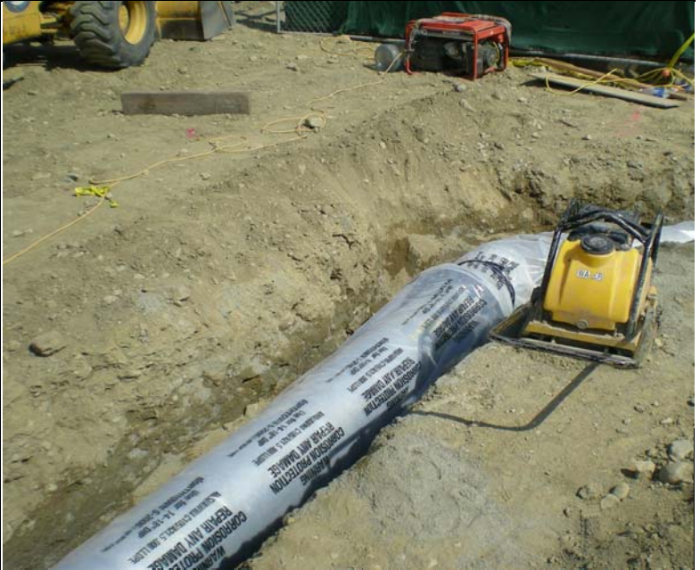
Installation of 16-inch air intake
