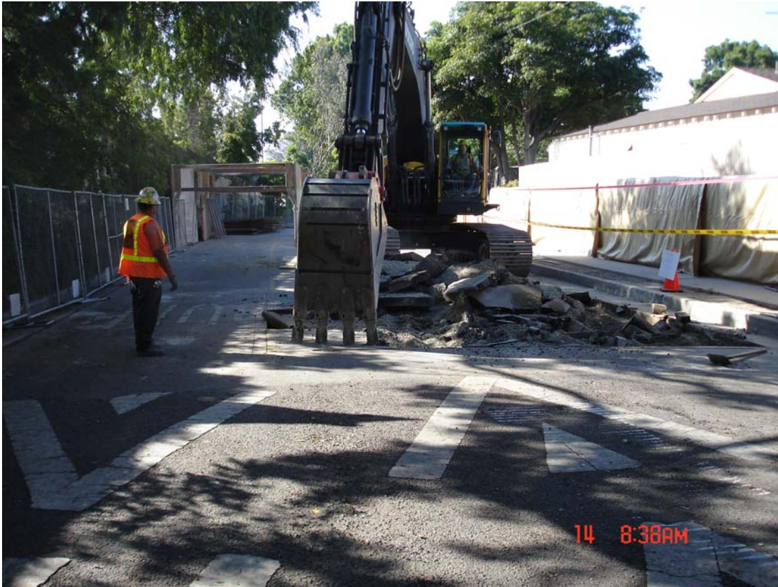
Figure 1: Excavation underway at the Sepulveda Feeder
