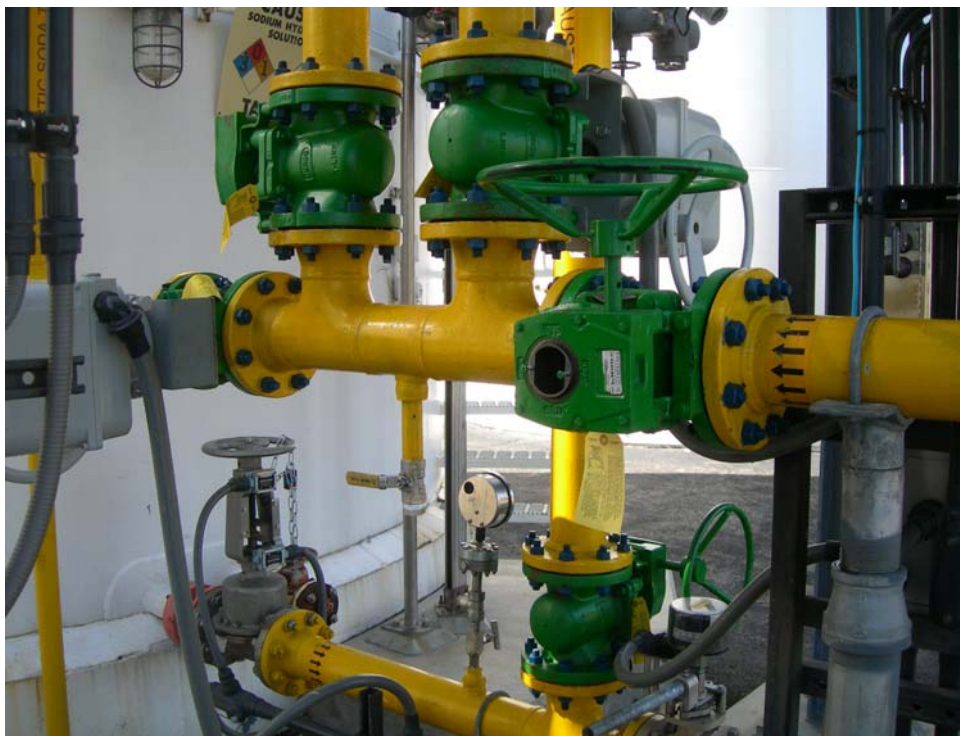
Figure 7: Valve replacement at Jensen plant
