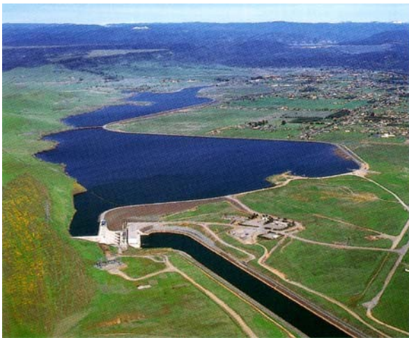
Figure 2. Thermalito Forebay and Power Plant (DWR Photo.)
