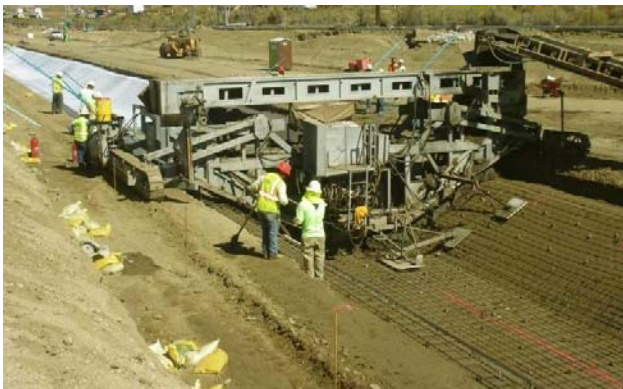
Figure 5. Gorman Creek Improvement Channel liner replacement. (DWR Photo.)
