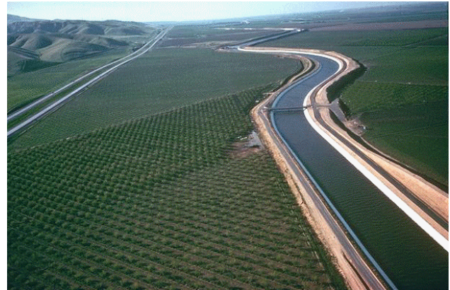
Figure 12. California Aqueduct in the San Joaquin Valley. (DWR photo.)
