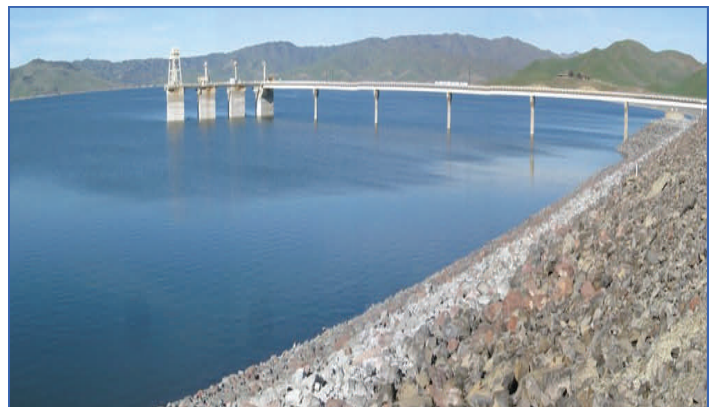
San Luis Reservoir Outlet Tower
