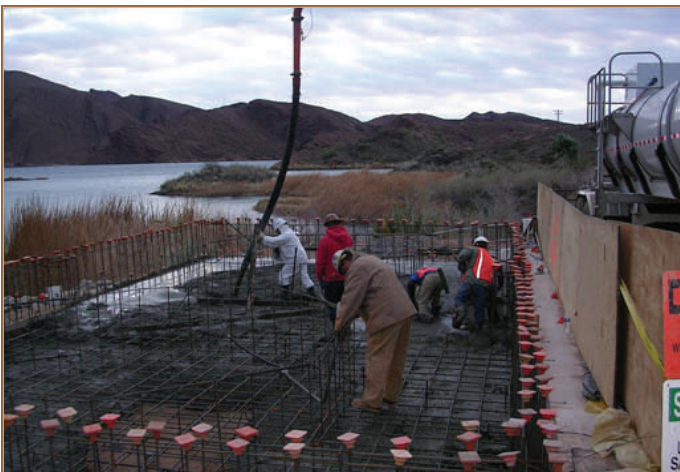
Copper Basin Sodium Hypochlorite Tank Storage Slab Being Placed
