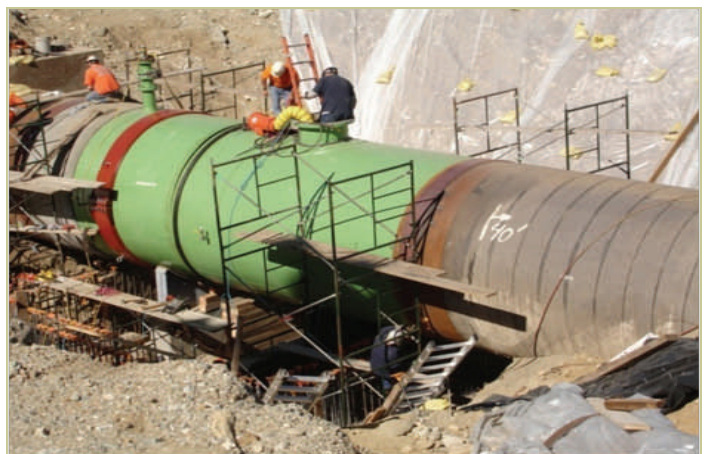
Rialto Pipeline Rollout
