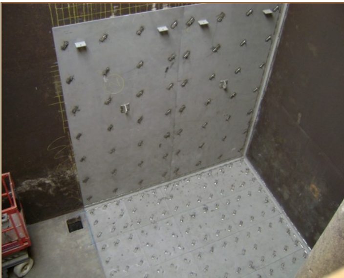
Stainless Steel plate installation for service connection LA35 at discharge structure.
