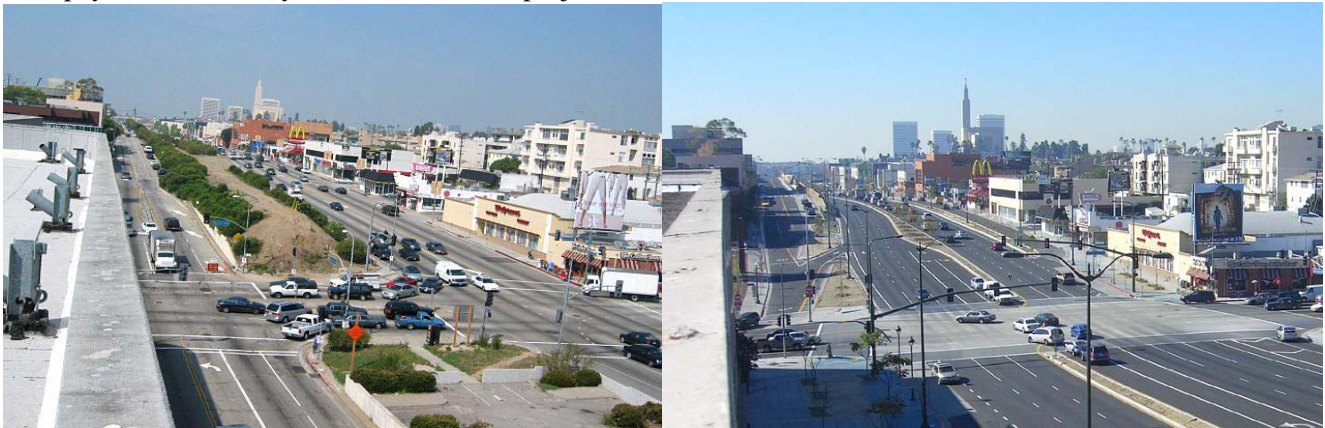
Figure 1: Before and after views of intersection of Santa Monica Boulevard and Beverly Boulevard
