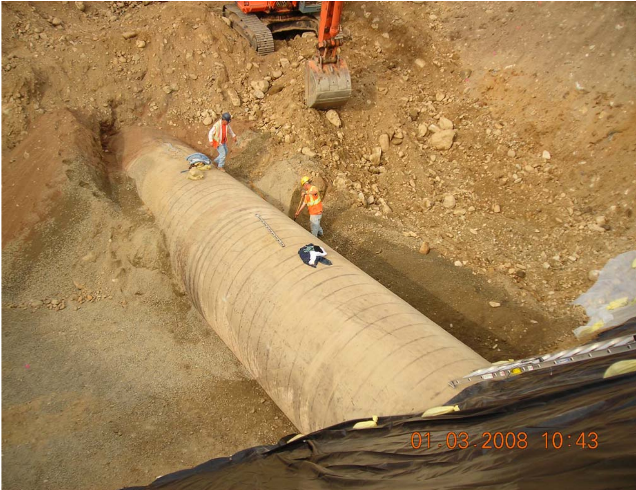
Figure 5: Excavation underway at Site No. 2 in the City of Upland
