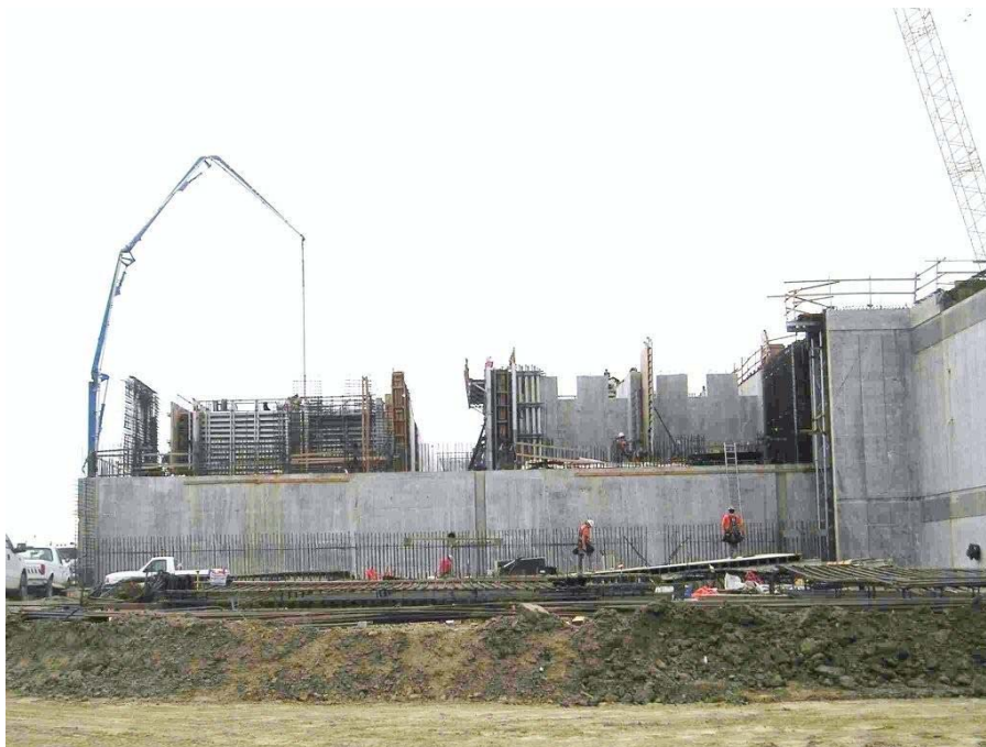
Figure 11: Skinner ORP inlet control structure construction
