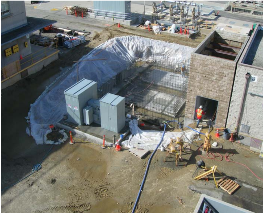
Figure 12: Construction of the foundation for the Jensen scrubber pad units
