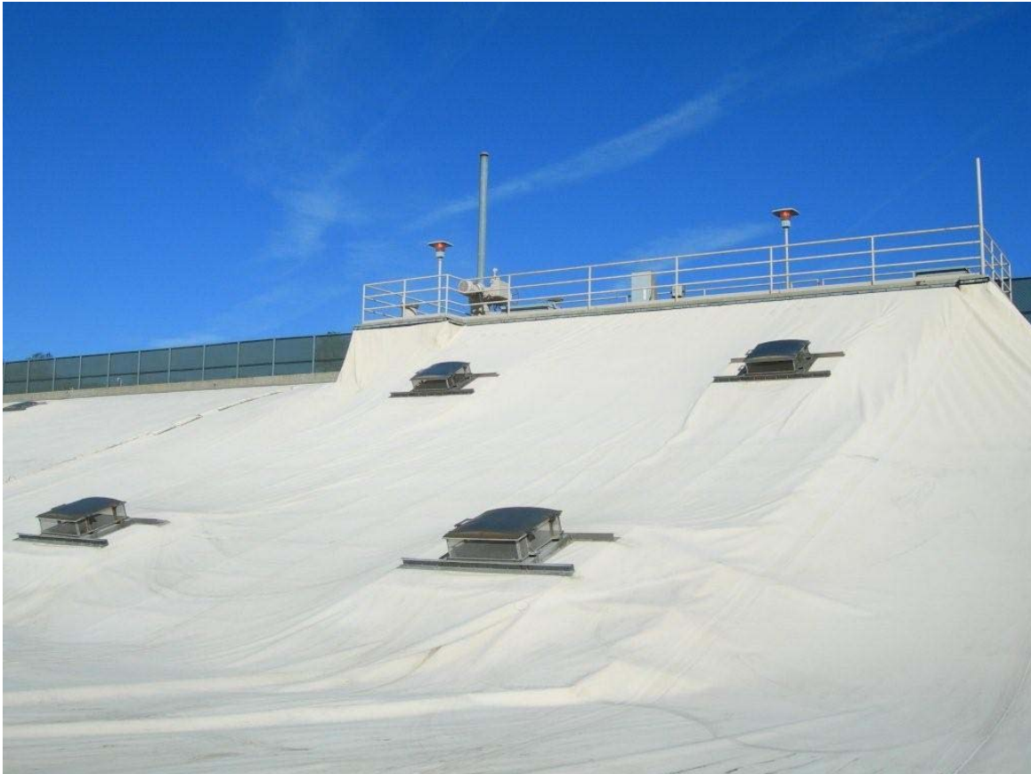
Figure 9: Existing floating cover at Jensen Finished Water Reservoir No. 2
