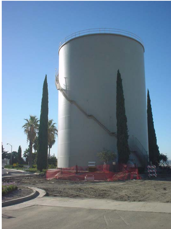
Figure 8: Diemer East Washwater Tank
