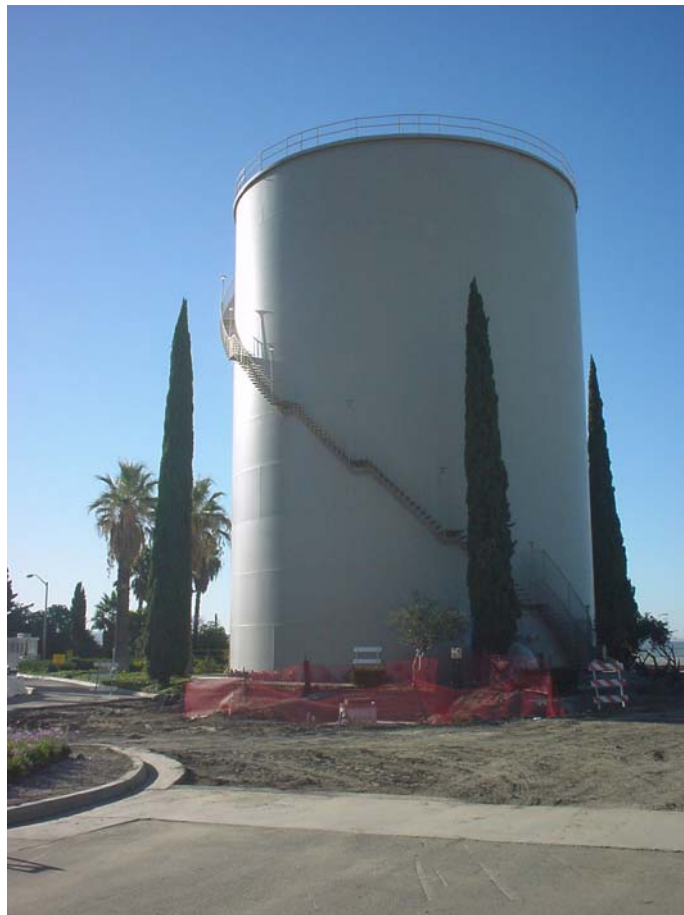
Figure 8: East Washwater Tank
