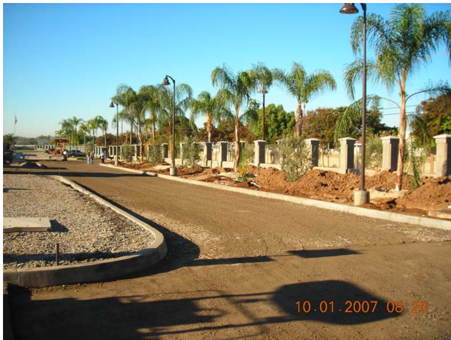
Figure 9: West side (Moreno avenue) of Weymouth perimeter improvements
