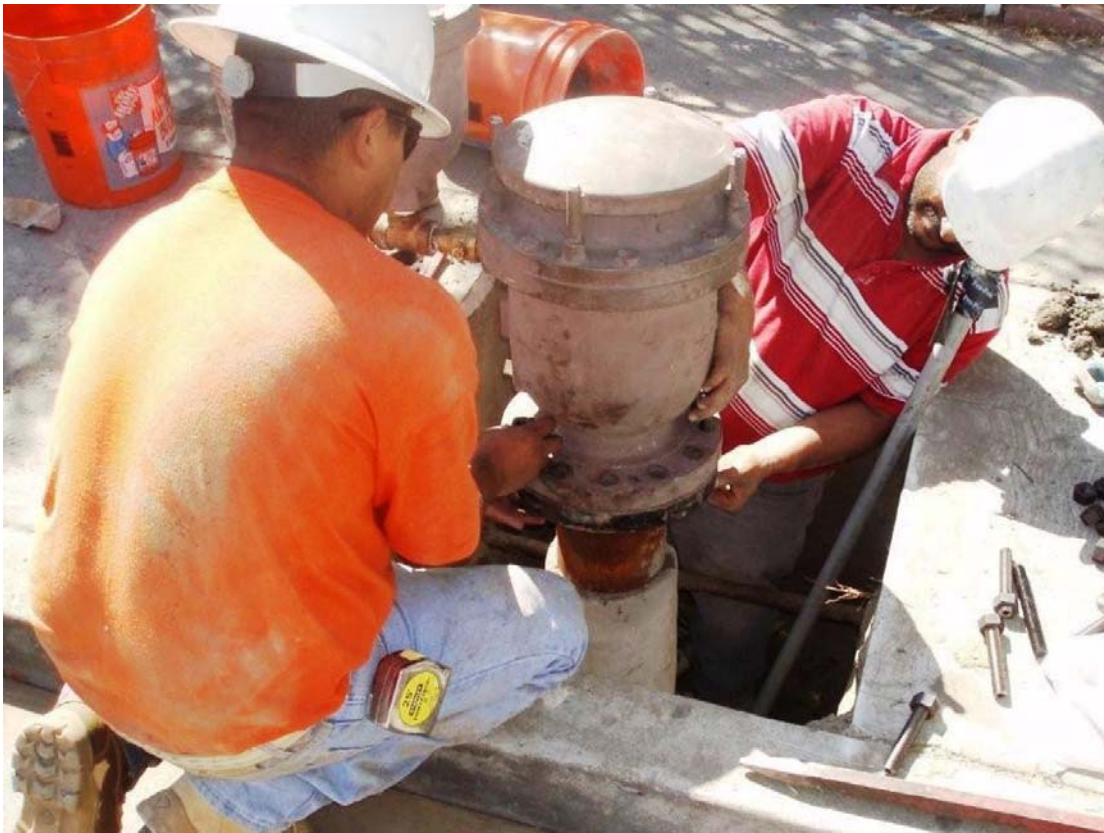
Figure 10: Removing air-vacuum relief valve
