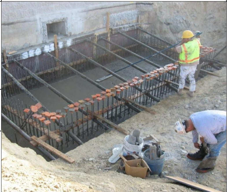
Placement of concrete for new electrical room vault
