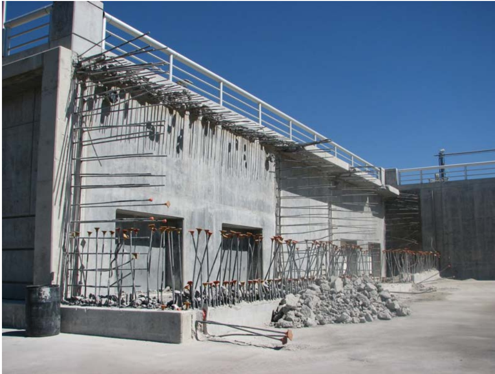
Figure 5: Demolition of concrete around existing rebar dowels for Mills Contactors Nos. 3 & 4
