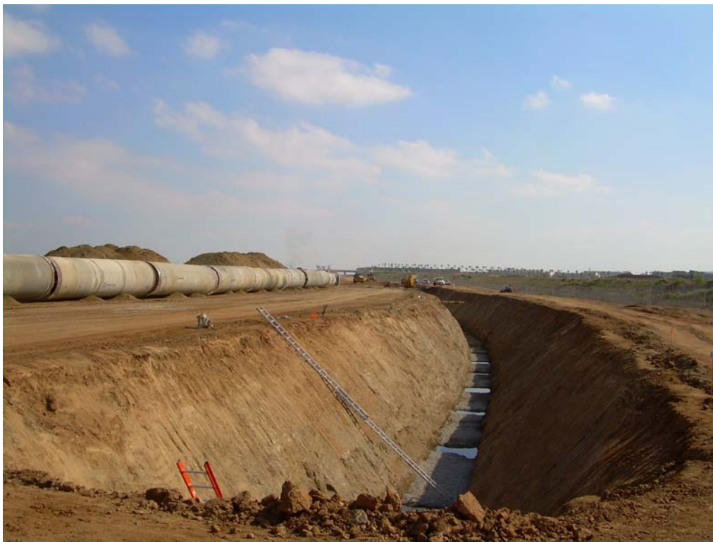
Figure 2: Perris Valley Pipeline North Reach construction
