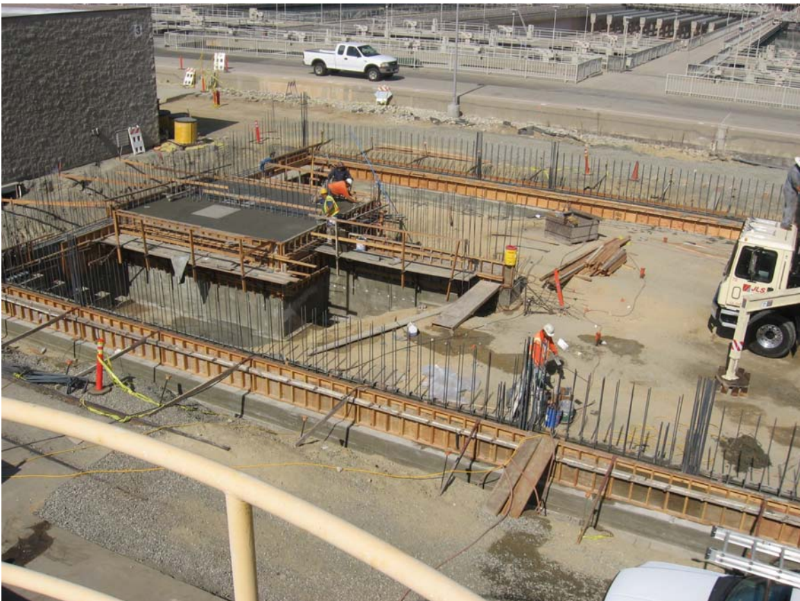
Figure 12: Concrete formwork for railcar storage building at Jensen
