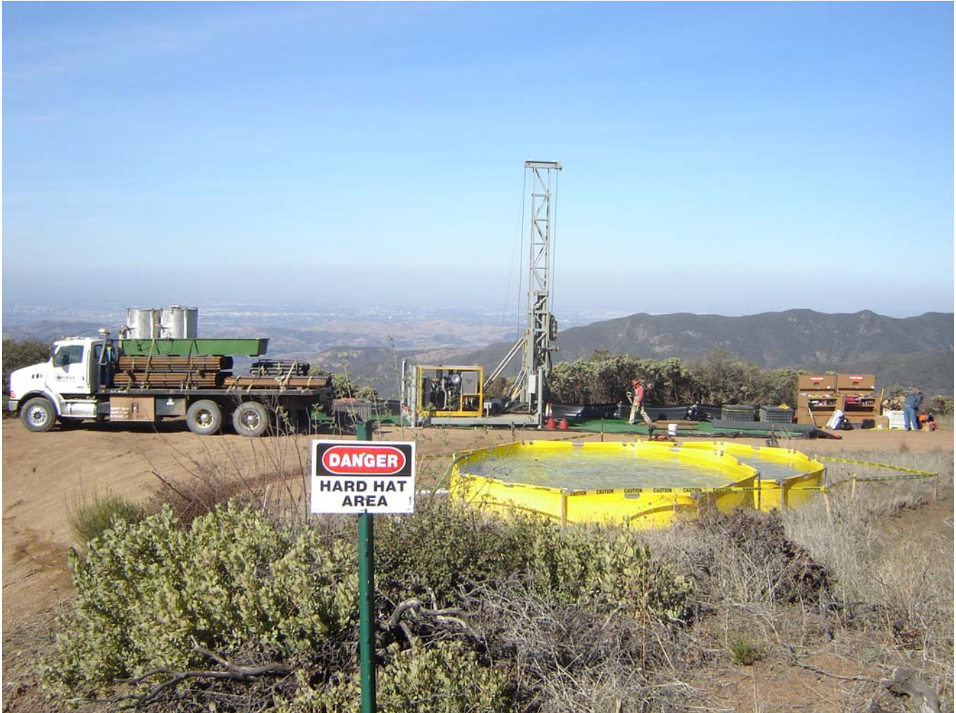
Figure 3: Drill site for Borehole No. C-1
