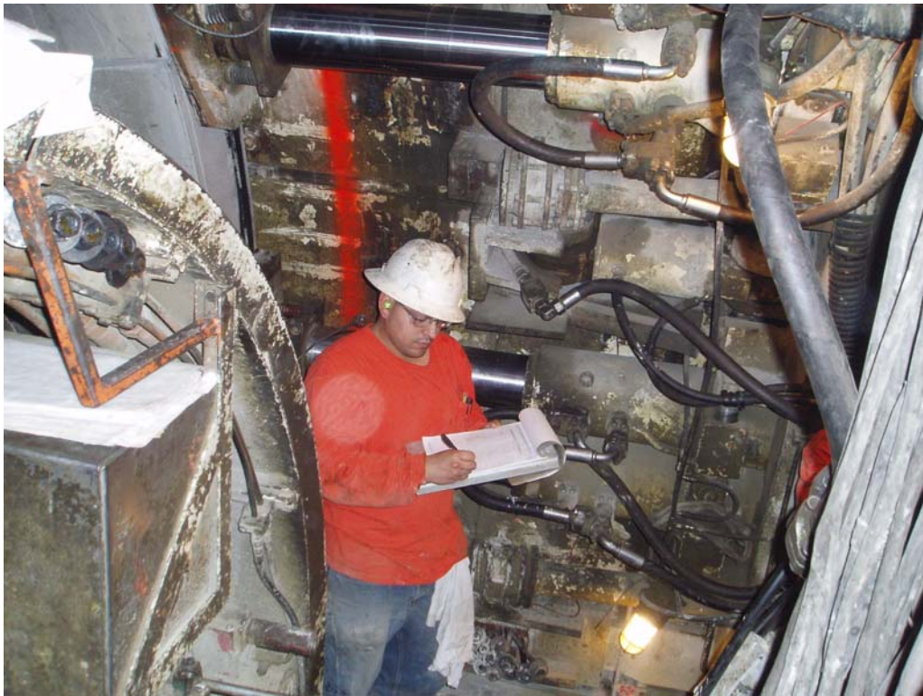
Figure 4: Inspection of Arrowhead East Tunnel
