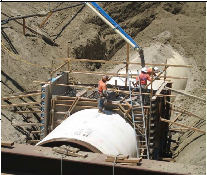
Concrete placement for manhole on Plant 2 inlet conduit
