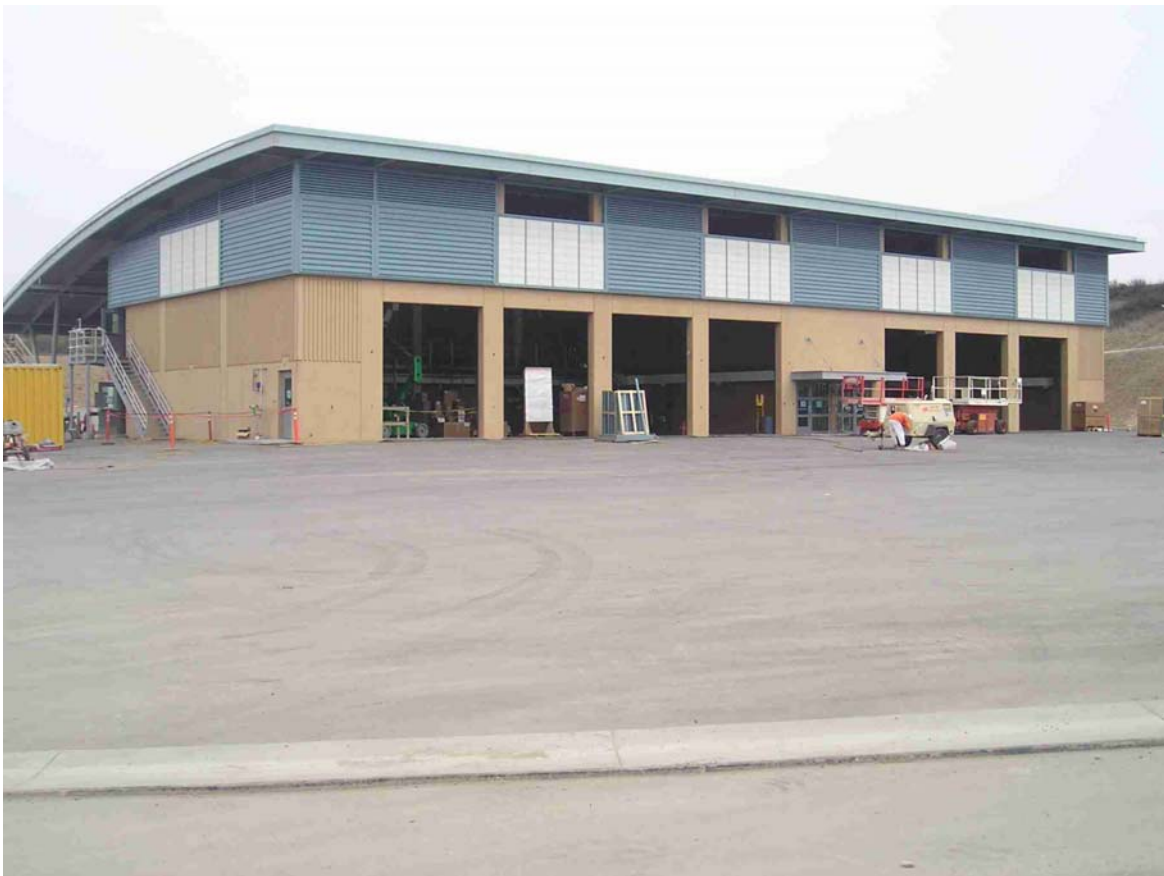
Figure 13: Skinner Chlorine Containment Facility
