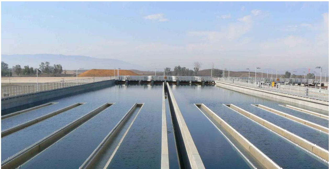
Figure 7: Module No. 7 sedimentation basin (looking south)
