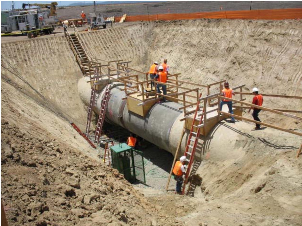
Figure 8: Newly installed pipe segment on San Diego Pipeline No. 5
