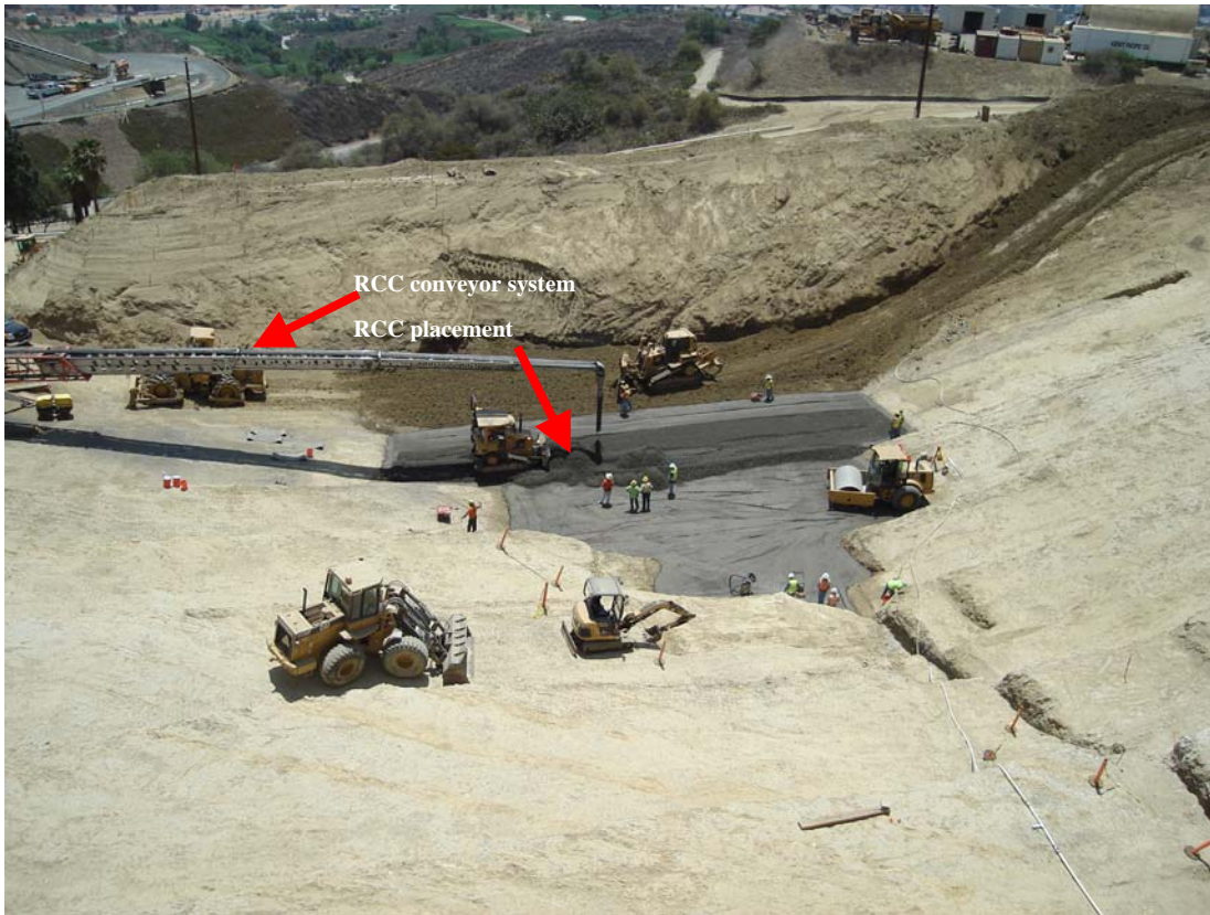
Figure 1: First Roller Compacted Concrete placement at Diemer plant
