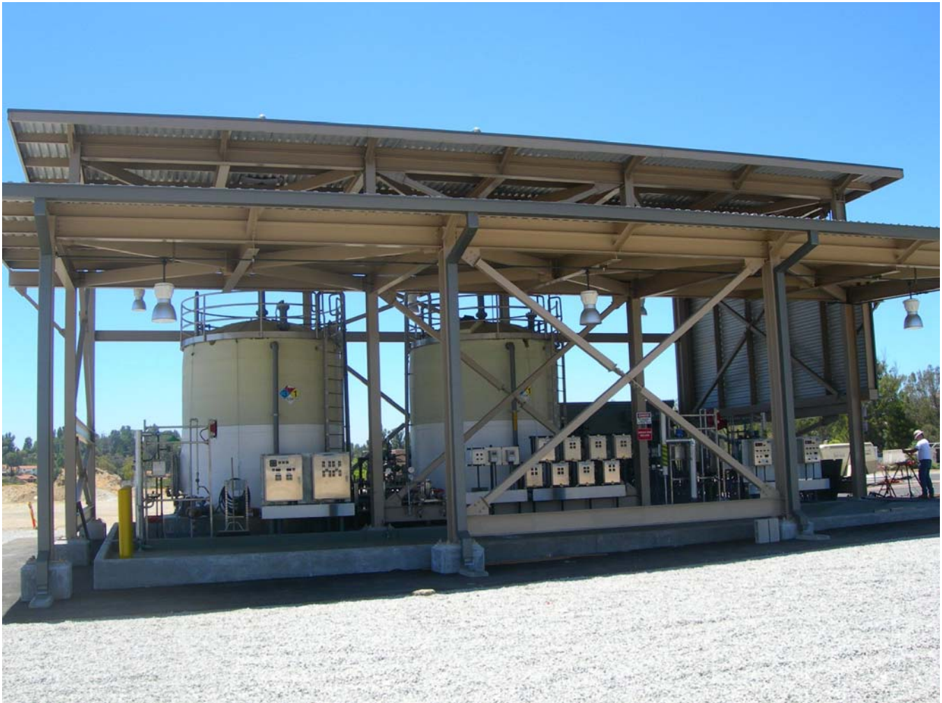
Figure 12: Jensen fluoride tank covered by roof structure
