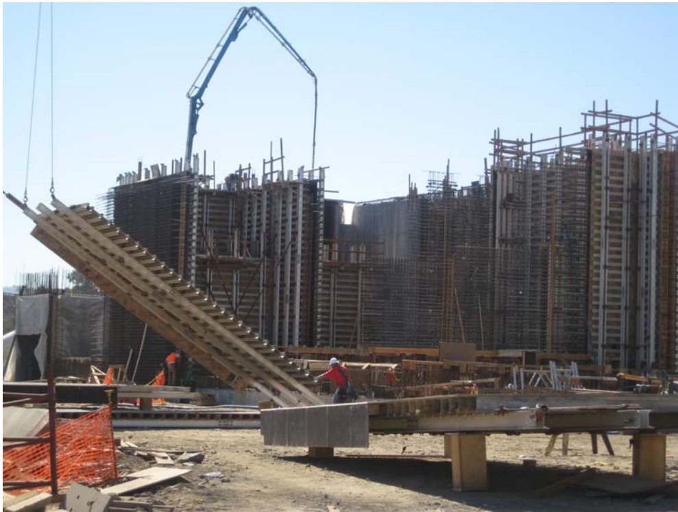
Figure 11: Skinner ozone contactor construction
