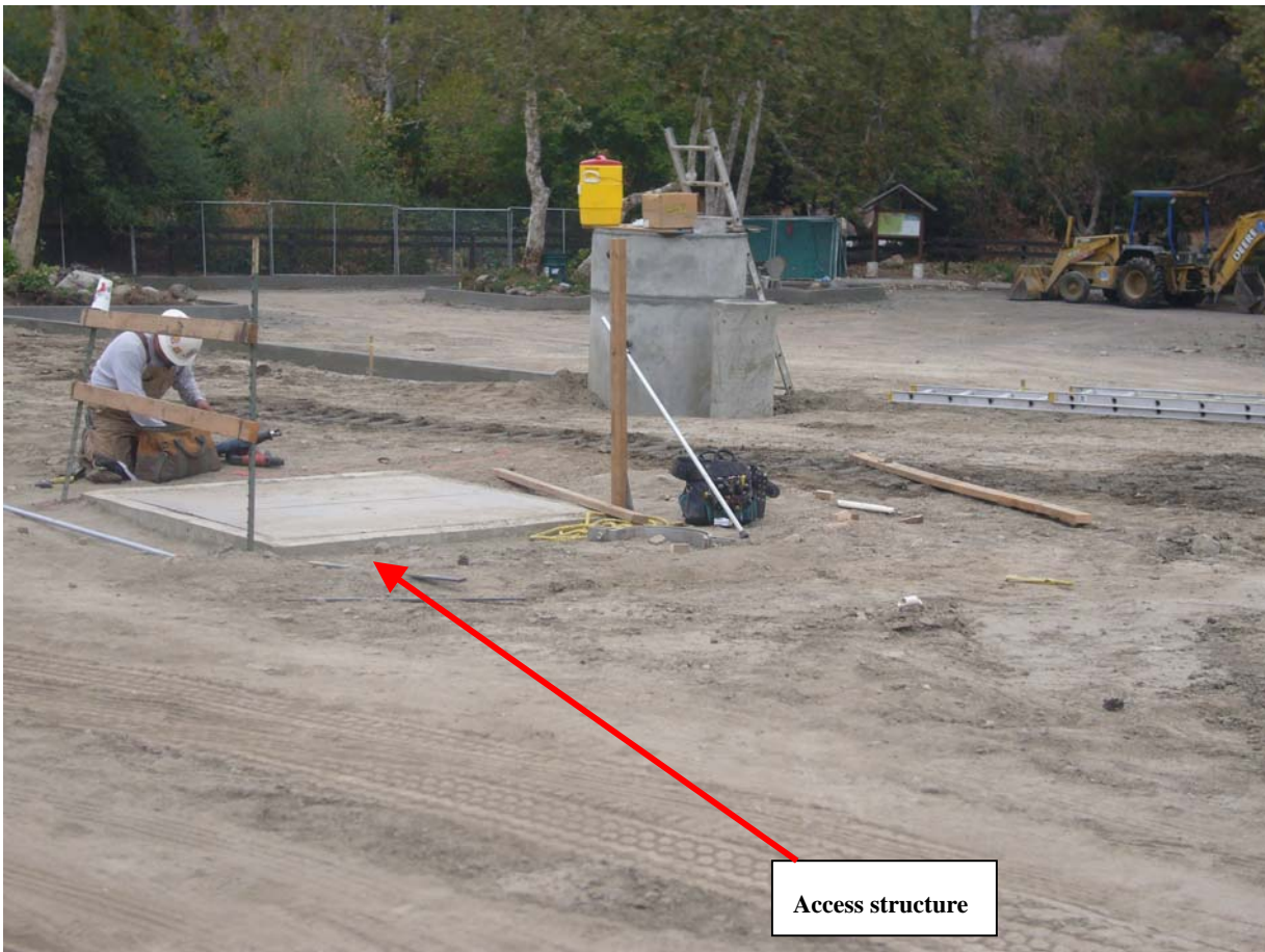
Figure 6: Access for Structure No. 3 in the City of Claremont
