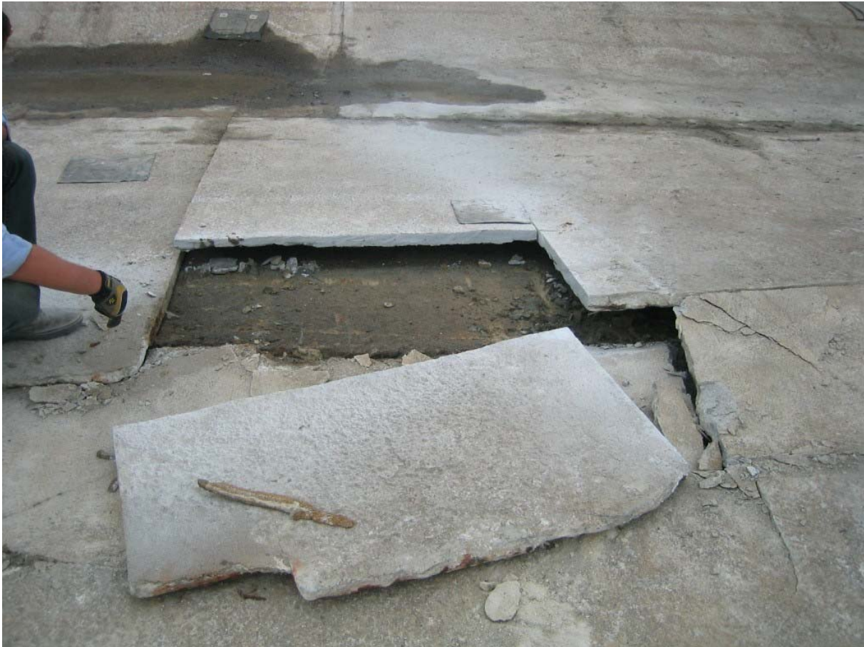
Figure 5: Concrete liner to be repaired at the Orange County reservoir
