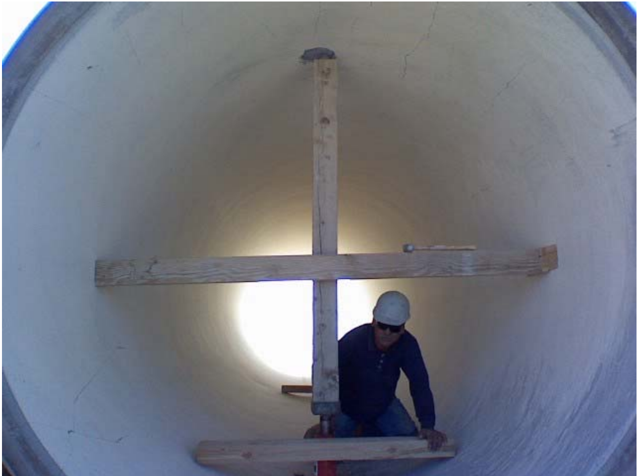
Figure 5: Completed pipe section
