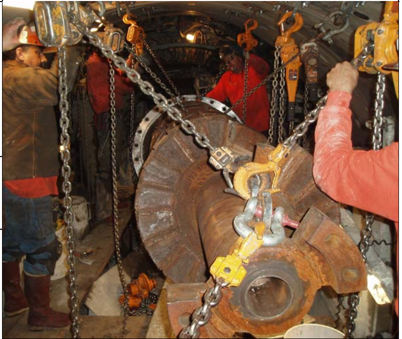
Installation of new auger section on Arrowhead West TBM
