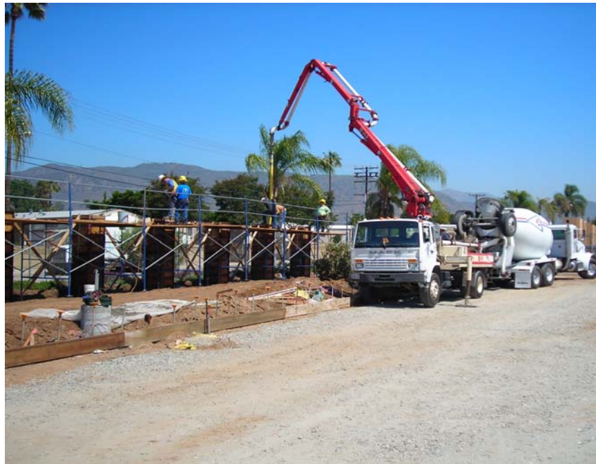
Figure 8: Concrete placement for pilasters at the Weymouth plant
