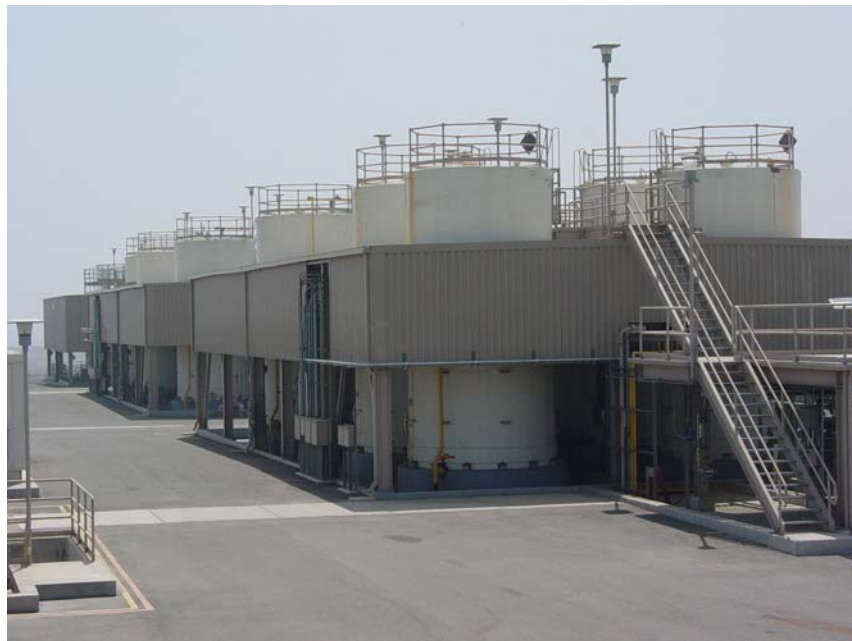
Figure 4: Existing alum-ferric chloride tank farm will be modified for 326 mgd capacity
