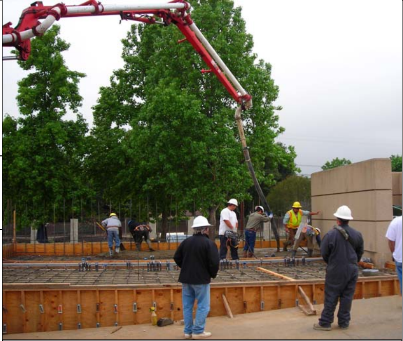
Concrete placement for slab-on-grade
