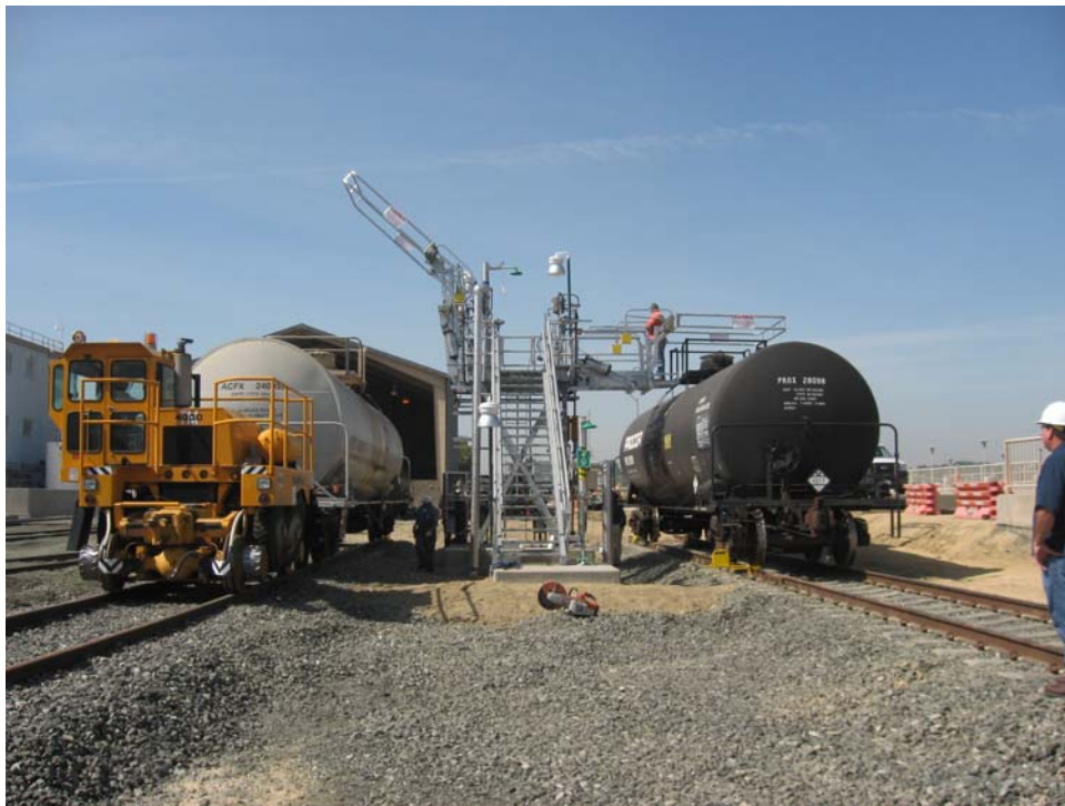
Figure 10: Temporary unloading platform field testing
