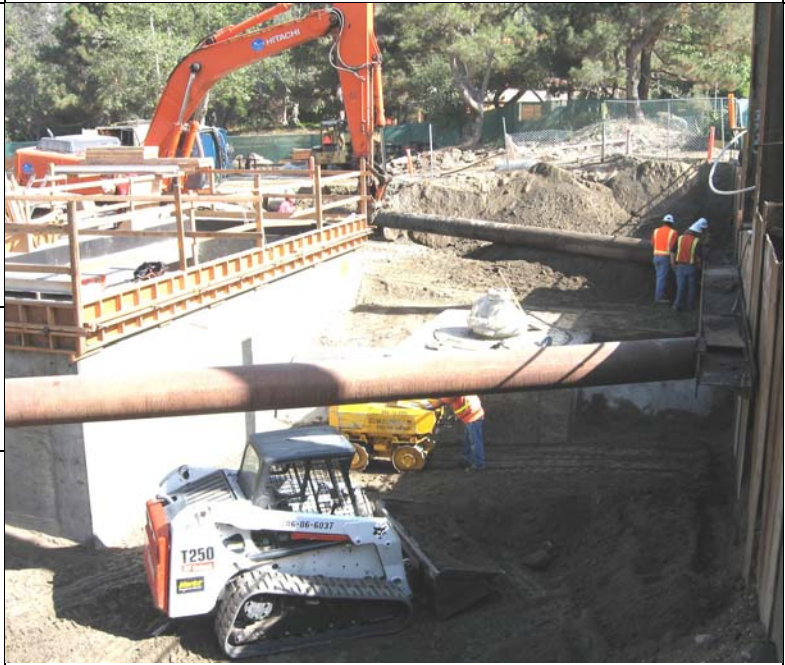
Backfill operation in progress
