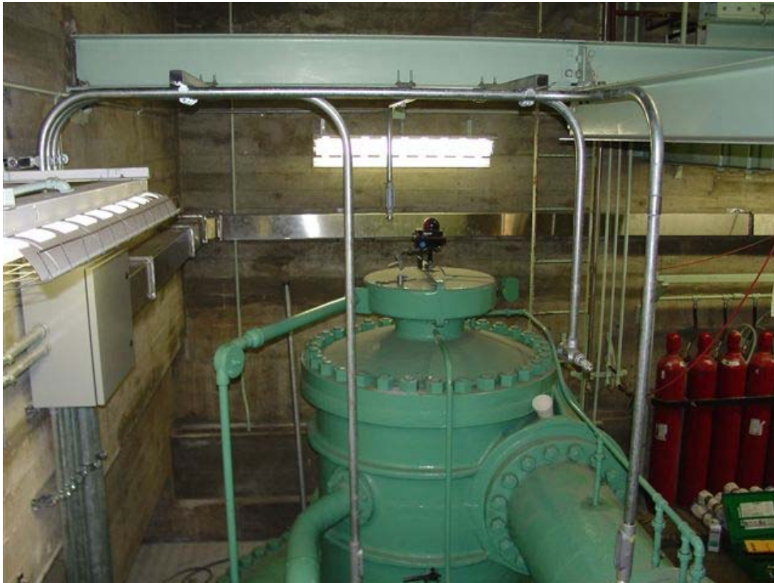
Figure 6: New installation at Unit 1 Pump Bay
