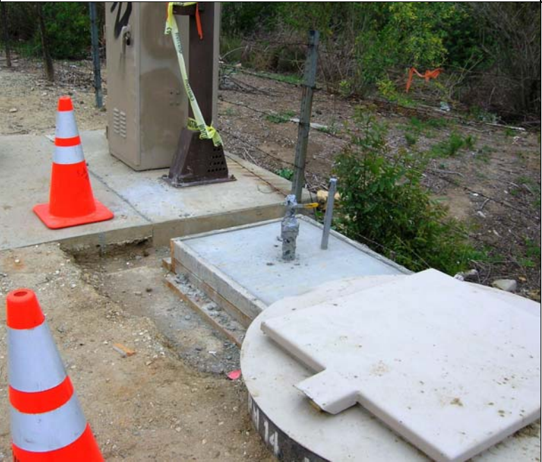
New foundation slab and brass piping at site in Los Angeles County
