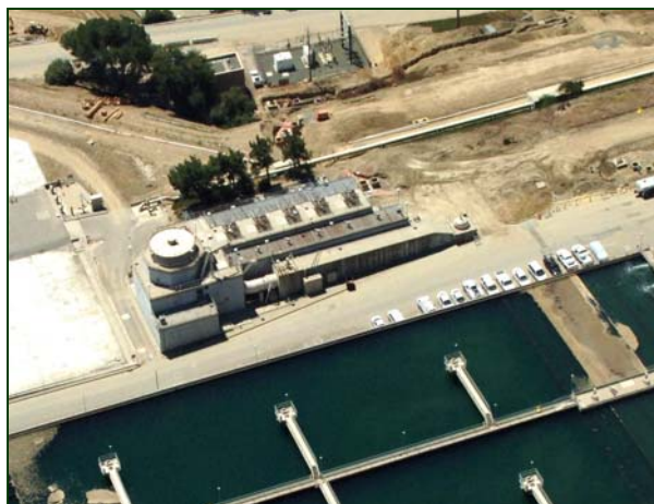
Yorba Linda Power Plant
