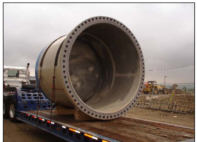
Bulkhead to be installed at a future sectionalizing valve location on the Rialto Pipeline
