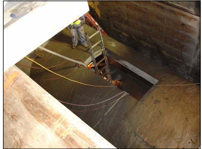
Contractor preparing to cut the pipe on the Rialto Pipeline
