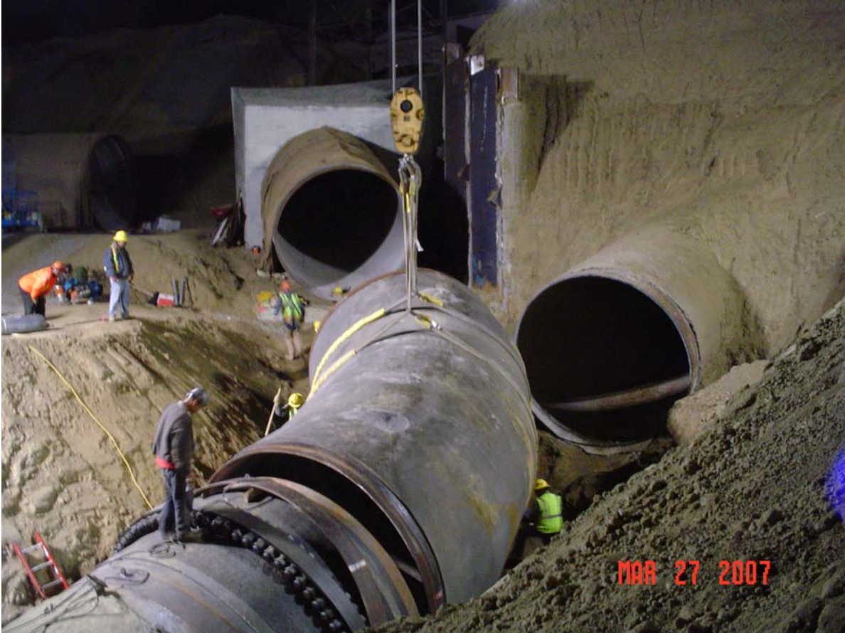
Figure 1: Diemer plant inlet conduit tie-in
