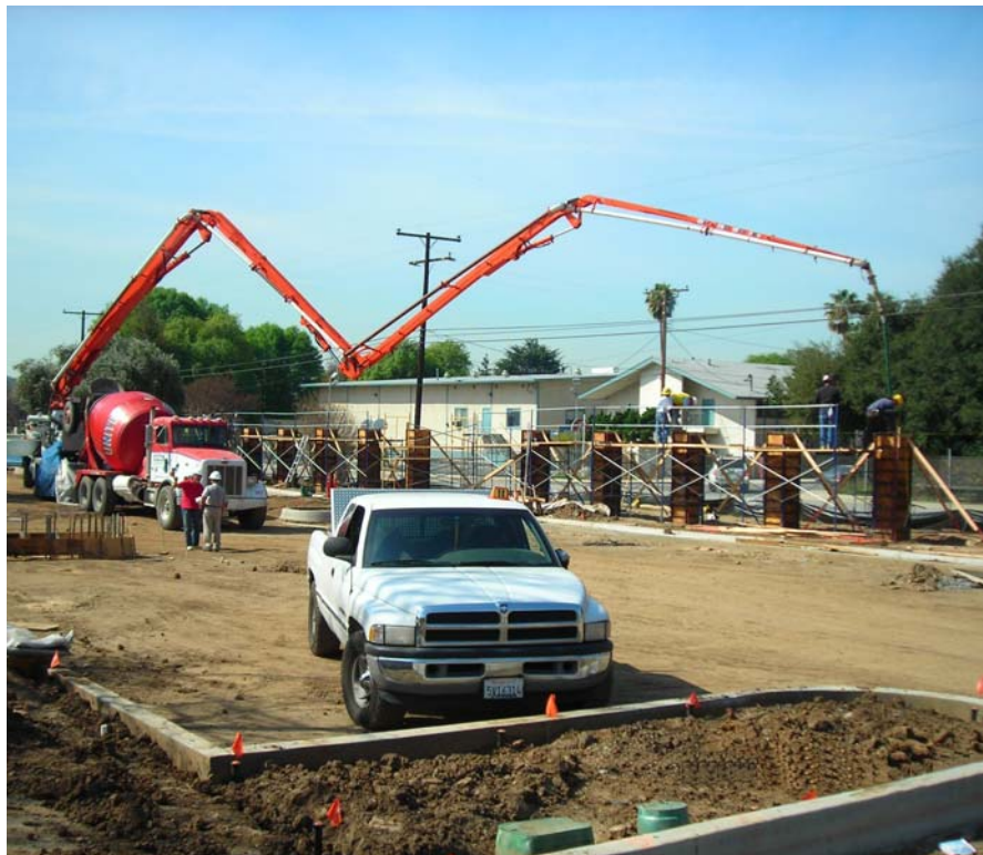
Figure 11: Concrete placement for decorative fence columns at Weymouth plant
