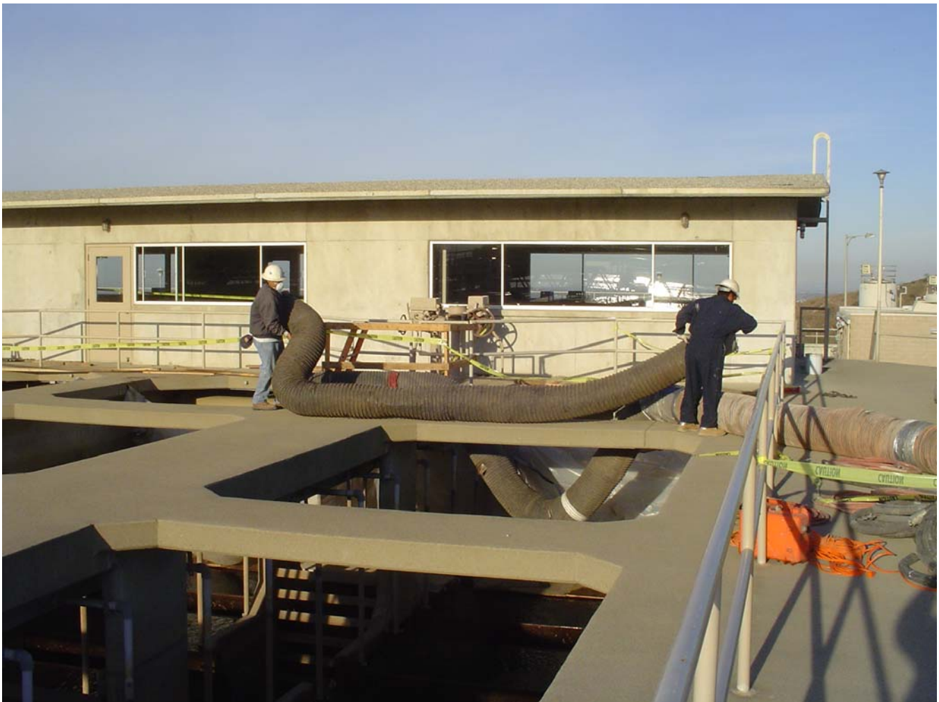
Figure 10: Completed rehabilitation of the filter surface wash headers at Diemer
