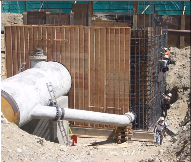
Installation of formwork and reinforcing steel for valve structure
