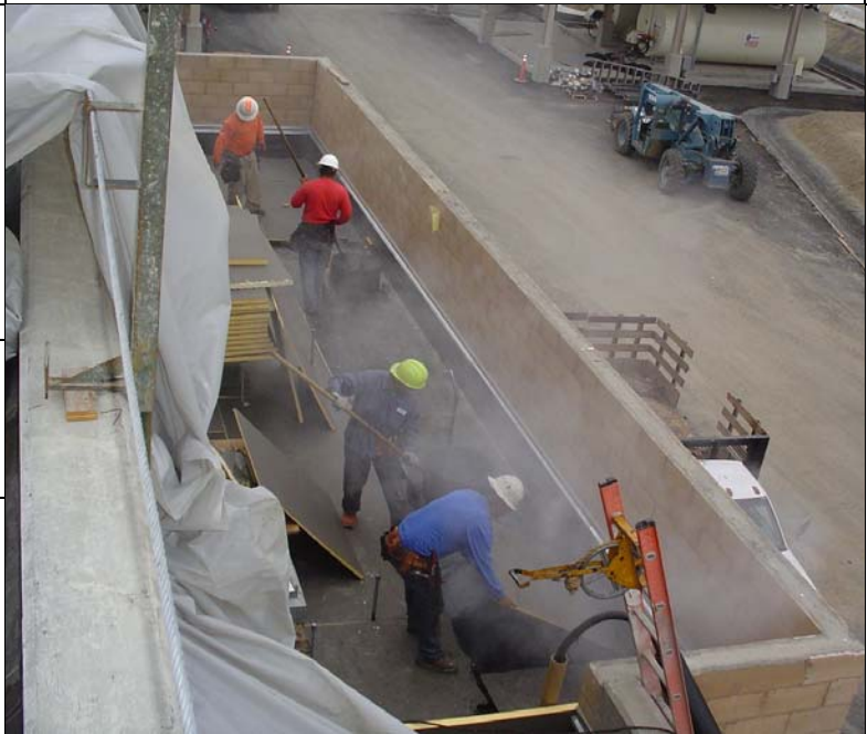
Installation of built-up roofing for Vehicle Maintenance Building
