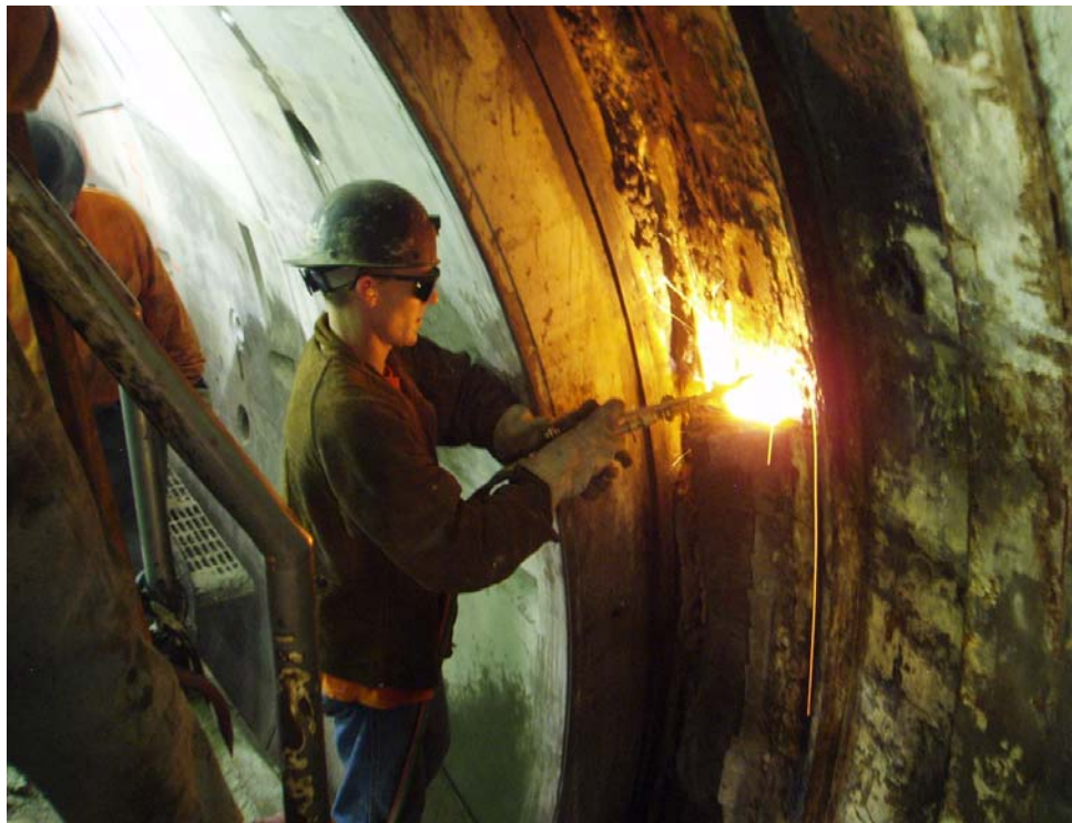
Figure 7: Arrowhead West Tunnel
