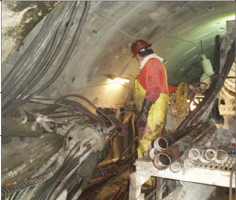
Drilling drain holes behind Arrowhead East Tunnel TBM
