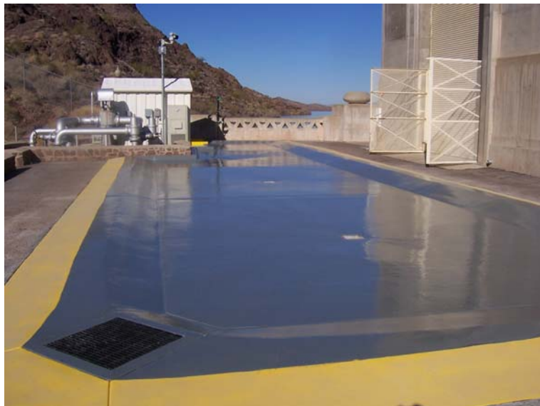
Figure 15: Completed sodium hypochlorite unloading pad
