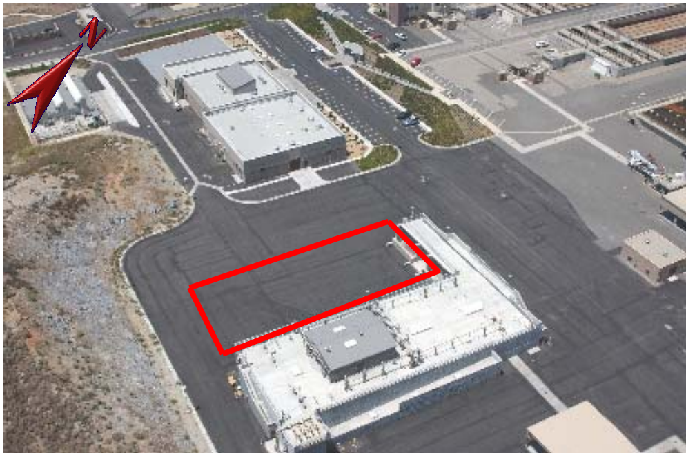
Figure 8: Site of Ozone Contactors Nos. 3 and 4
