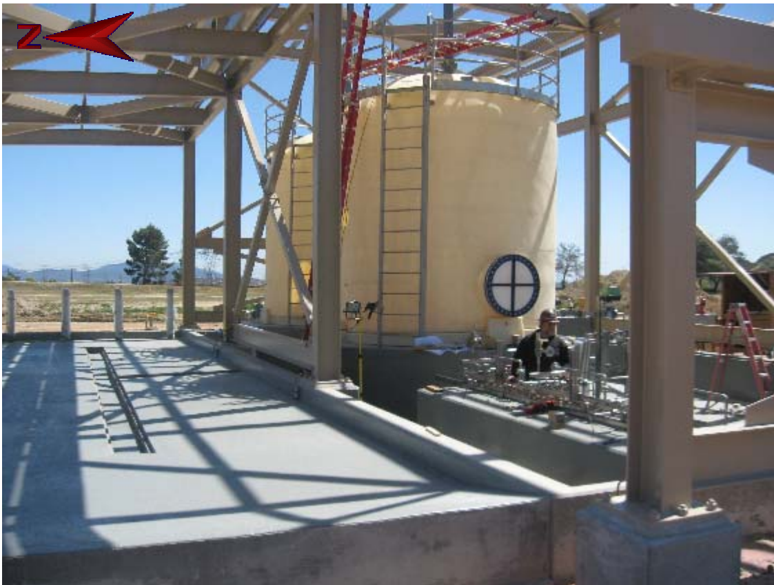
Figure 13: Jensen fluoride tank farm roof structure
