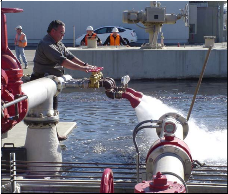
Testing of fire pump
