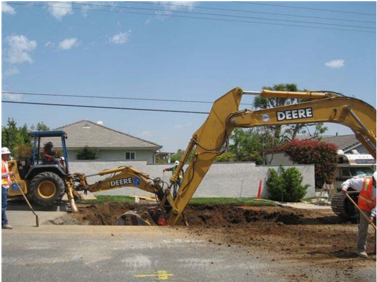
Figure 2: Excavation for Rialto Pipeline repair
