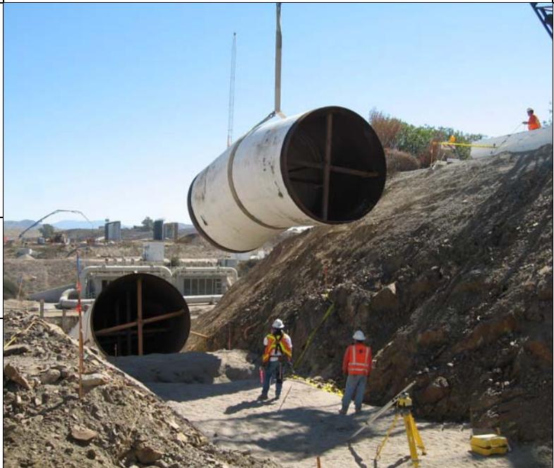
Placement of 144-inch Plant One inlet conduit
