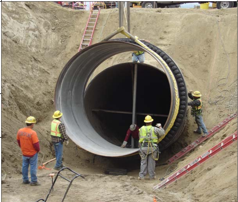
Installation of isolation joint connecting to 144-inch inlet line
