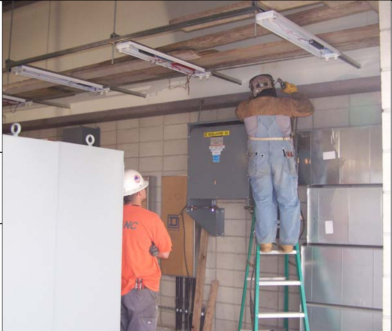
Welding straps to secure electrical transformers
