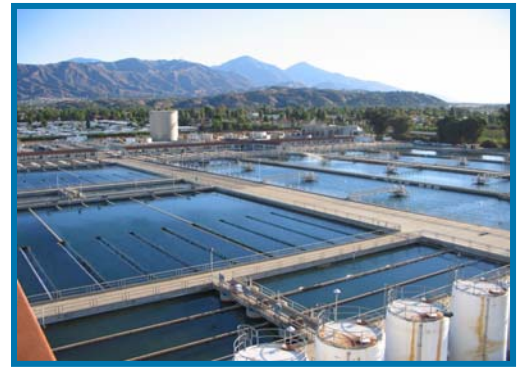
Weymouth Filtration Plant
