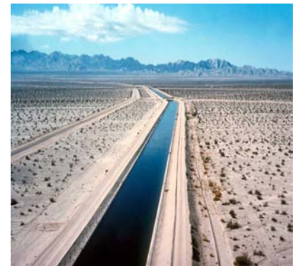
Colorado River Aqueduct
