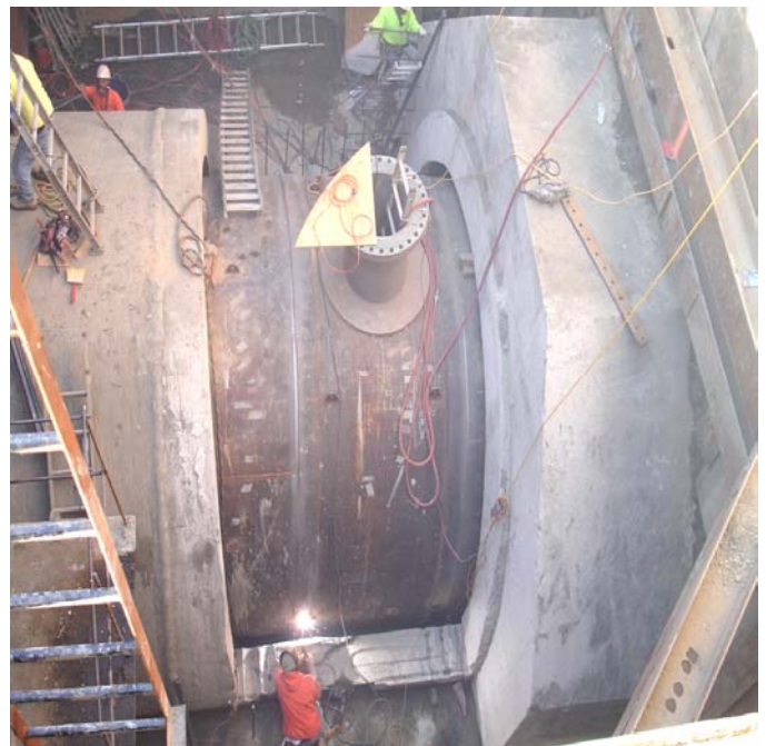
Repair work on the Foothill Feeder located at Valencia Boulevard.
