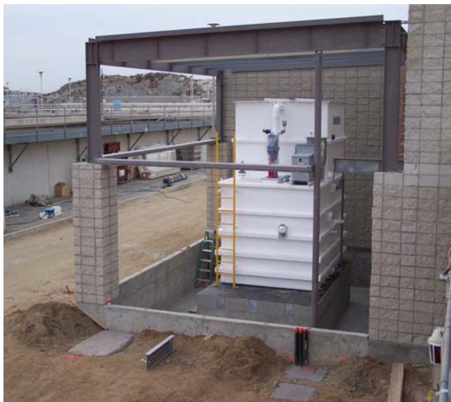
Mills Plant—Installation of chlorine scrubber
