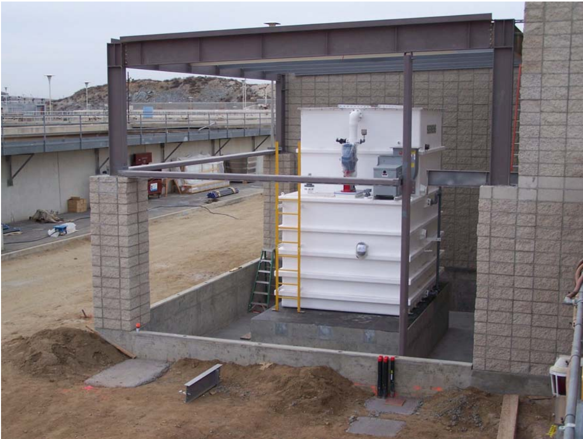
Figure 9: Mills Plant – Installation of chlorine scrubber
