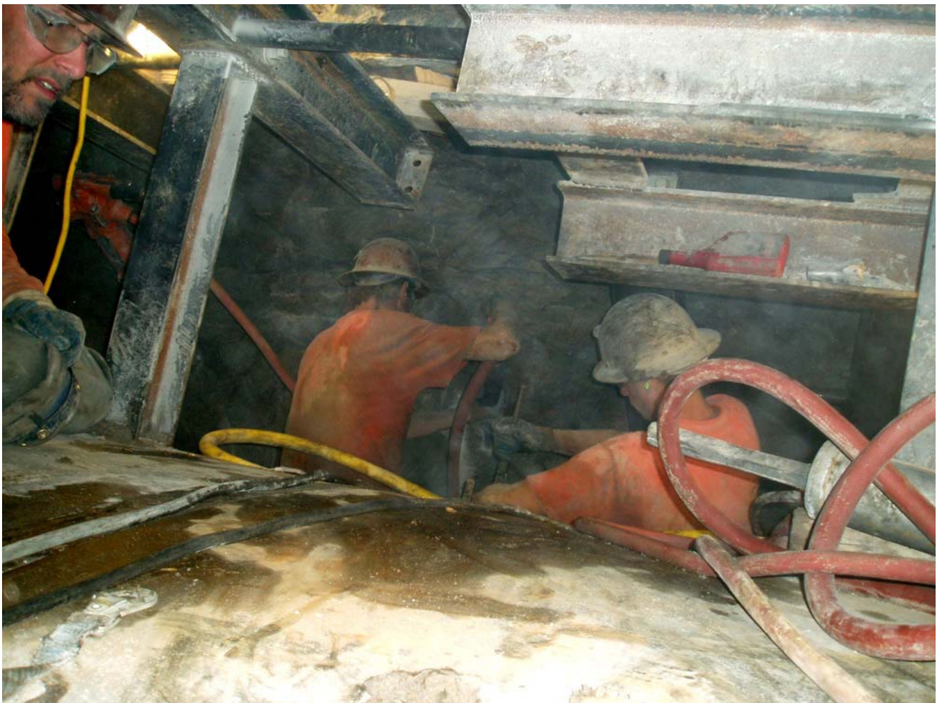
Figure 4: Crew hand excavation above Arrowhead East TBM shield
