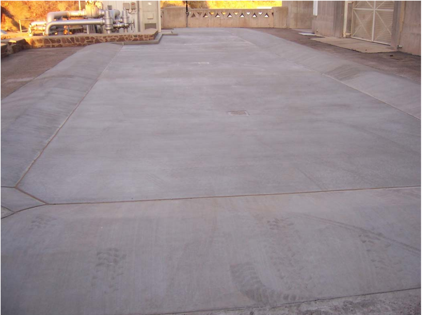
Figure 10: Intake Pumping Plant's new unloading pad for sodium hypochlorite
