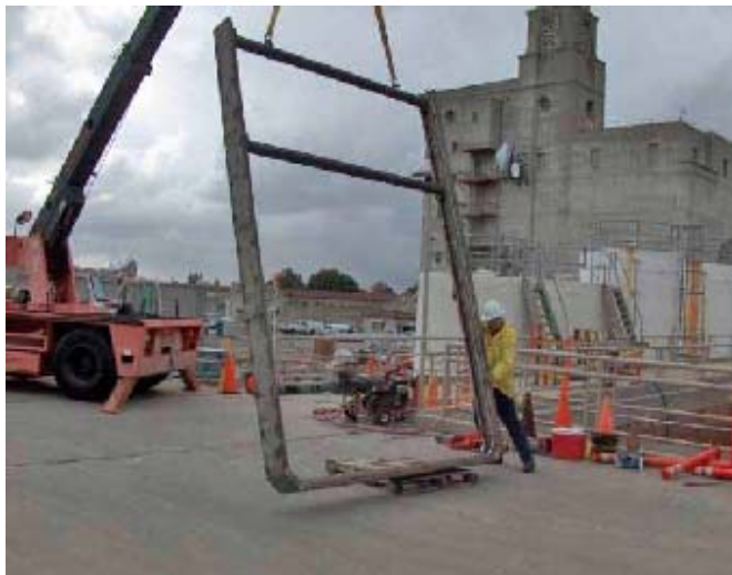
Installation of drop-gate guide at Weymouth
