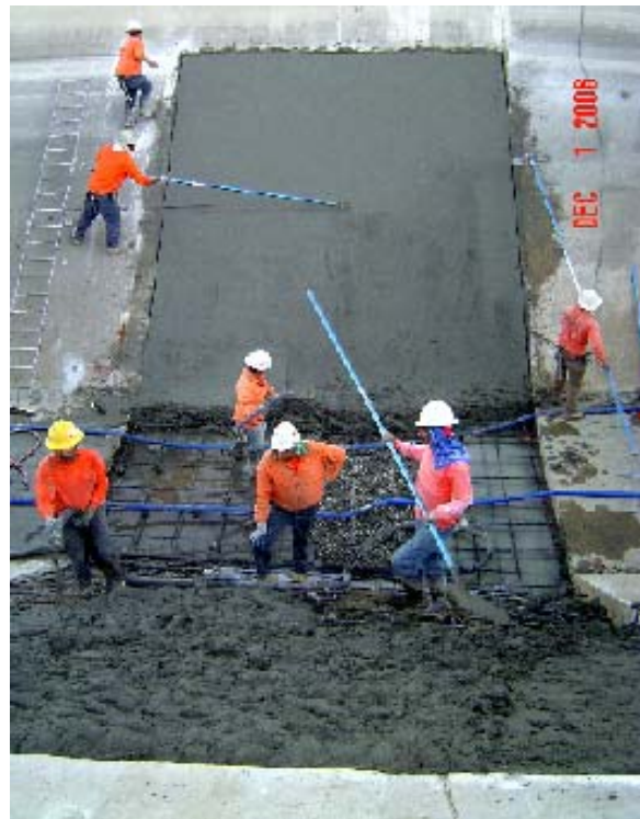
San Diego Canal Finish
