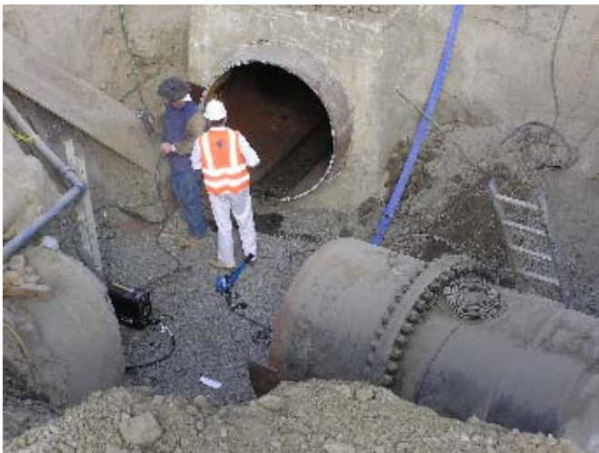
Effluent pipe tie-in of new facilities at Skinner
