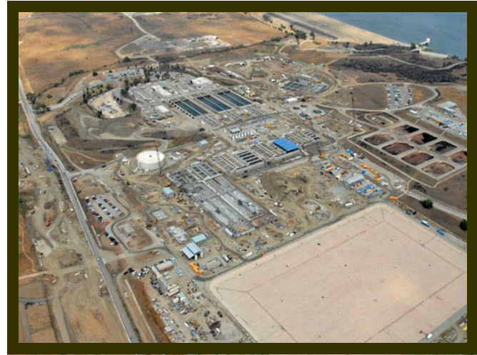
Construction at Skinner treatment plant
