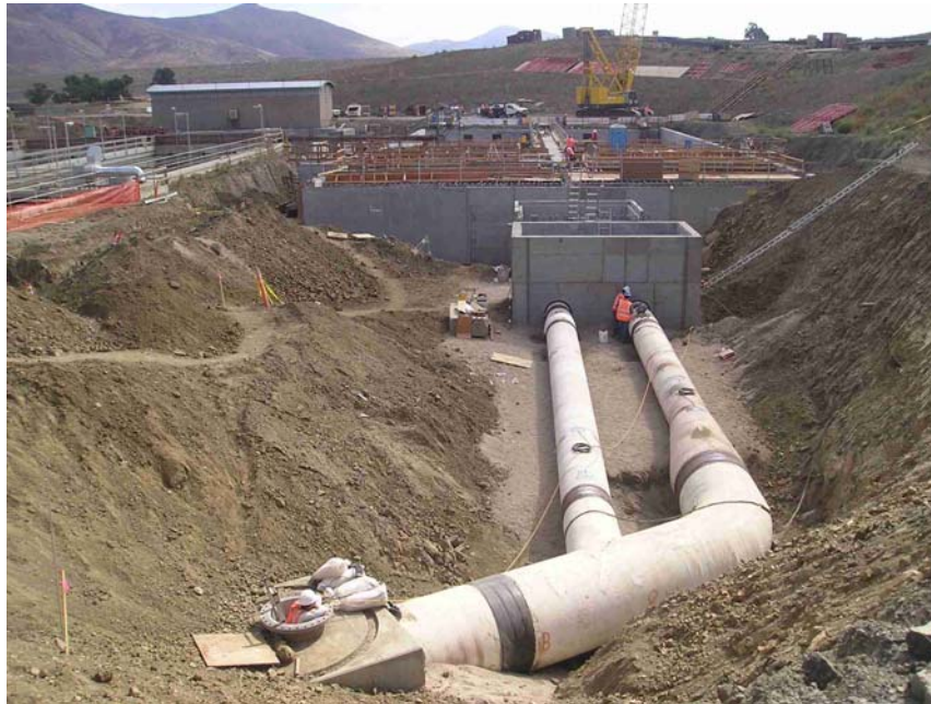
Figure 2: Washwater Reclamation Plant No. 3 Inlet Line – looking southwest
