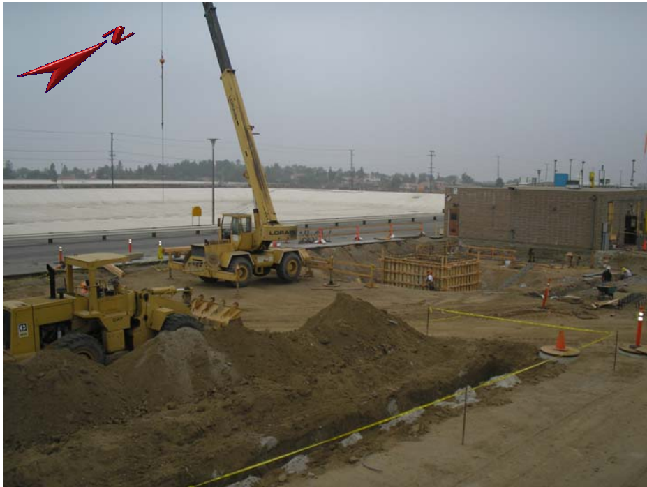
Figure 8: Mills plant – Chlorine containment excavation and formwork
