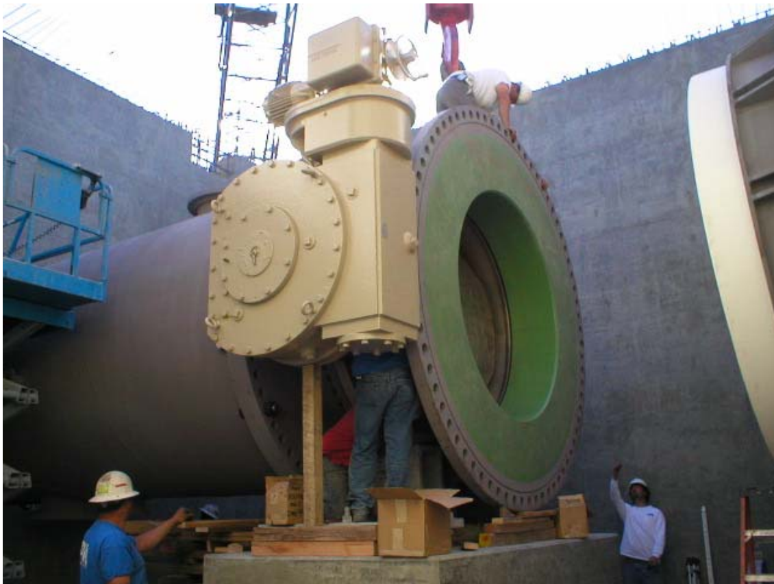
Figure 4: Installation of valve for Perris Valley Pipeline -Phase I
