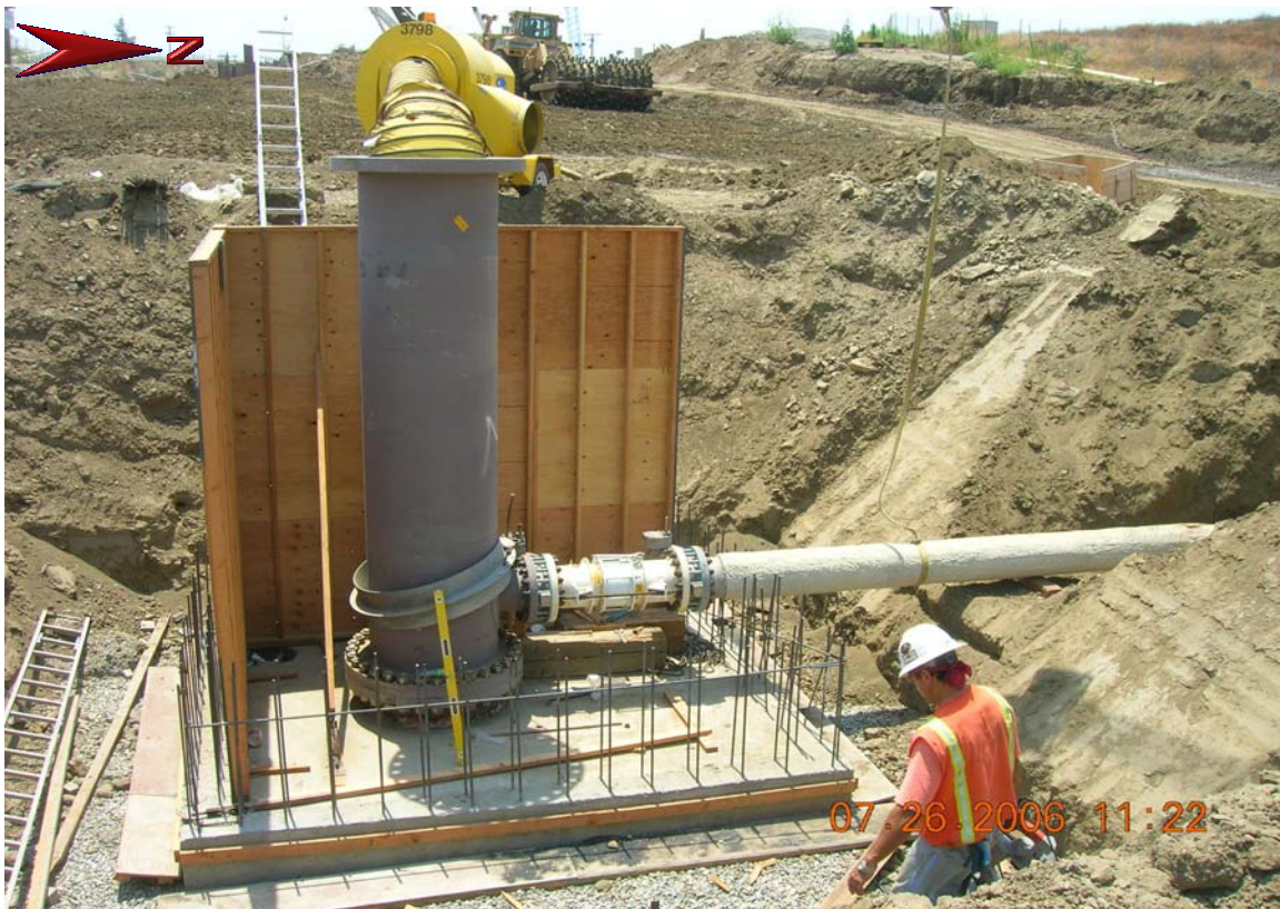
Figure 1: Installation of piping at the blow-off structure
