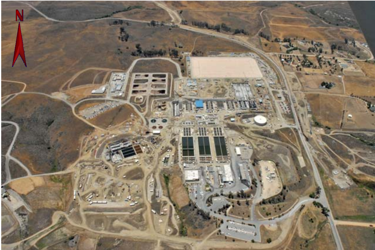
Figure 6: Skinner Finished Water Reservoir in background
