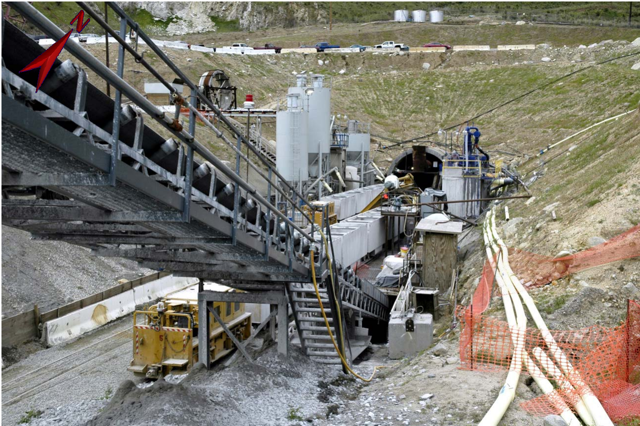
Figure 3: Tunnel operations at the Waterman Canyon portal site
