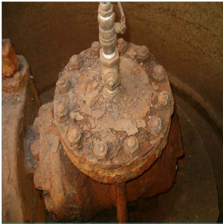
Figure 5: Existing valves to be replaced
