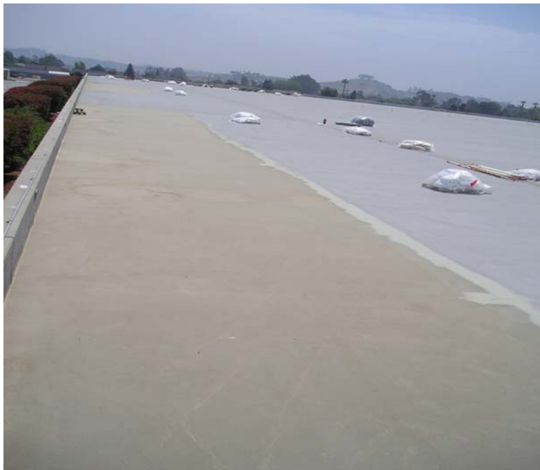
Figure 6: Finished water reservoir roof recoating in process
