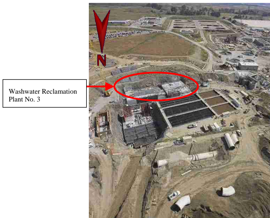
Figure 2: Wastewater Reclamation Plant No. 3
