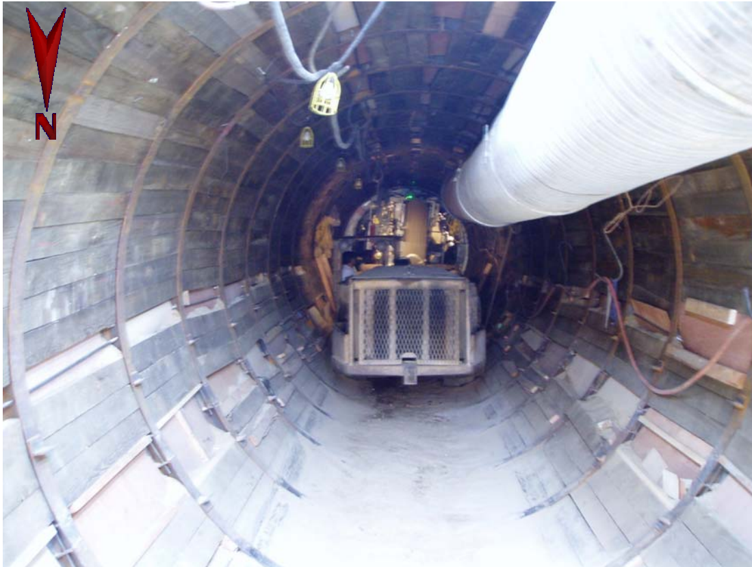
Figure 1: Tunnel Excavation at Rancho California Road
