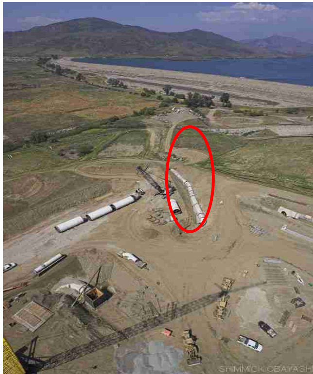
Figure 8: Contactor rejection pipe installation at Skinner
