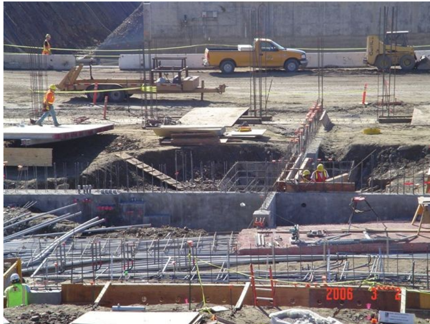
Figure 9: Skinner chlorine containment construction
