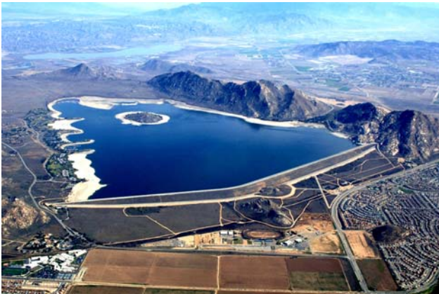
Lake Perris at its interim maximum water surface elevation of 1563 feet, 25 feet below the normal operating level. (MWD Photo.)
