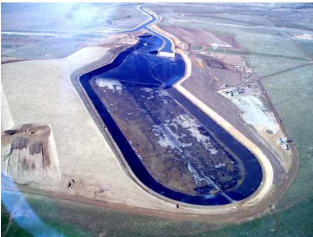
The Tehachapi East Afterbay Phase 1 construction has been completed and the interim connection will begin providing benefits in April. This photo shows the facility during its initial filling in March. (Photo courtesy of DWR.)
