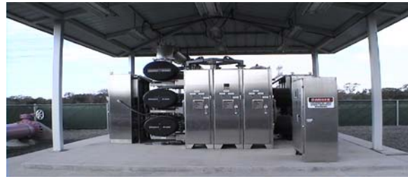
Alamitos Barrier Reclaimed Water Project (Ultra-violet Disinfection) (sponsored by Central Basin MWD)
