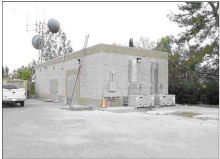
Metropolitan’s Disaster Recovery Facility
