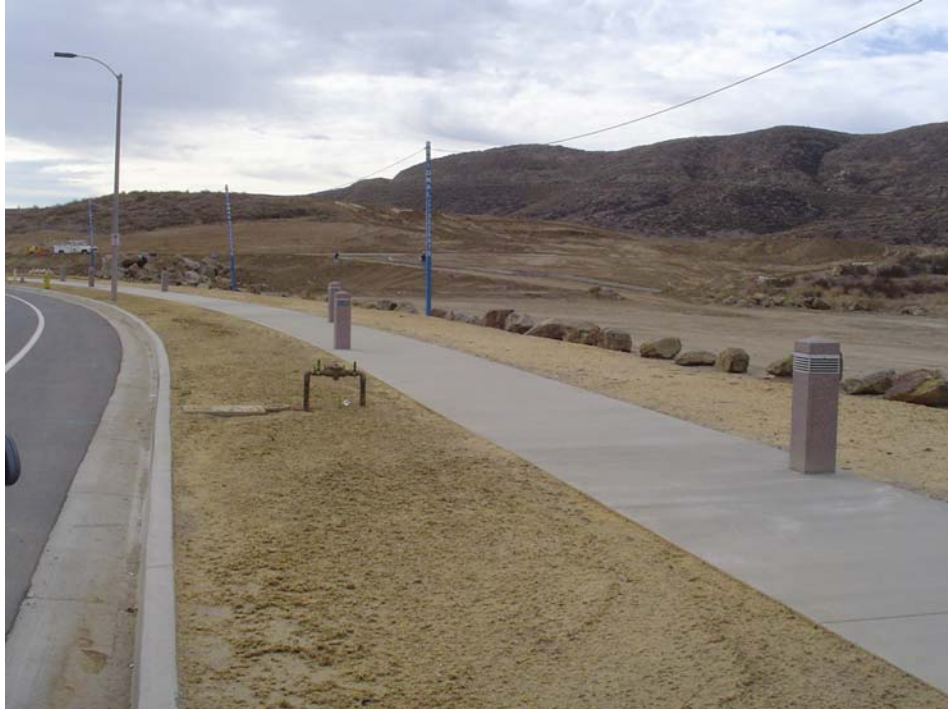
Figure 1: Searl Parkway Phase I area, ready for landscaping.
